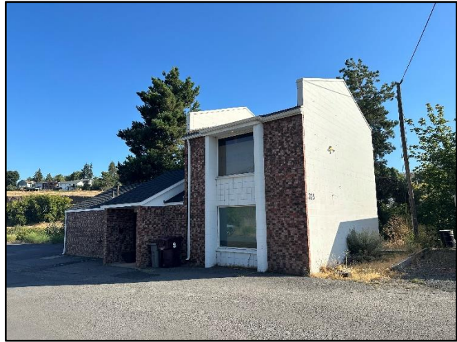
Pullman Marketing Building 325 NW State Street, Pullman, Washington
