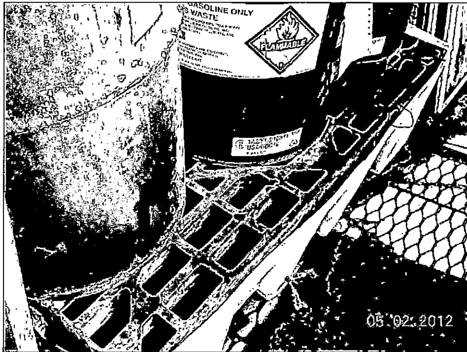
Photograph 21: Secondary containment for drums in storage yard.
