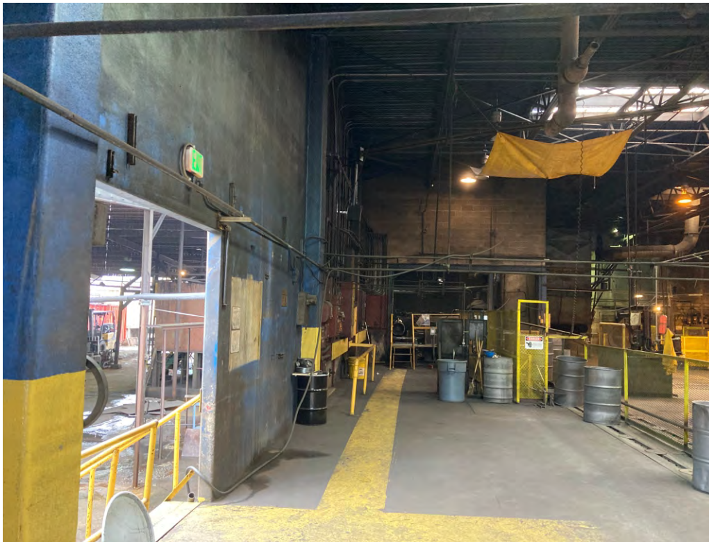
Fig. 7a - 10' Door in North Wall (view to east -10-2021 #1339)
