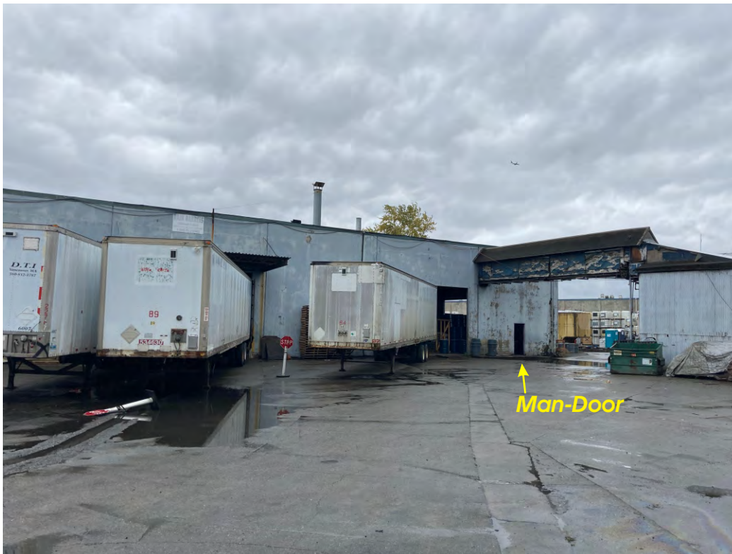
Fig. 3b - 20' Doors and Man-Door - SW Bldg. Corner (view to south-east (10-2021 #1323)
