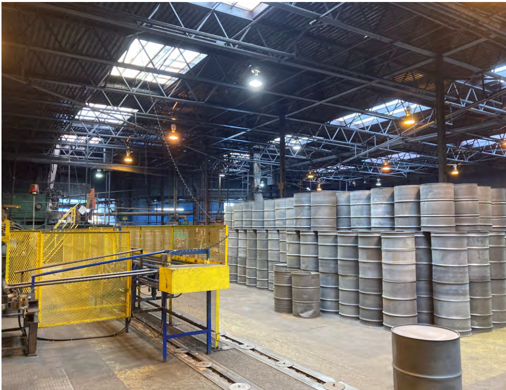
Fig. 7b - General View of Building Interior (10-2021 #1345)
