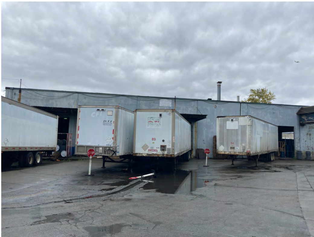
Fig. 3a - Three 20' Loading Doors (view to east - 10-2021 #1322)
