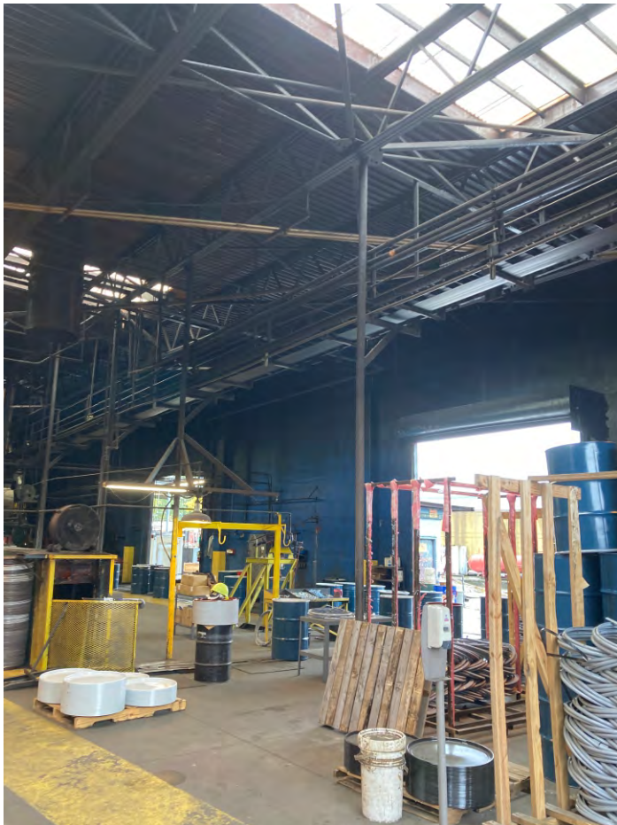
Fig. 6b - 15' Doors in South Wall view to southeast (10-2021 #1328)
