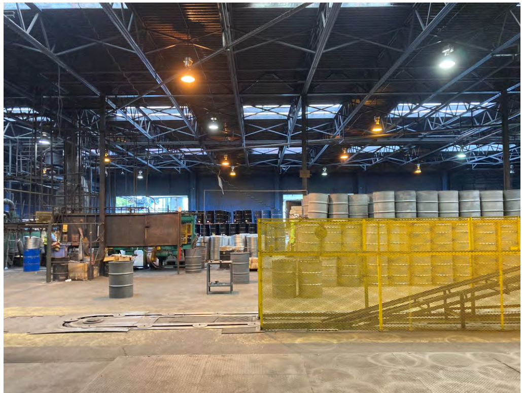
Fig. 4b - 20' Doors West Wall + Interior (view to west (10-2021 #1350)
