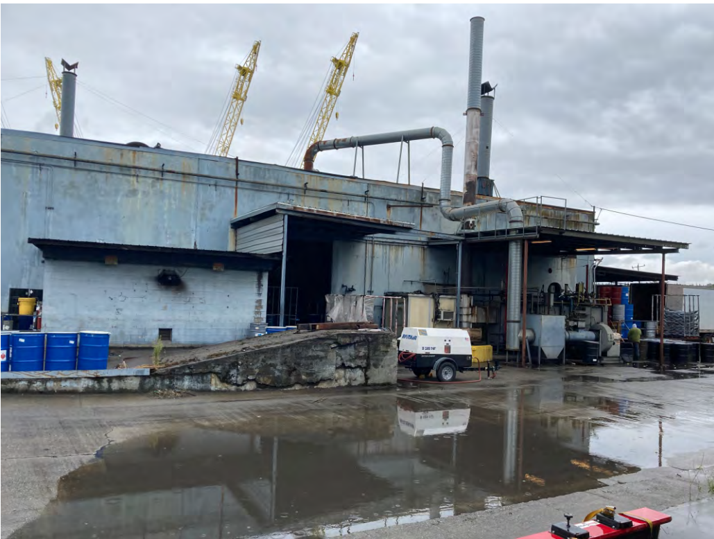
Fig. 5b - East 15' Door in South Wall (view to northeast (10-2021 #1327))
