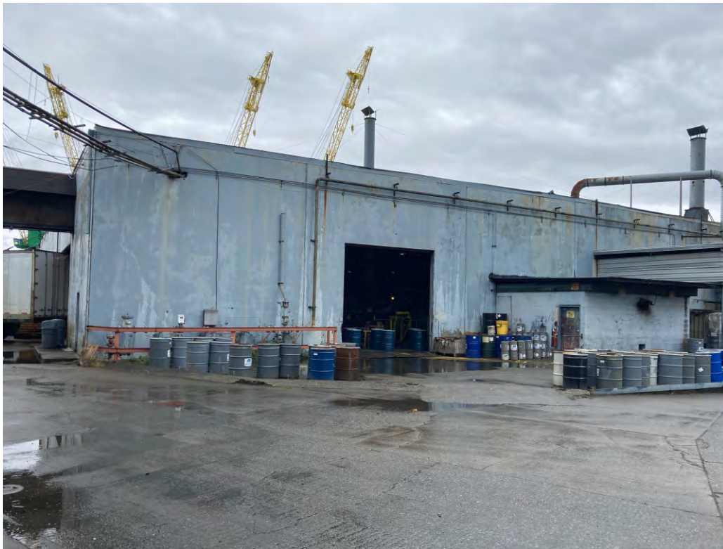
Fig. 5a - West 15' Door in South Wall (view to northeast (10-2021 #1325))
