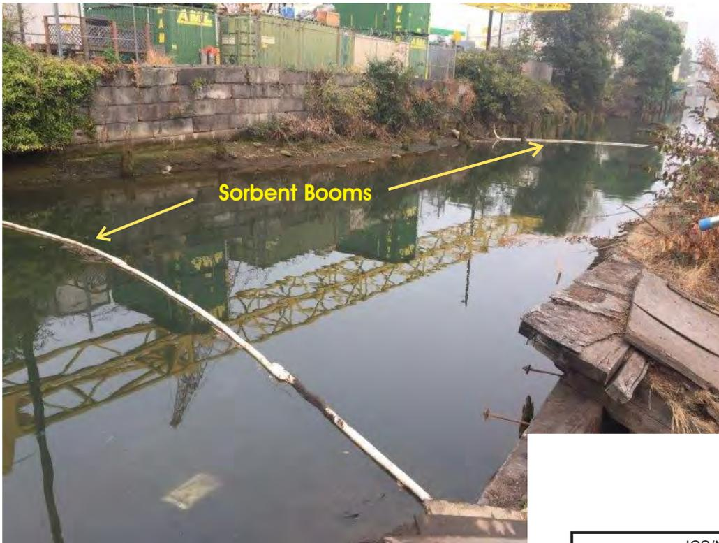
Fig. D-2b - Water Surface During Flood w/ Booms In-Place (After sampling 9-16-20 - view to east - mouth)
