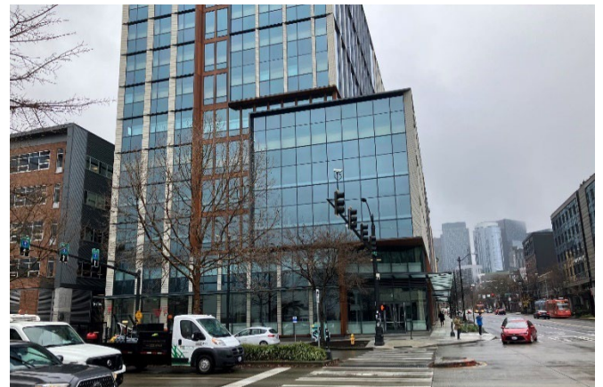
New construction at Block 38 West Property, February 2023
