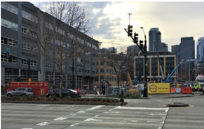
Construction progress at Block 38 West Property, December 2019
