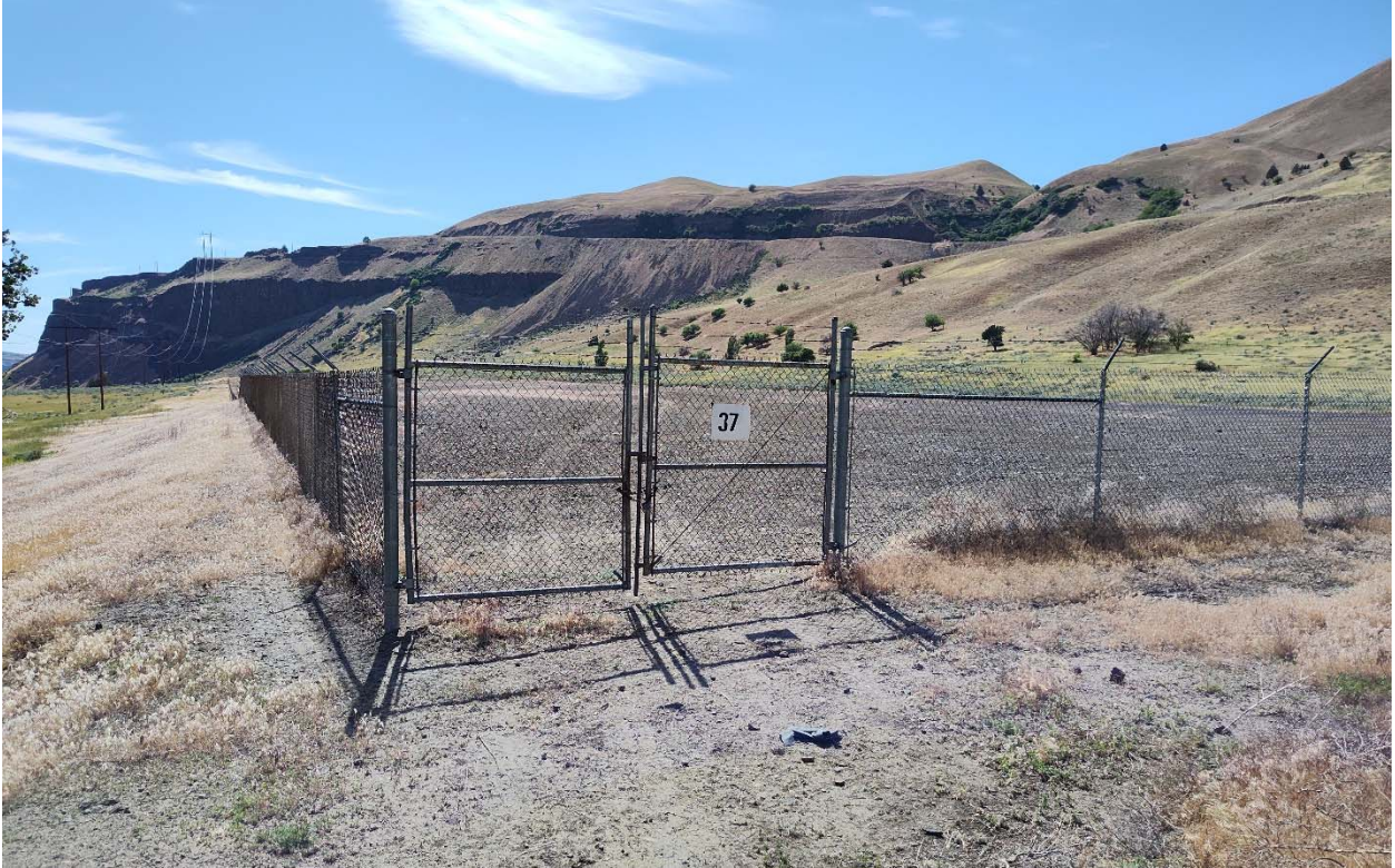
Cleared out sagebrush at the gated entrance in the southeast corner of the WSI.
