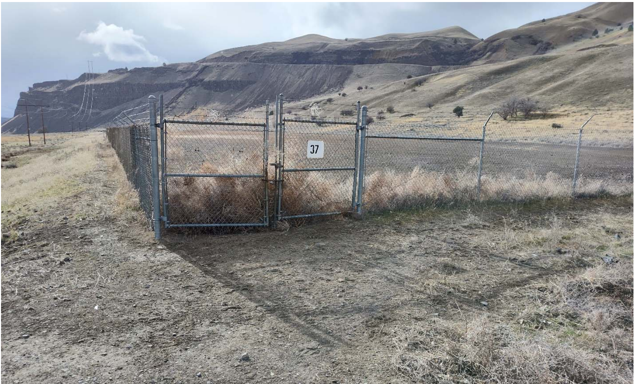
Sagebrush at the entrance to the gate near the southeast corner of the WSI.
