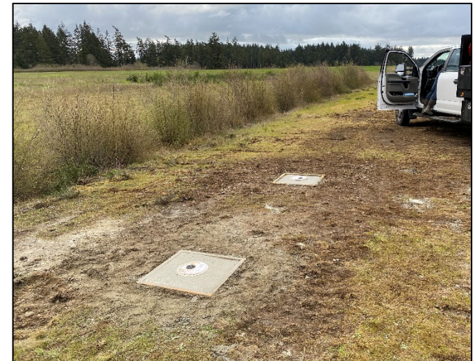
Complete groundwater well installation (two wells at 'same location' and 'different depths')
