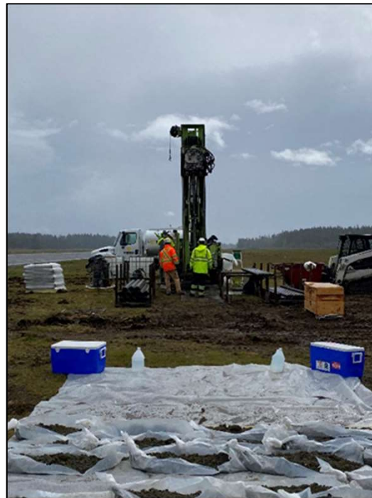
Drilling new monitoring well and soil samples
