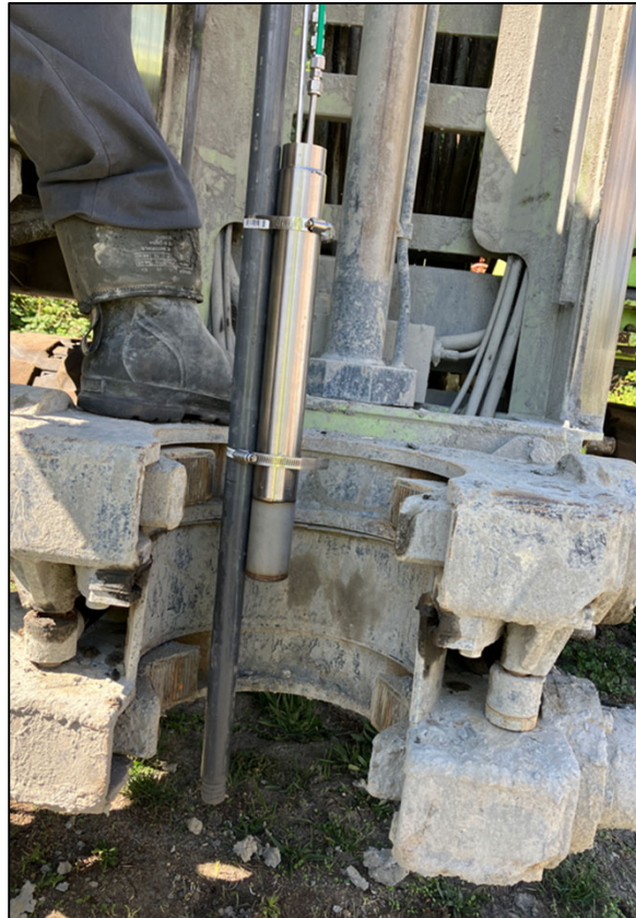
Lysimeter installation at Current Fire Training Area
