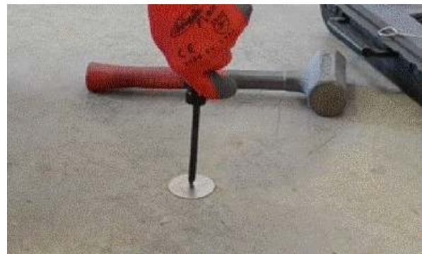
Figure 5. Tightening the Secured Cover.
