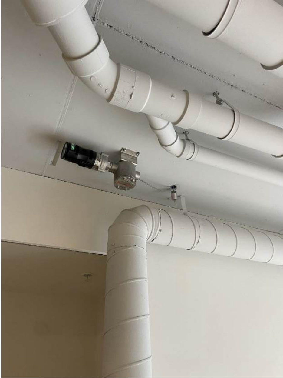
Photo 2. Installed and calibrated temporary PrimaX® IR detector in Building A Live/Work Unit.
