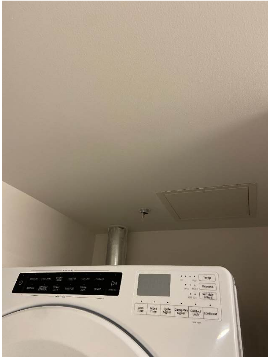
Photo 5. Main level gas sample point.
