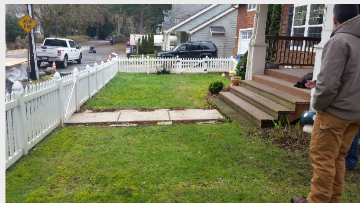
2 From the northwest corner, facing east.
