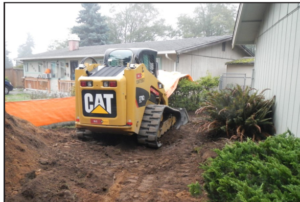
We remove the top 6 to 18 inches of contaminated soil.
