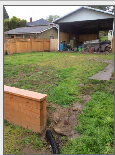
1 Former blacktop driveway exclusion area
