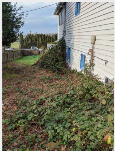
1 South side looking west.
