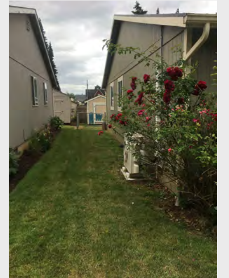
4 From northeast, facing south.
