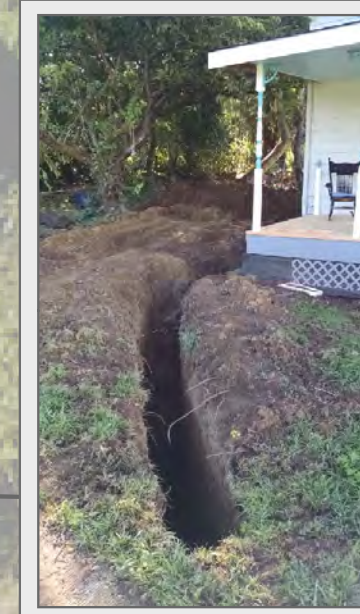
5 Front yard - exclusion area
