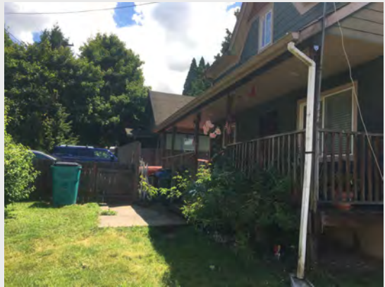
1 From northwest corner looking east.
