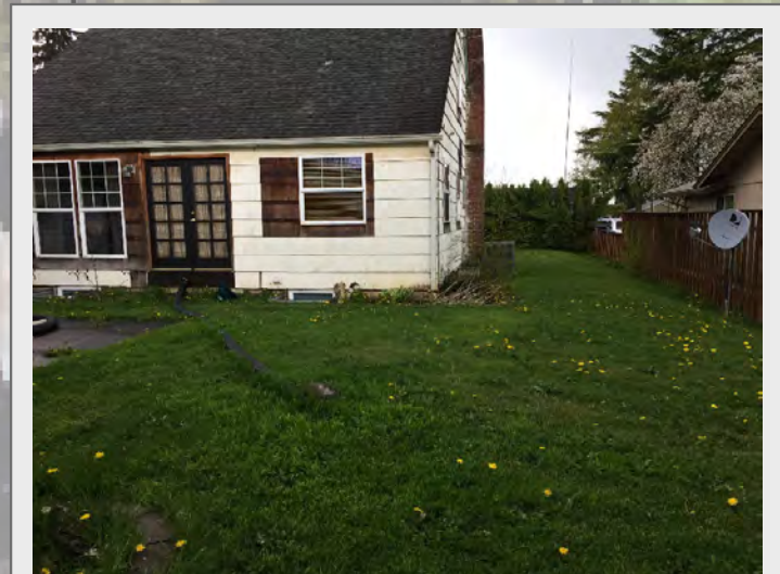
3 Back yard / north side yard, facing west.
