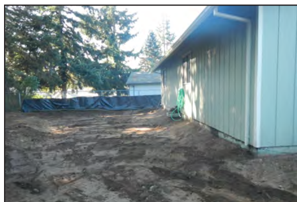
We bring in new soil to backfill the area.
