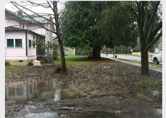
3 From the north, facing west.
