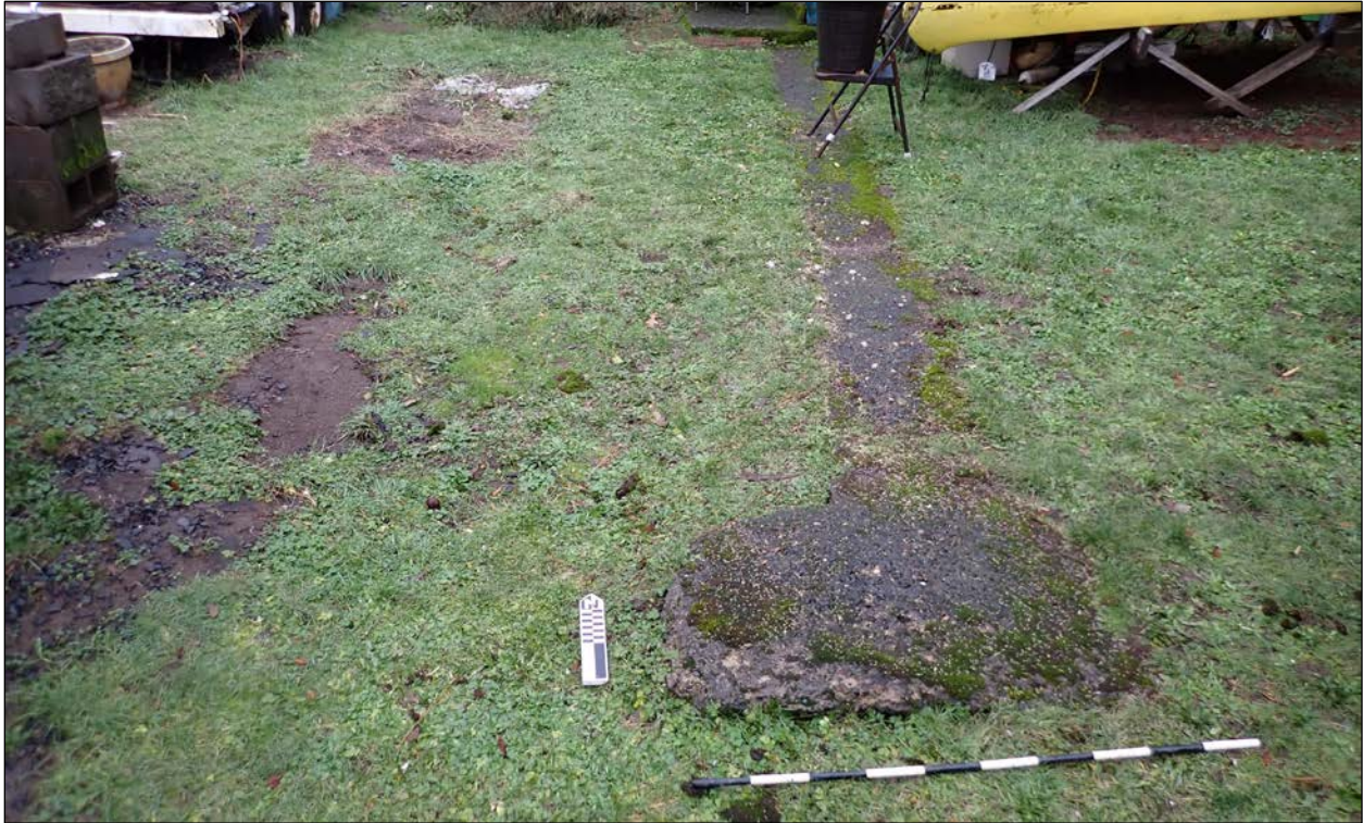
Figure 12. A northward view of the concrete protruding from the ground within the back yard of parcel 080.
