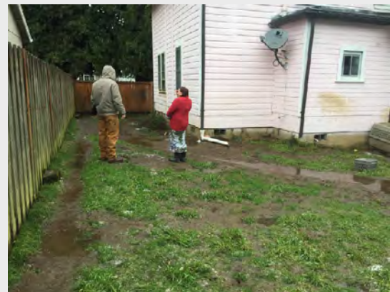
2 From the southeast corner, facing west.
