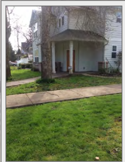
1 Front yard - facing southwest
