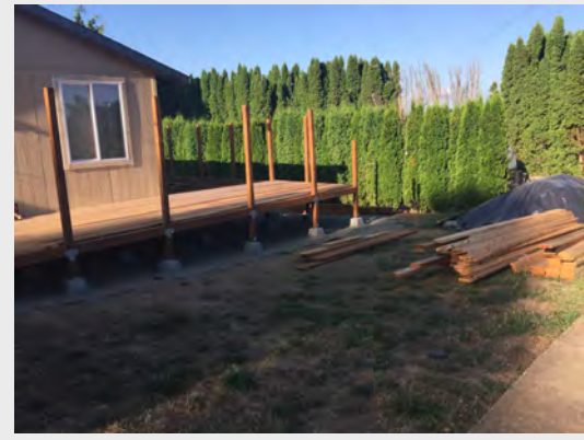
1 From northeast corner facing southwest.
