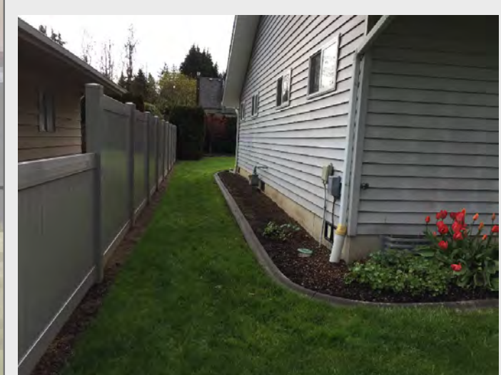
1 North side yard, facing east.
