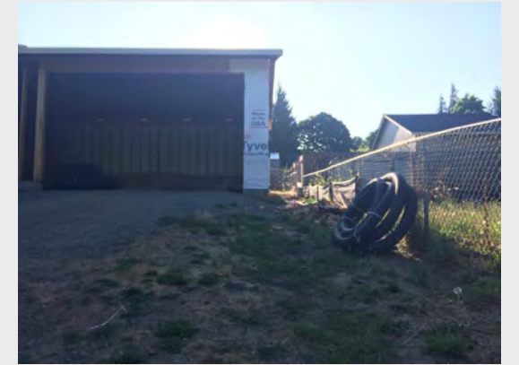
4 From southwest corner facing east.
