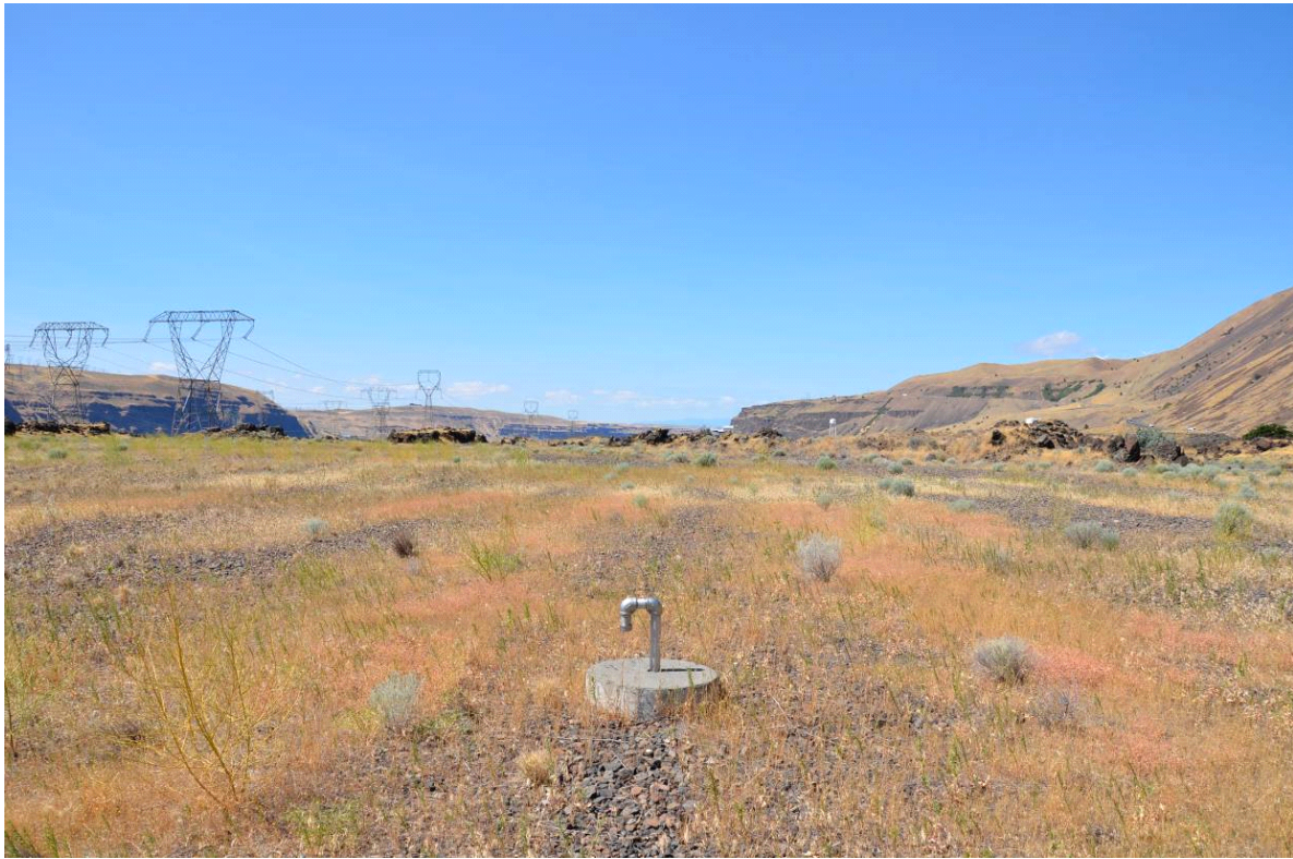
Photograph No. 1: View of capped Vent #1 (typical of Vents #1 and Vents #3 through #9).
