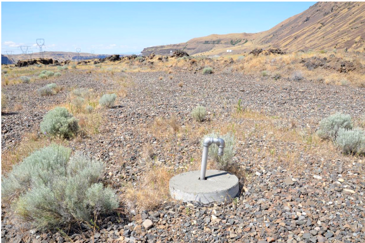
Photograph No. 2: View of capped Vent #2 with bent riser.
