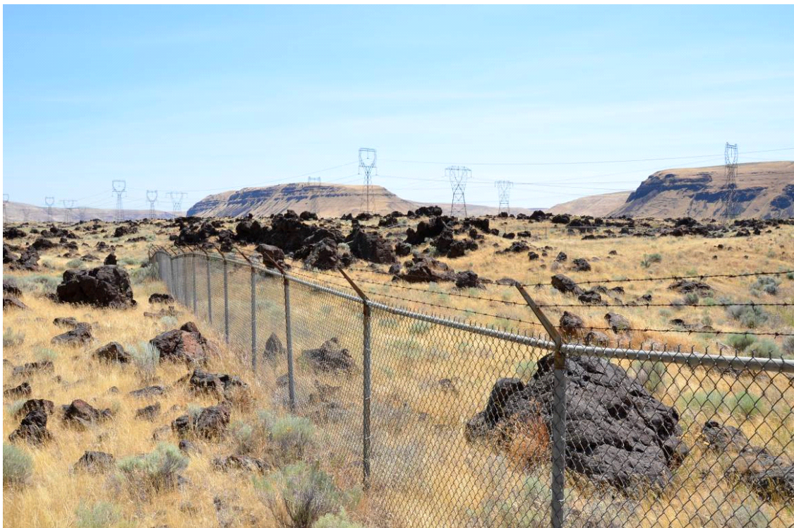
Photograph No. 12: View to the east along northern boundary fence of ESI (typical of entire exterior fence perimeter).
