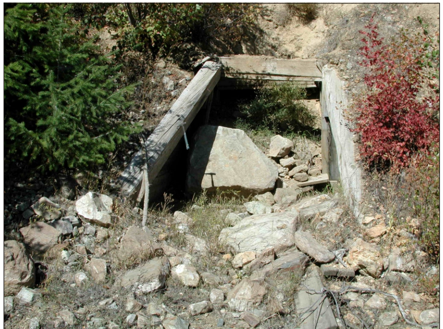
Figure 9. Deer Trail #2 adit showing typical condition of pre-1920 openings.
