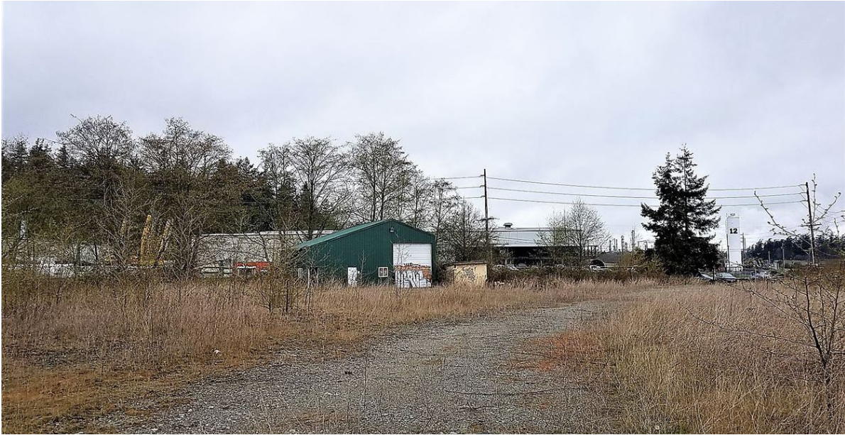
Photo 5 Whitmarsh Landfill prior to vegetation and tree removal. View toward T. Bailey facility (white building in background) and the western half of the project. Note the tall trees in front of the T. Bailey facility but behind the landfill, along South March Point Road.
