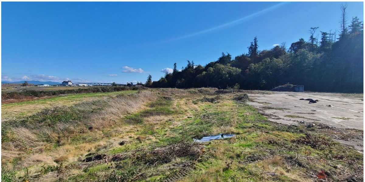
Photo 4 Whitmarsh Landfill post-vegetation and tree removal. Photo taken near Photo 3 location, view toward the northeastern half of the project site and the March Point Heronry. Much of the tall vegetation along South March Point Road, between the landfill and the heronry, remains.
