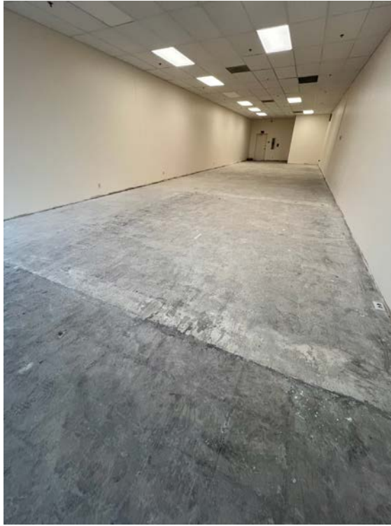
Photograph 15. Floor Slab and Ceiling in Suite B7 (November 14, 2024)
