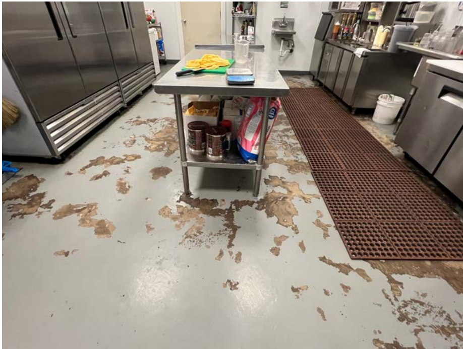
Photograph 10. Floor Slab in Kitchen of Adjacent-West Tenant Space (Suite B5) (November 14, 2024)
