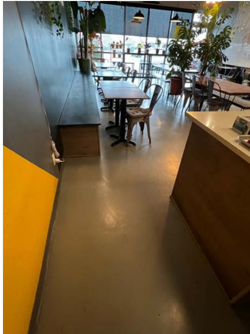
Photograph 8. Floor Slab in Adjacent-West Tenant Space (Suite B5) (November 14, 2024)
