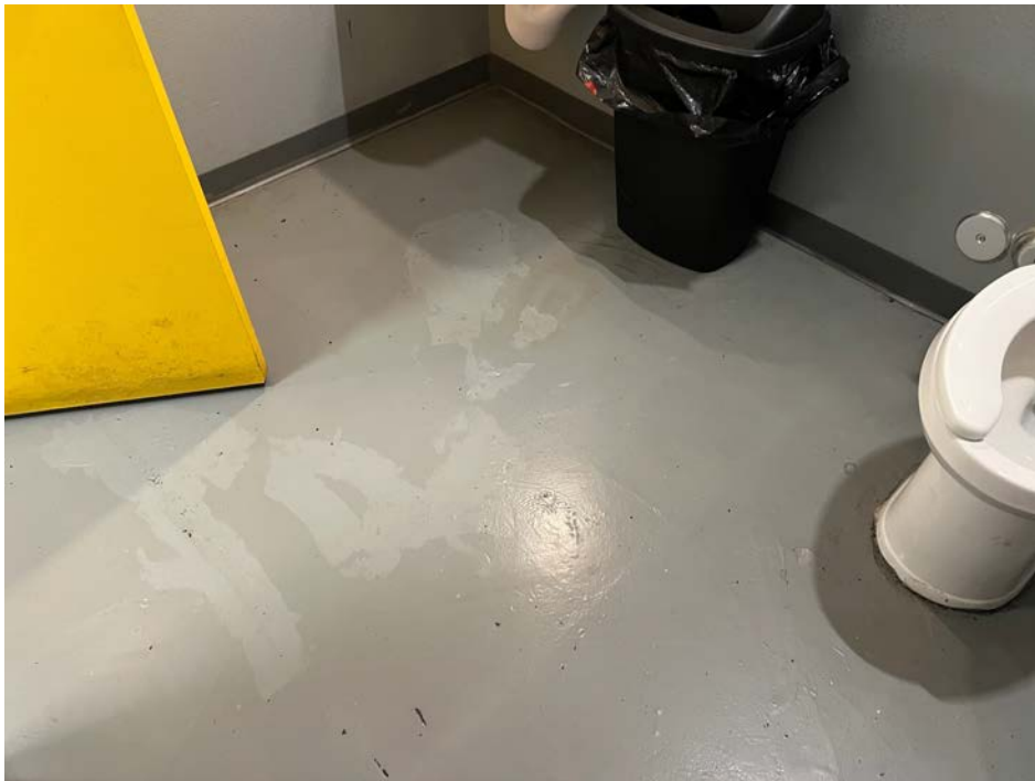
Photograph 14. Floor Slab in Bathroom 2 of Adjacent-West Tenant Space (Suite B5) (November 14, 2024)
