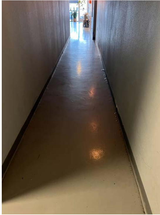
Photograph 9. Floor Slab in Hallway of Adjacent-West Tenant Space (Suite B5) (November 14, 2024)
