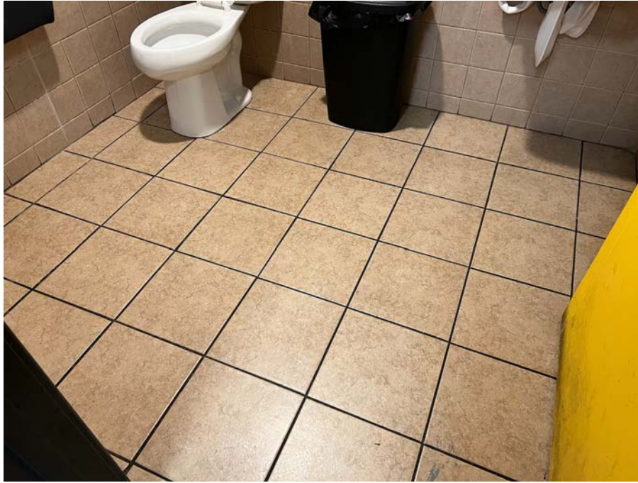
Photograph 13. Floor Slab in Bathroom 1 of Adjacent-West Tenant Space (Suite B5) (November 14, 2024)
