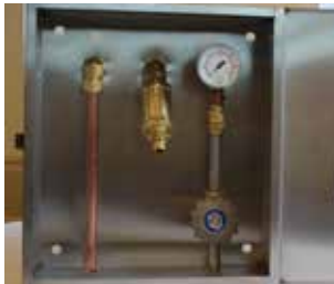
Exterior stainless steel wall box for remote filling of the Perma-Cyl storage vessel.
