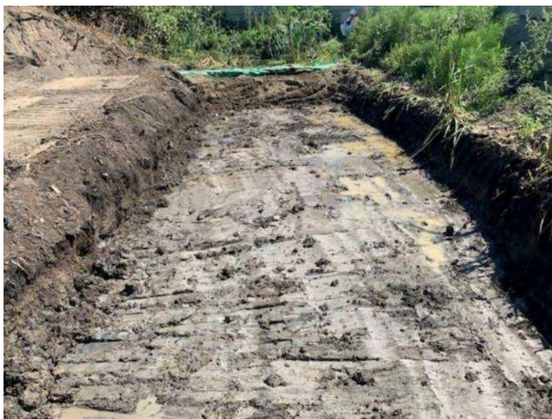
Figure 49: Bottom and western sidewall of RAU D11
