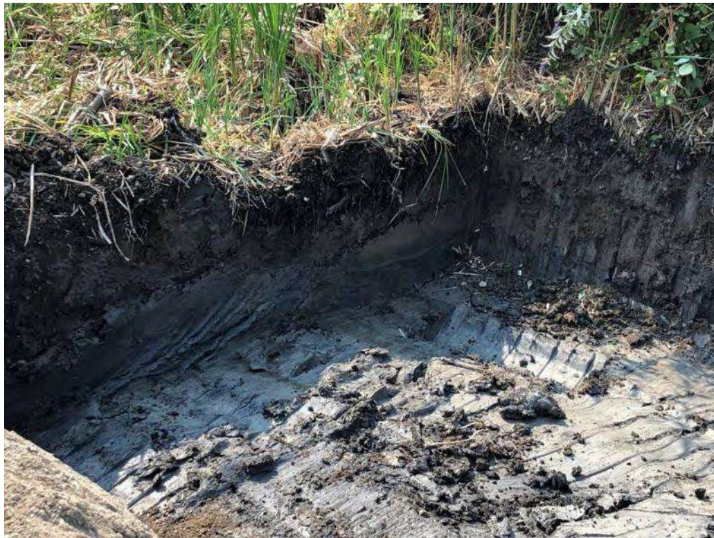
Figure 40: Bottom of RAU D2 NOTE: Three foot thickness of clay-rich silt bottom
