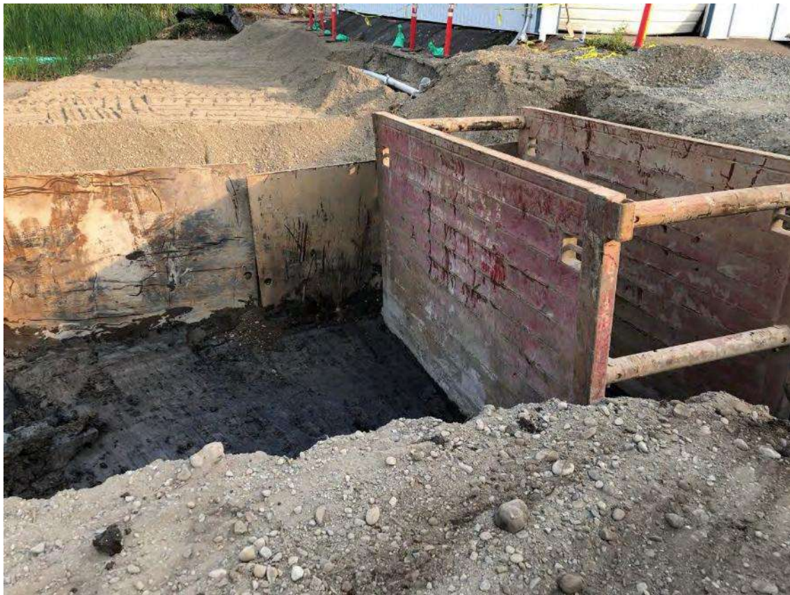
Figure 29: Bottom of RAU B8 – Note use of Trench box and steel sheets to prevent caving
