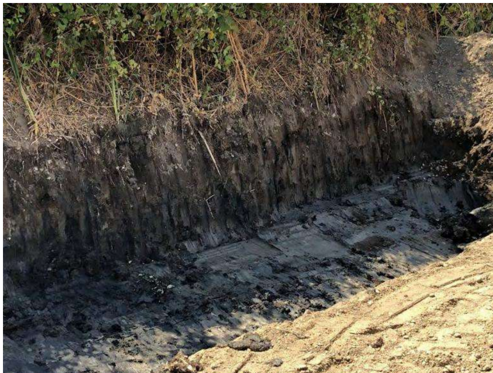
Figure 44: Bottom and western sidewall of RAU D6
