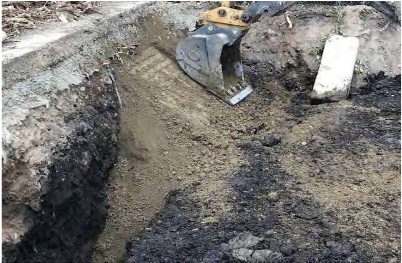
Figure 10: Construction of Clay barrier. Finished product. Note ragged edge of introduced fabric two feet bgs. The fabric was placed below the grade backfill was installed during remediation of the adjacent soils
