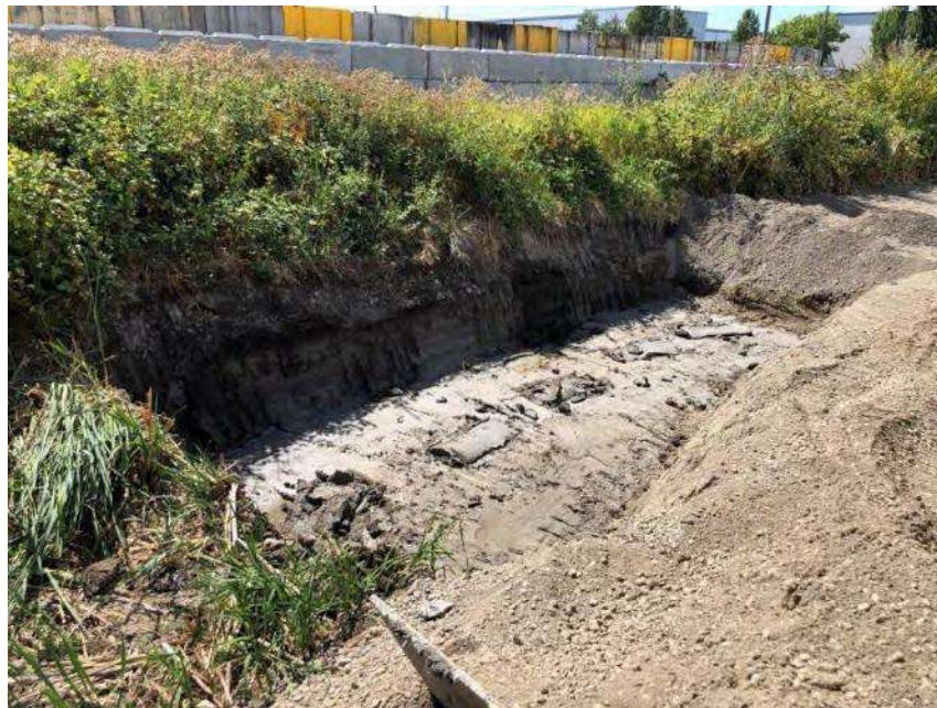
Figure 42: Bottom and western sidewall of RAU D4
