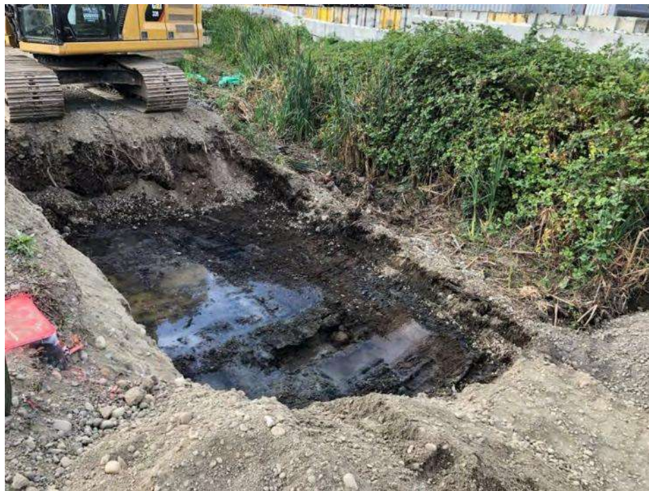
Figure 33: Bottom of RAU B12 - NOTE Narrow width the RAU and oil sheen on water
