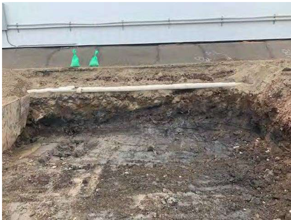
Figure 24: RAU B5: Eastern sidewall at 0-5 feet: Note shot intermixed with soil on the right end of the excavation.
