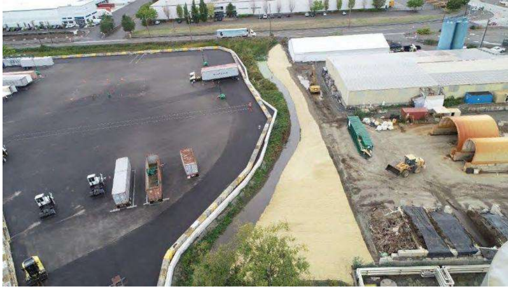
Figure 14: Aerial view of straw mat prior to hydroseeding
