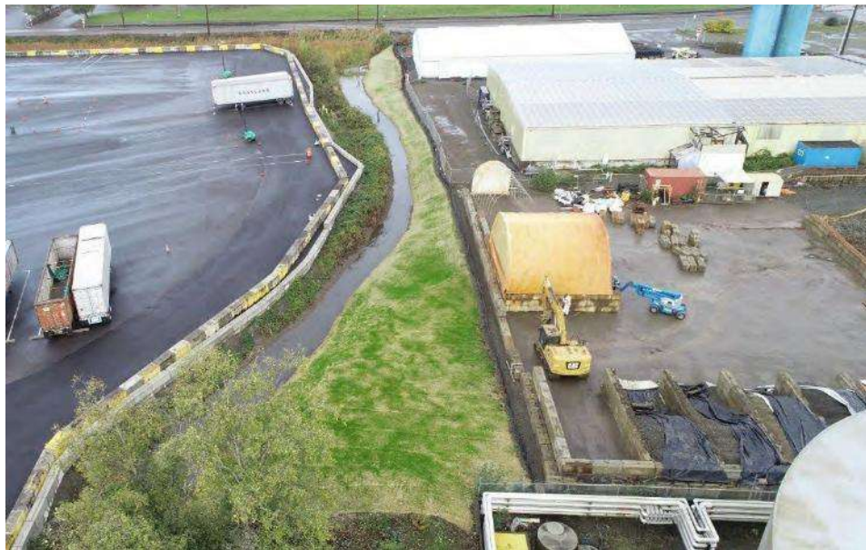
Figure 15: Aerial View 10 days after hydroseeding
