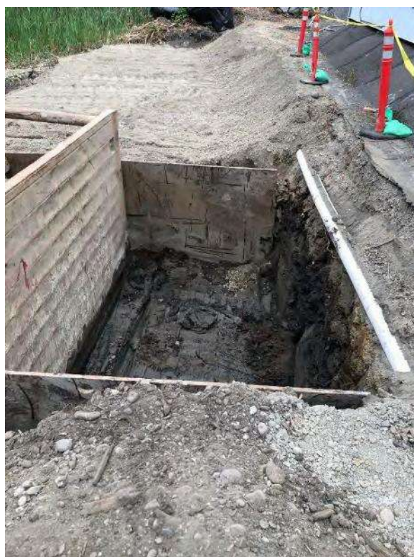
Figure 27: Use of steel plates and trench box to prevent caving
