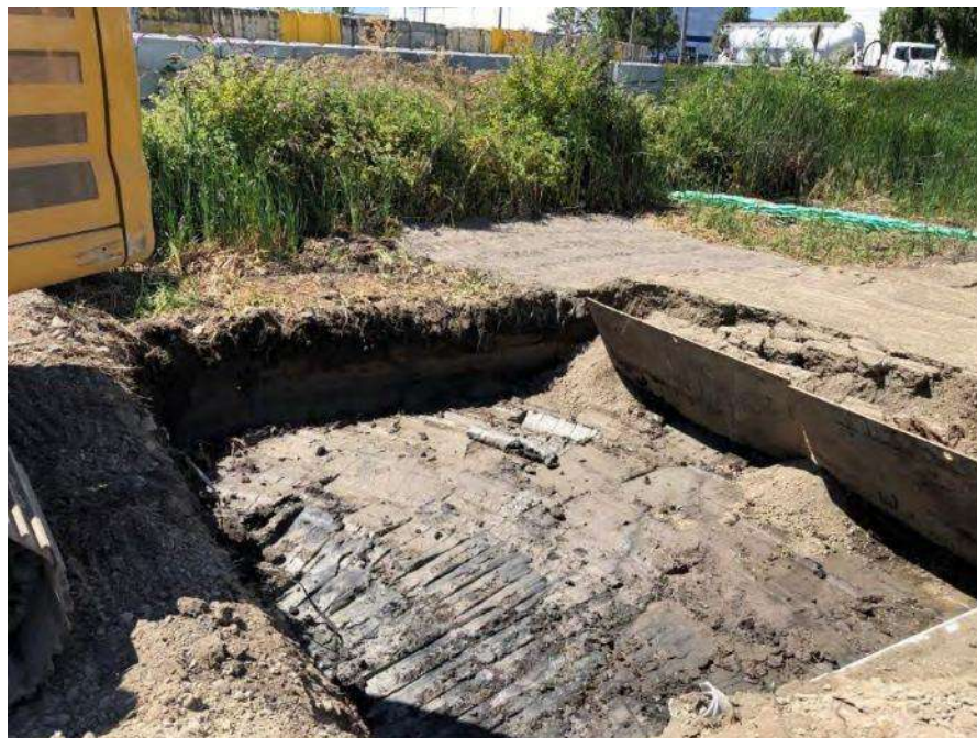
Figure 26: Bottom of RAU B6 – NOTE Steel plates used to prevent sidewall caving
