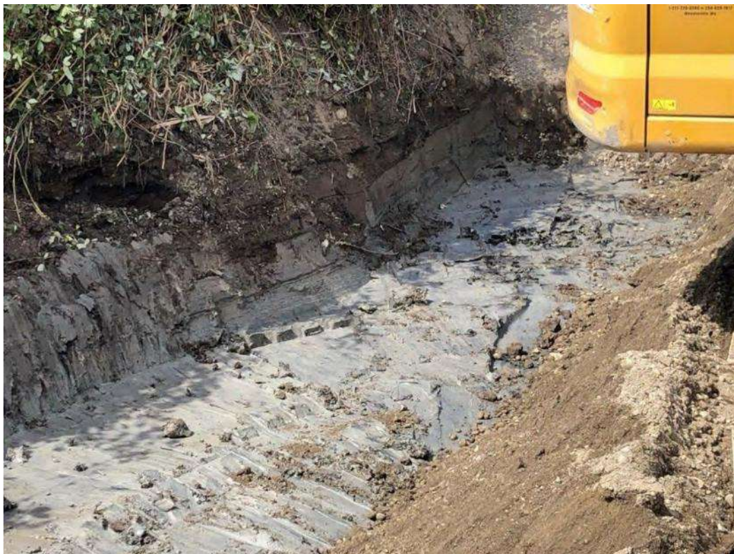
Figure 46: Bottom and western sidewall of RAU D8
