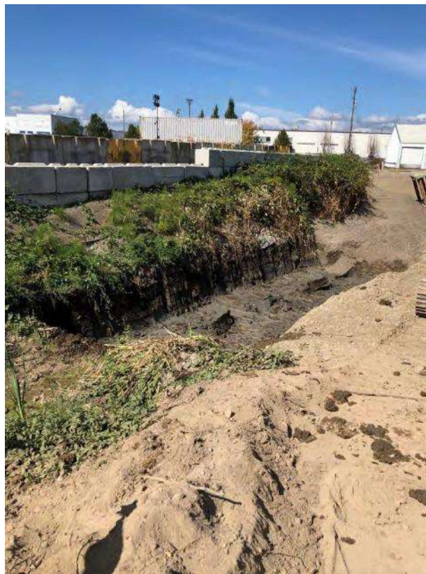
Figure 47: Bottom and western sidewall of RAU D9
