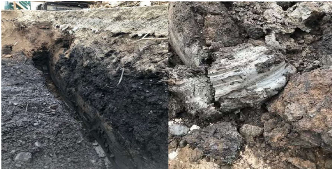
Figure 11: Trench prior to filling with Clay
