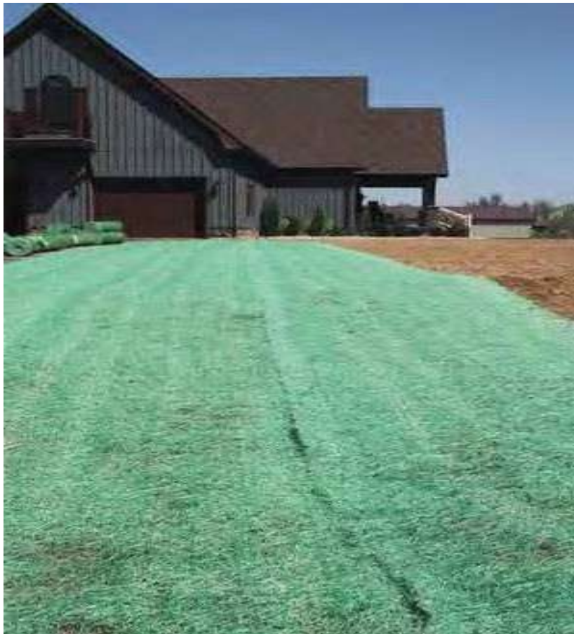
Figure 13: Stock Photograph – Bio-gradable Erosion Control Netting (Product Installed)
