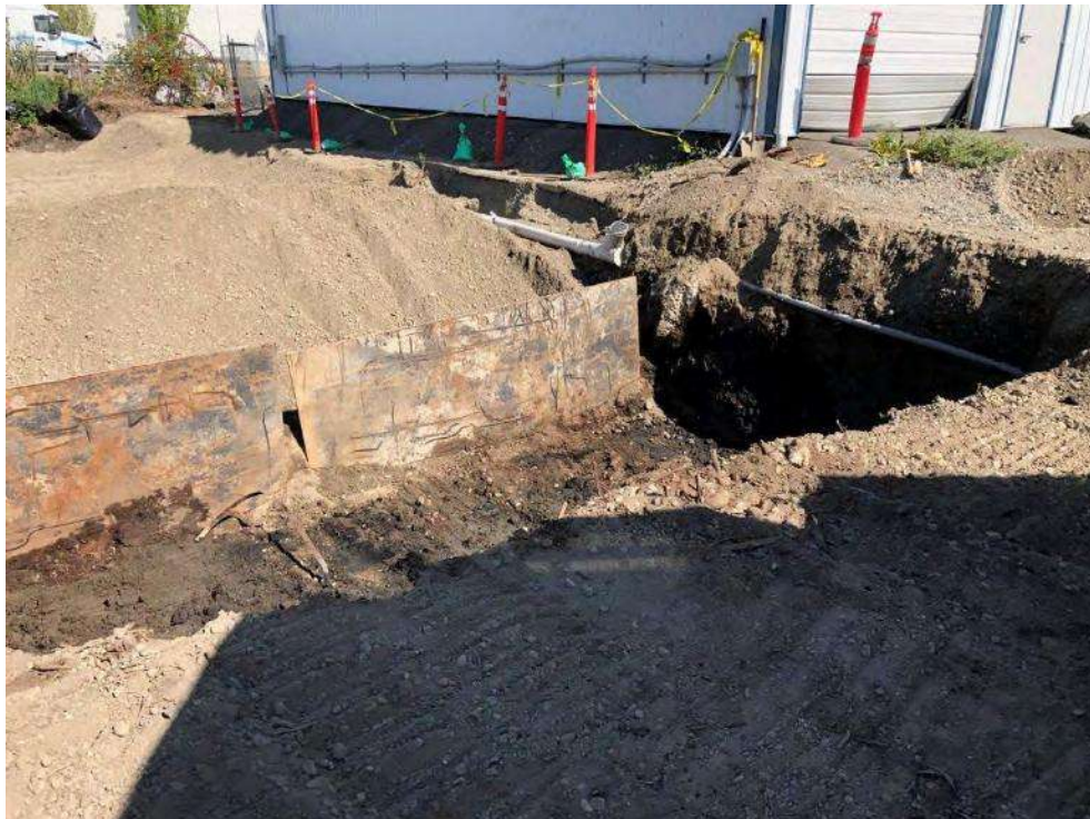
Figure 28: Bottom of RAU B7 – NOTE Steel plates used to prevent sidewall caving
