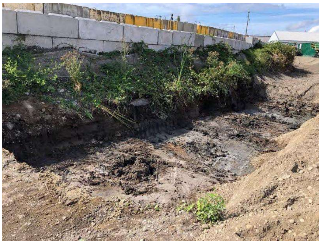
Figure 48: Bottom and western sidewall of RAU D10
