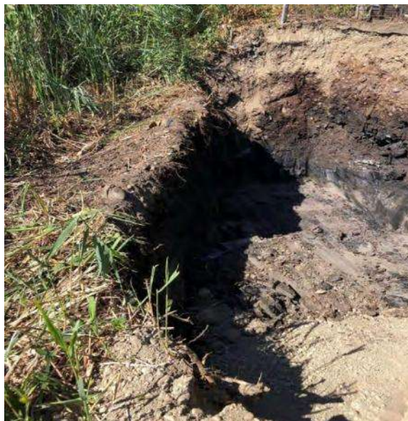
Figure 18: Bottom of RAU B1. Note oil staining in headwall
