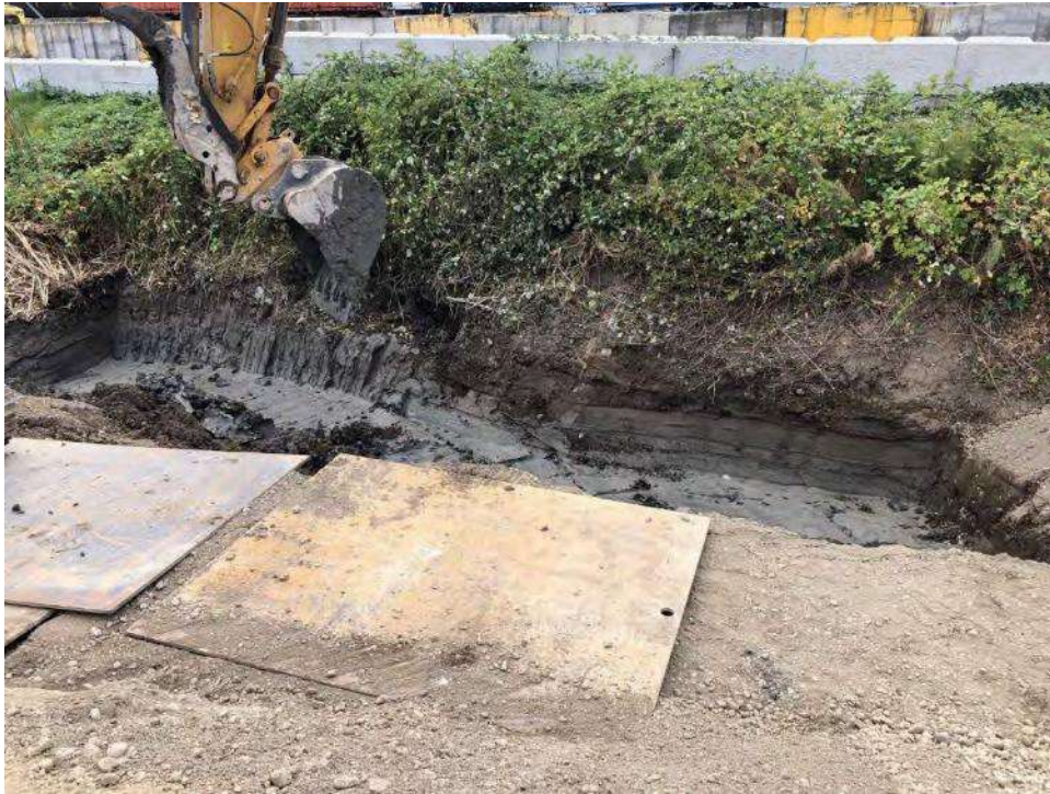
Figure 8: Western excavation limit
