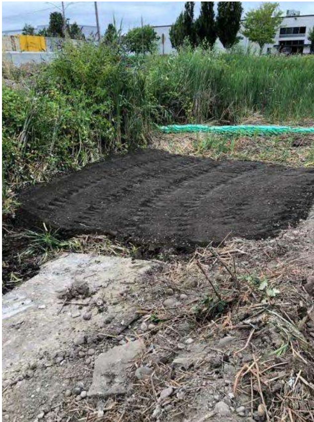
Figure 16: Typical Steam bed backfilling
