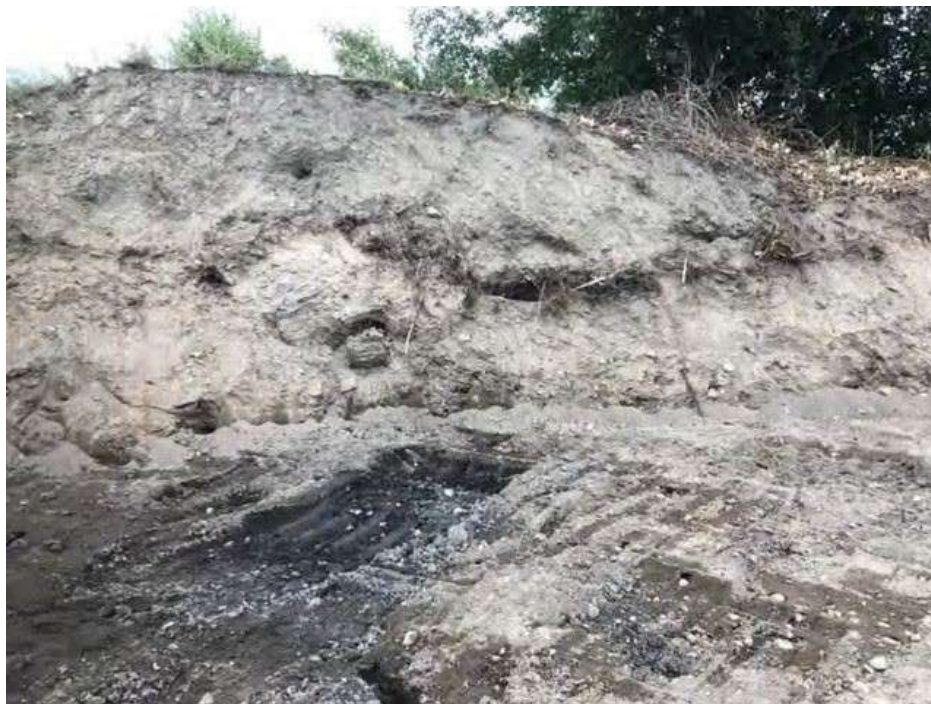
Figure 38: South wall of excavation on Port property. Sand and silt fill with rocks and concrete blocks
