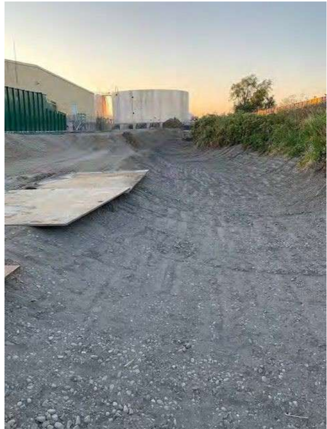
Figure 17: Completed ditch bed restoration prior to re-vegetation
