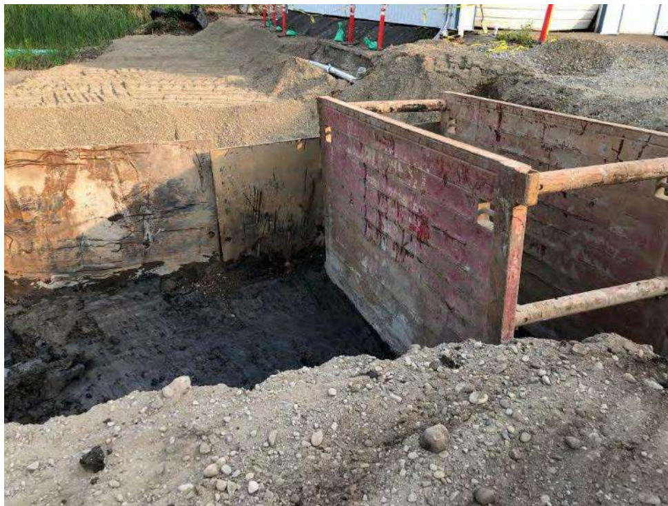
Figure 9: Use of a Trench box and steel sheeting to ensure that all impacted soils are removed and prevent caving.
