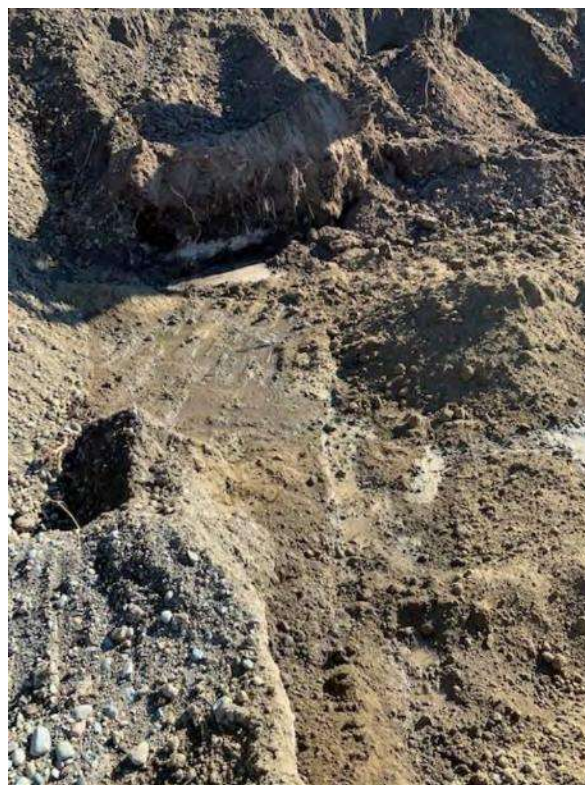
Figure 37: Excavation of RAU B14 - Note Waste water sludge as white band in sidewall
