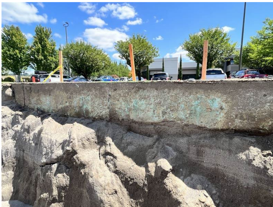
Photo 3. Oxidized copper and coarse sandy soils encountered during excavation on the eastern property are visible. Photo taken looking to the east on July 11, 2023.
