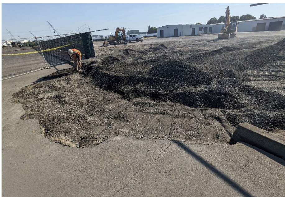
Photo 6. Following completion of excavation activities, the excavation was backfilled with compacted crushed rock.
