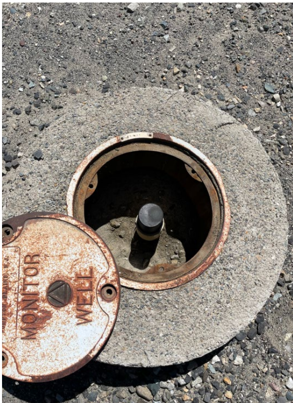
AR-09 Bioventing well, old gasket
