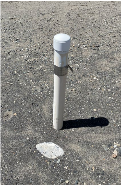
Well AR-06. No protection
