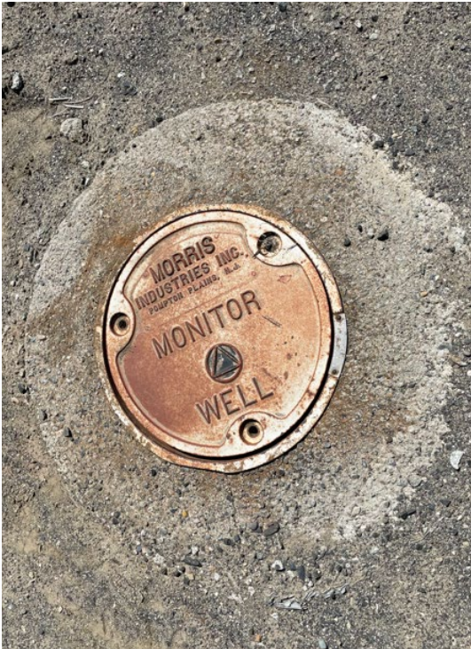
Well AR-11. No bolts
