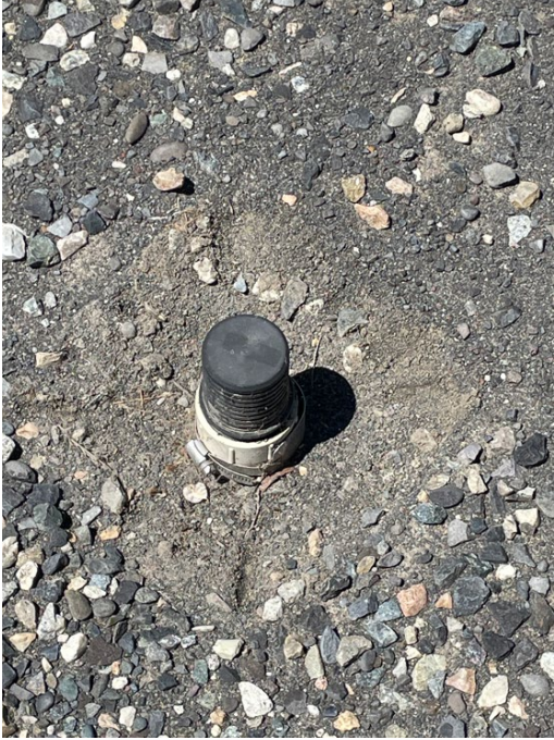
Biovent well AR-05. No protective cover or bollards.
