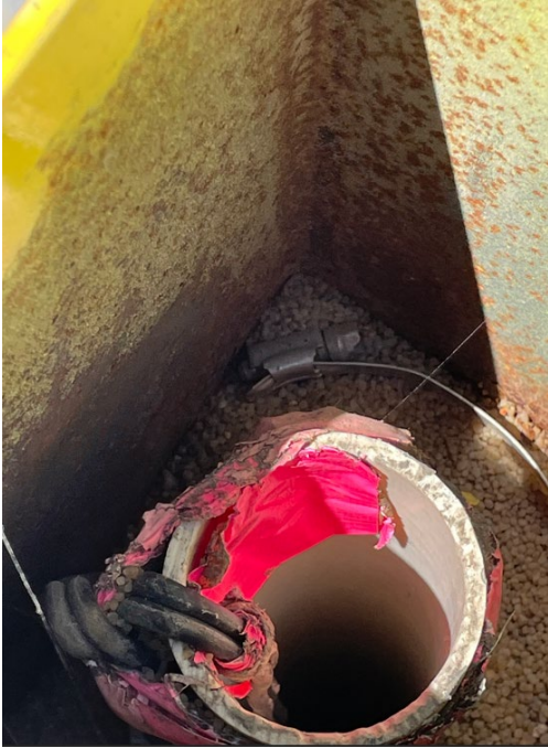
Well AR-04, with stuck pump
