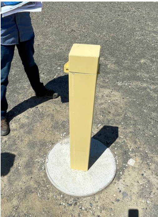
Well AR-04, well cover, no bollards
