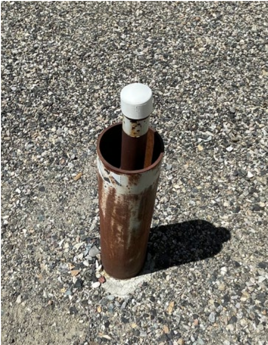
Well MW-5, No bollards, low visibility, open top
