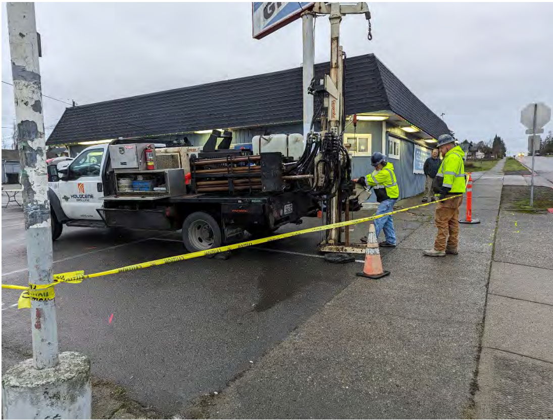
View of Boring B1, located southeast of the suspected USTs along the northeastern property boundary.
