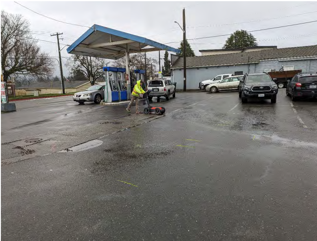
View of the ground penetrating radar survey being completed in the vicinity of the active USTs. Yellow paint identifies the locations of the current USTs.
