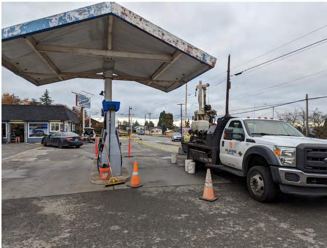
View of Boring B7, located down gradient of active fuel pumps, looking northeast.
