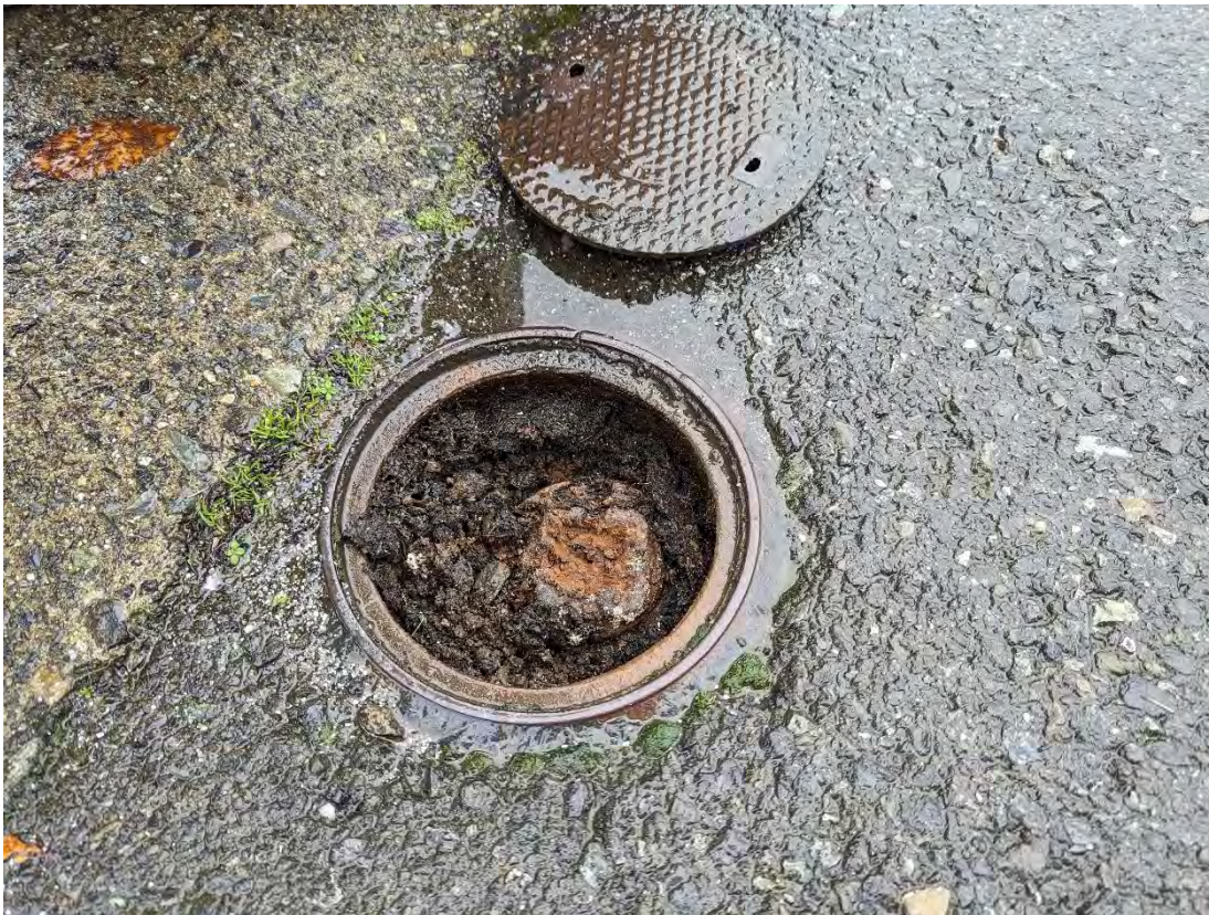
View of a suspected fill port access to the eastern UST.
