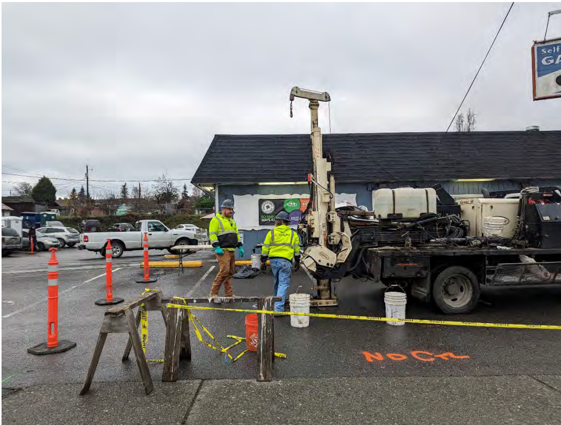
View of Boring B2, in suspected former fuel pump island for a 1940s gas station, looking northwest.
