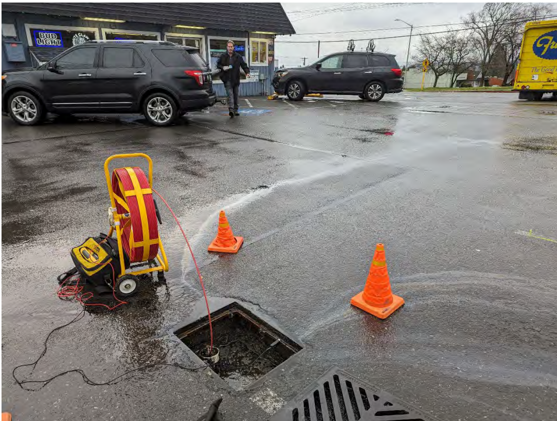
View of a cable placed within the stormwater drains to identify their underground pathway.
