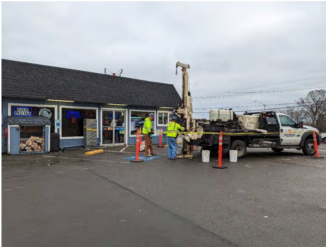
View of Boring B4, looking east. Boring was completed between the building and the active USTs.
