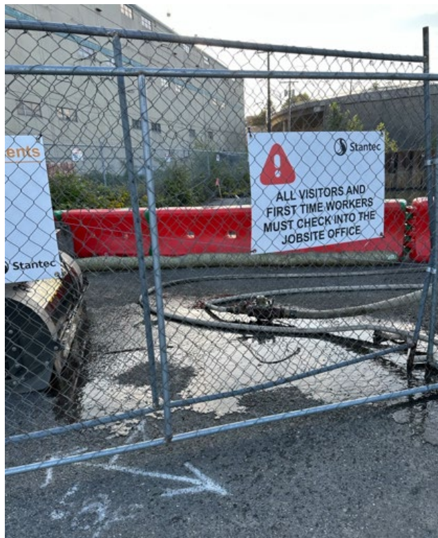
Photo 2. Wattle Placed Around Excavation to Keep Sediment From Leaving the Site.
