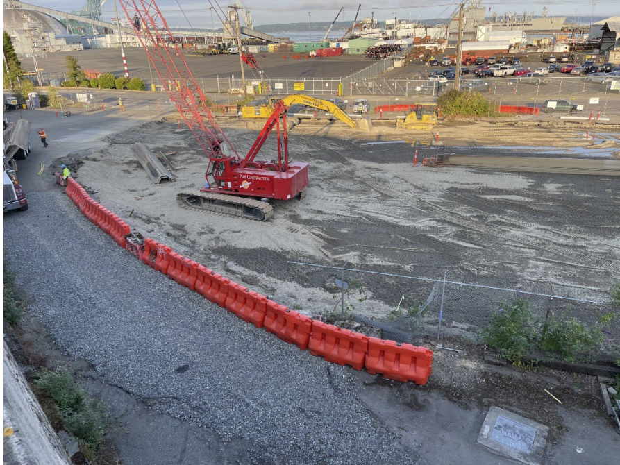
Photo 3. Edge of Excavation Sloped so that Potential Stormwater Runs off into the Excavation.
