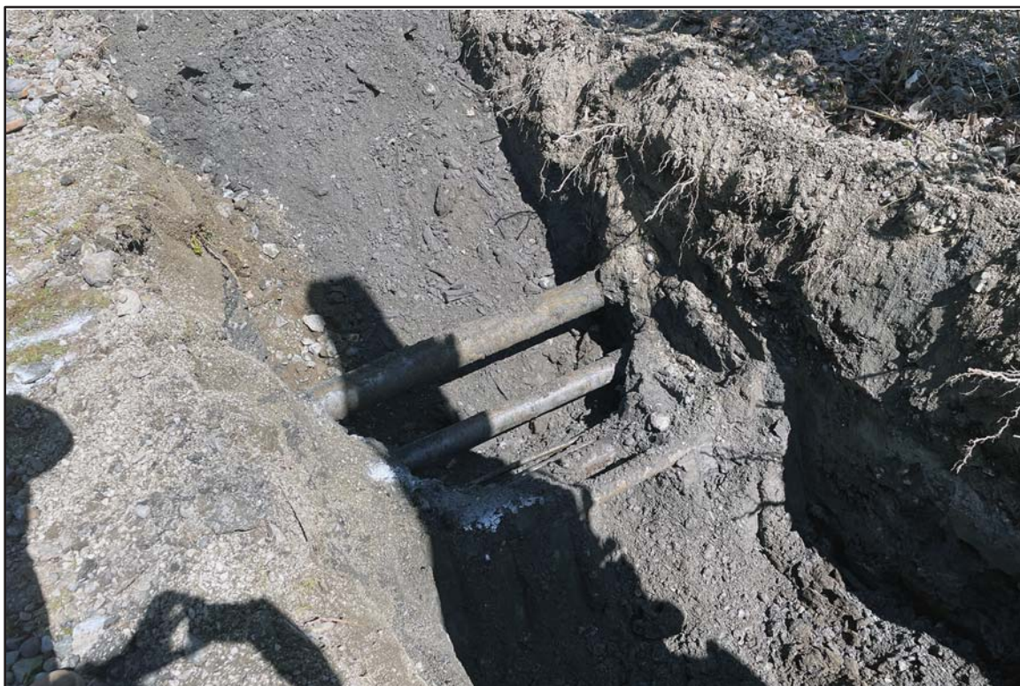
Photo 3. Example of exploratory trenching along the east project boundary showing previous utilities disturbance. View to the northeast.
