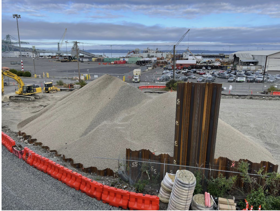
Photo 3. Stockpile on Soil Sloped so that Stormwater Runs off into the Excavation.
