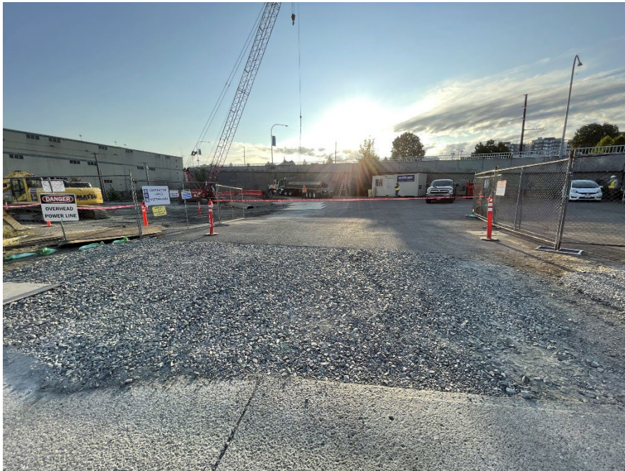
Photo 4. Quarry Spalls at Site Entrance.
