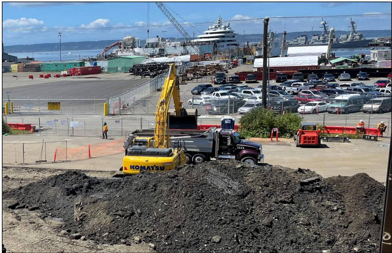
Photograph 7 Temporary Soil Stockpiling
