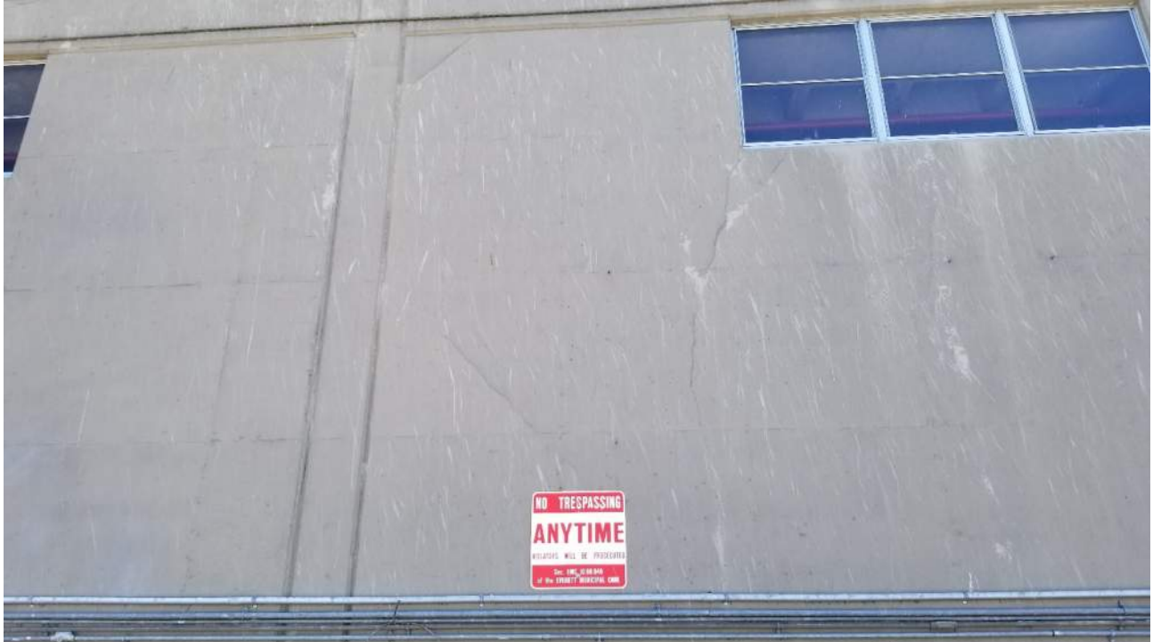
P1.13 – Cracking at panel corner and panel opening on west face of Kimberly Clark Building
