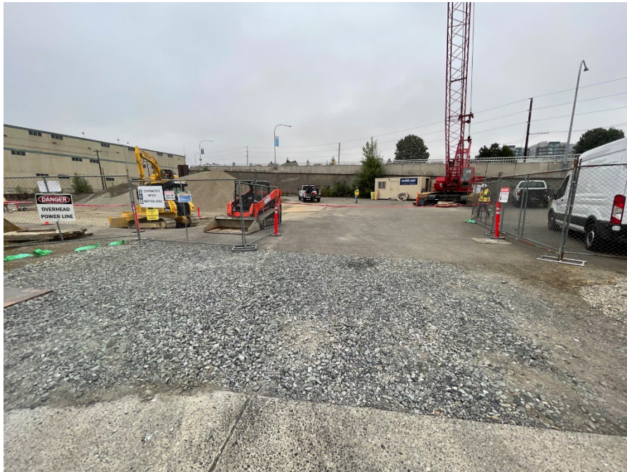
Photo 4. Quarry Spalls at Site Entrance.
