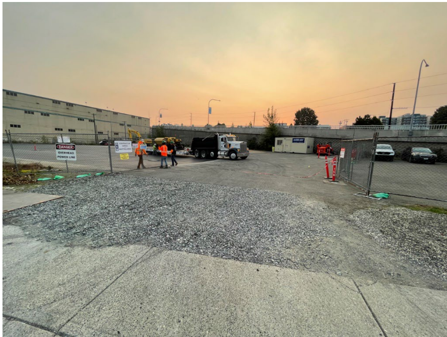
Photo 4. Quarry Spalls at Site Entrance
