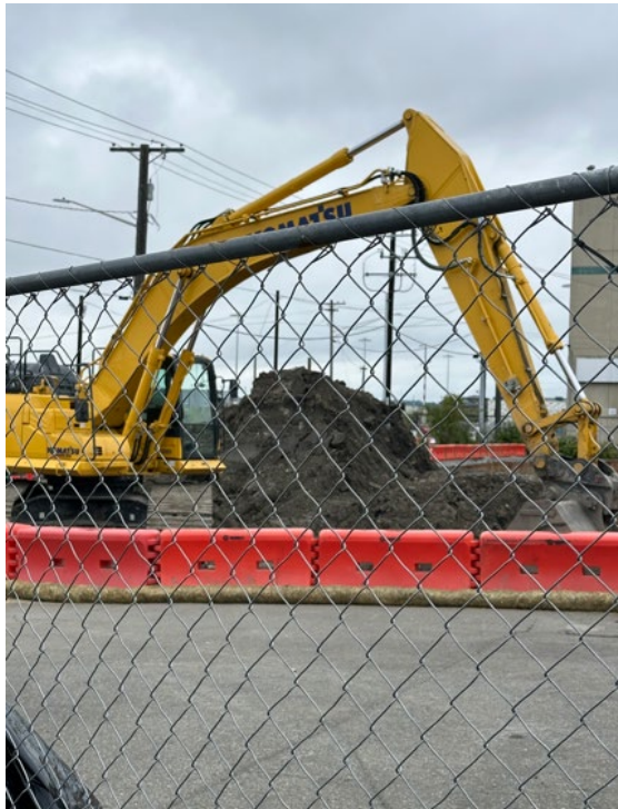
Photo 2. Stockpile of Soil Sloped so that Stormwater Runs off into the Excavation.
