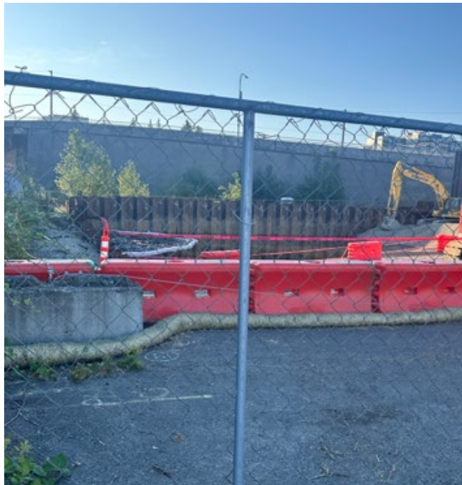
Photo 2. Wattle Placed Around Excavation to Keep Sediment From Leaving the Site.
