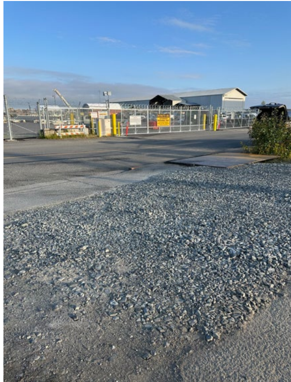
Photo 3. Quarry Spalls at Entrance of Site to Keep Sediment off of Street.
