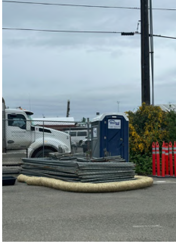
Photo 3. Wattle Set Aside from Stockpile before Weekend. It was Dirty and No Rainfall was Expected.
