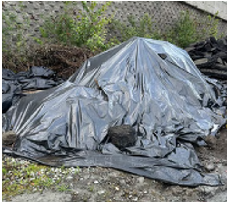
Photo 2. Stockpile Covered and Weighted Down.
