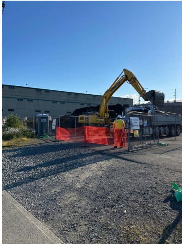
Photo 3. Quarry Spalls at Entrance of Site to Keep Sediment Run Off into Street.
