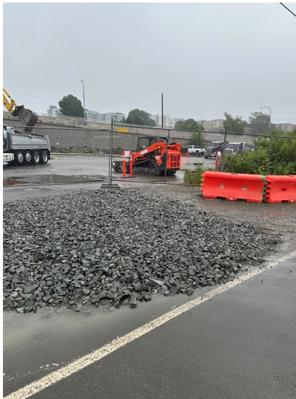
Photo 4. Quarry Spalls at Entrance of Site to Keep Sediment From Tires from Being Tracked onto the Road.
