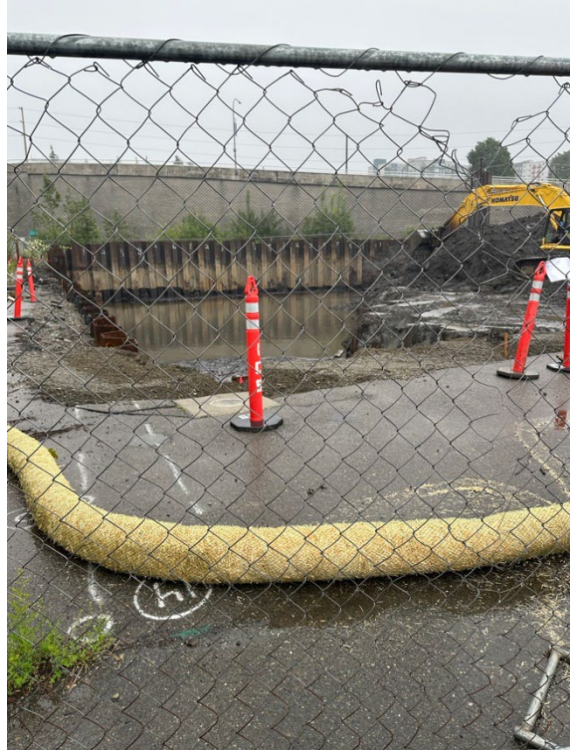
Photo 3. Straw Wattles Placed Around Excavation to Catch Sediment.
