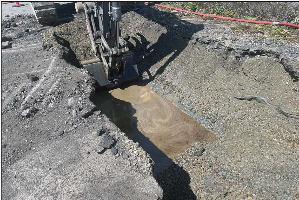
Photo 2. Example of exploratory trenching along the east project boundary showing typical gravel fill. View to the northeast.
