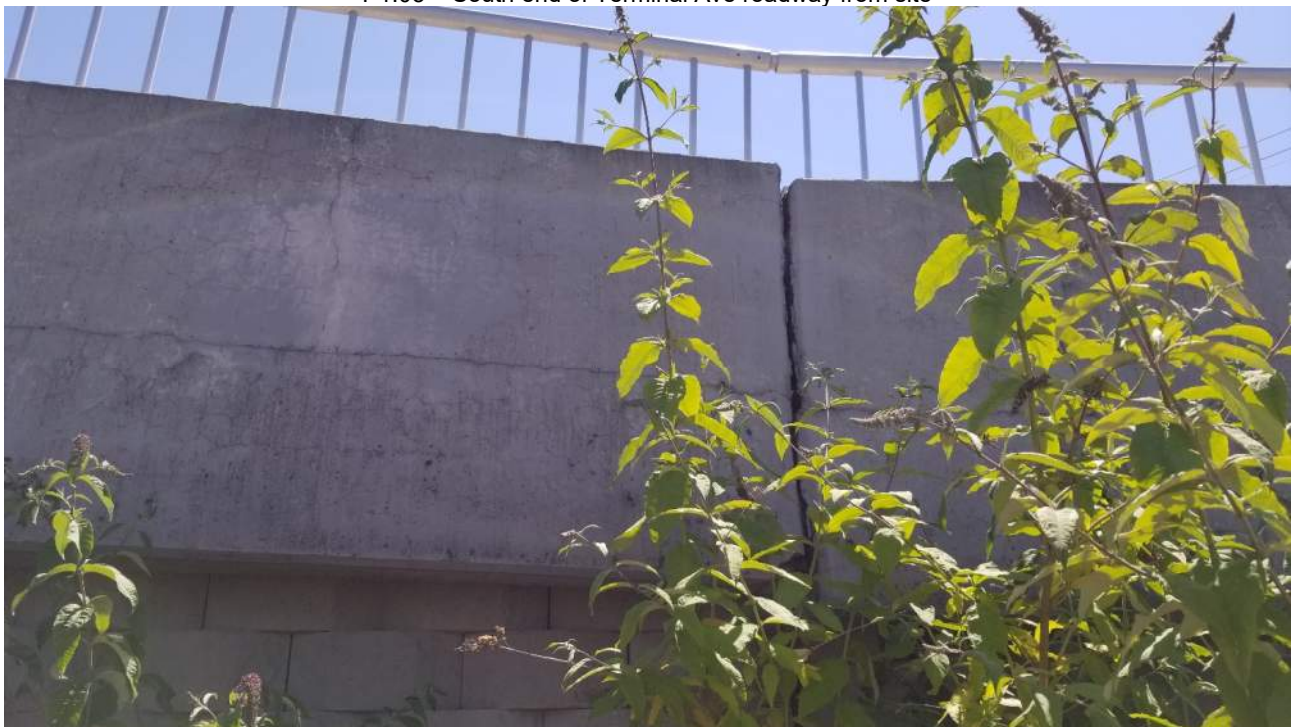
P1.06 – Movement at joint and shrinkage cracking in Terminal Ave Bridge
