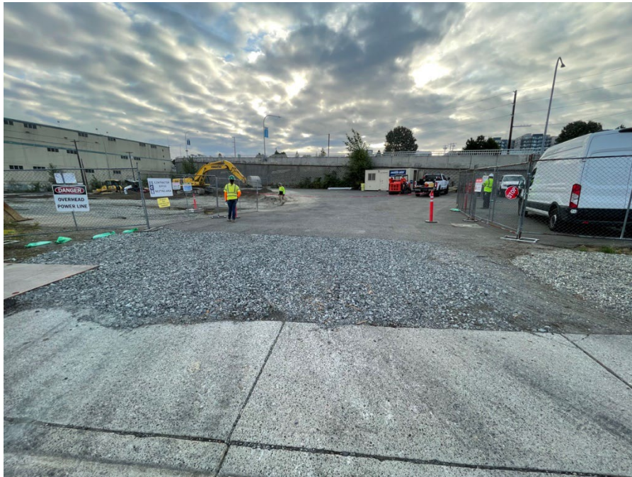
Photo 4. Quarry Spalls at Site Entrance.
