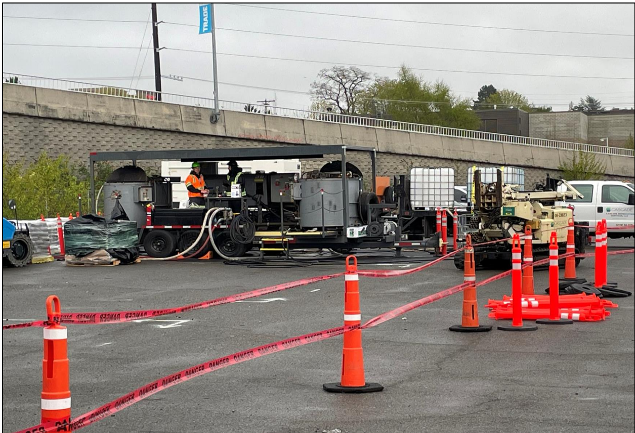
Photograph 2 In-situ Soil Stabilization Grout Plant & Direct Push Drill Rig
