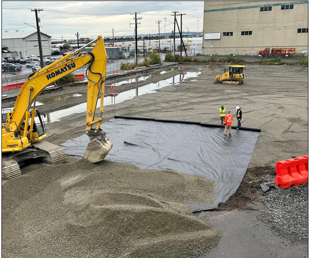
Photograph 11 Installation of Geotextile Fabric
