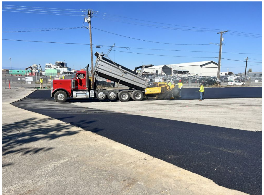
Image 2: Placement of HMA
