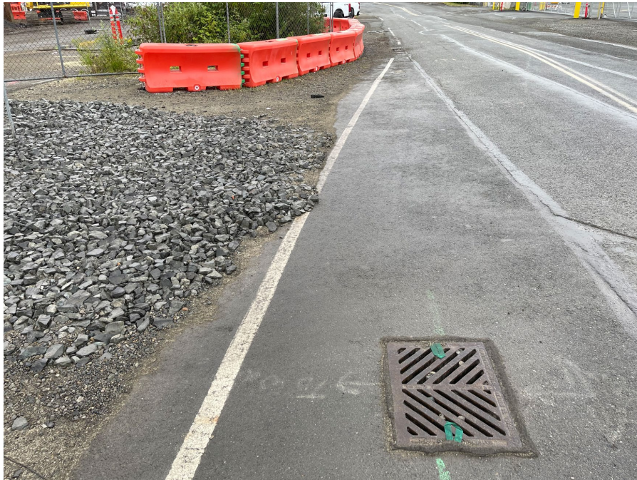
Photo 4. Quarry Spalls at Entrance of Site and Street Swept Road.
