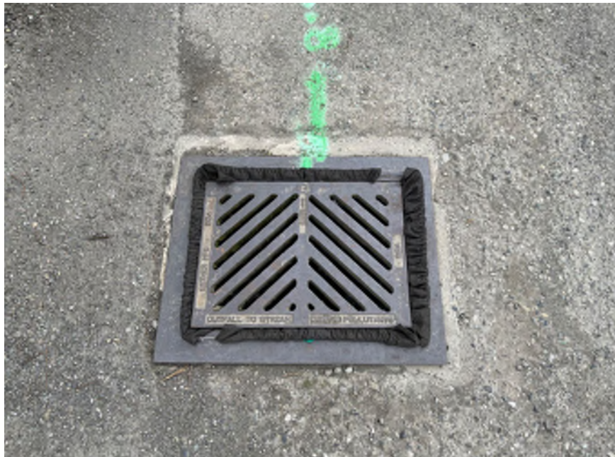
Photo 2. Functioning Silt Sock in Storm Drain.
