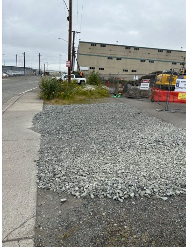
Photo 3. Quarry Spalls at Entrance of Site to Keep Sediment off Street.
