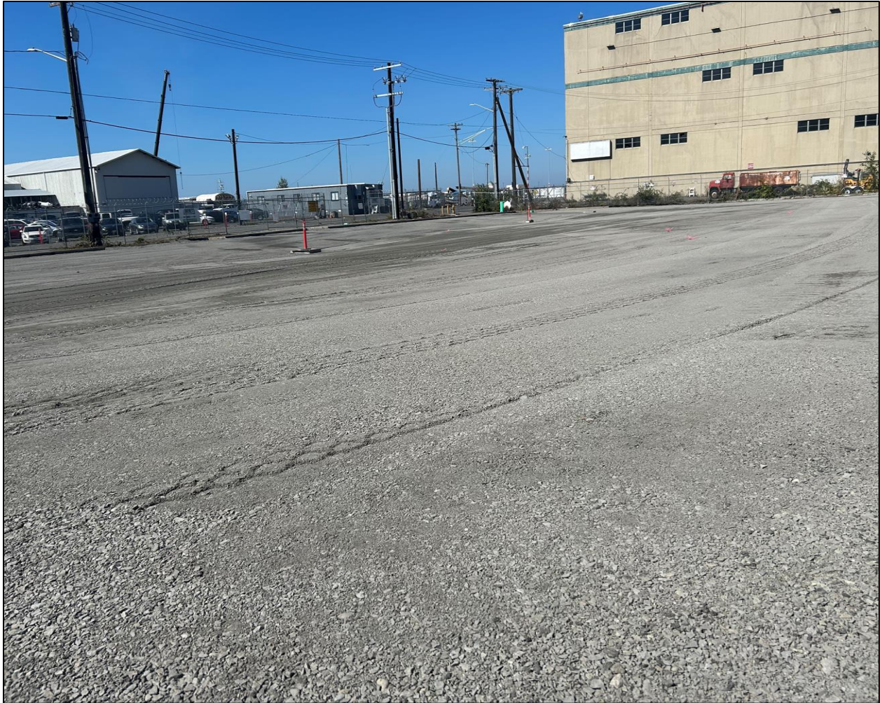
Photograph 12 Compacted Aggregate Base
