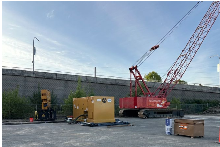
Photo 2. Equipment with BMP Underneath to Catch Leakage.
