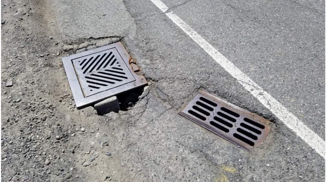
P1.17 – Failed drain on Federal Avenue
