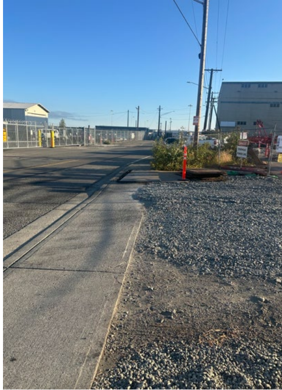
Photo 3. Quarry Spalls at Entrance of Site to Keep Sediment off of Street.
