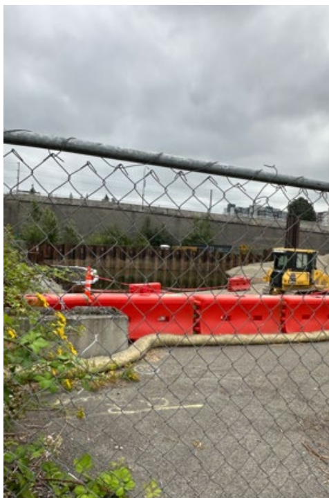
Photo 2. Wattle Placed Around Excavation to Keep Sediment From Leaving the Site.
