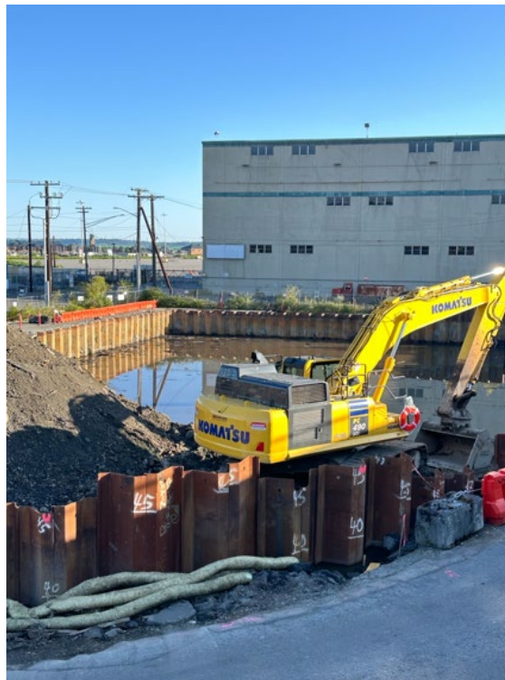
Photo 2. Stockpile on Soil Sloped so that Stormwater Runs off into the Excavation.
