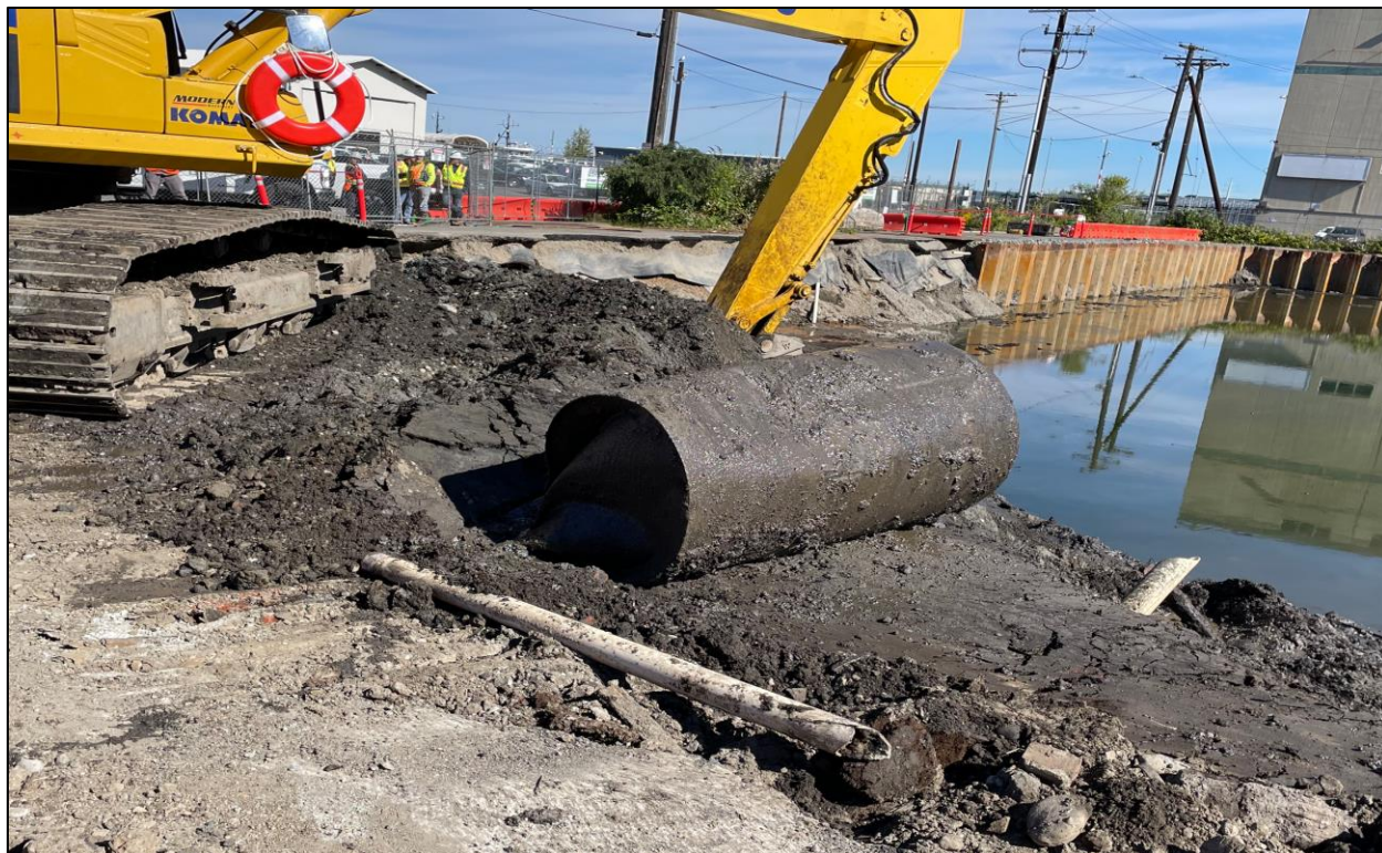
Photograph 16 Heating Oil UST Discovery and Removal
