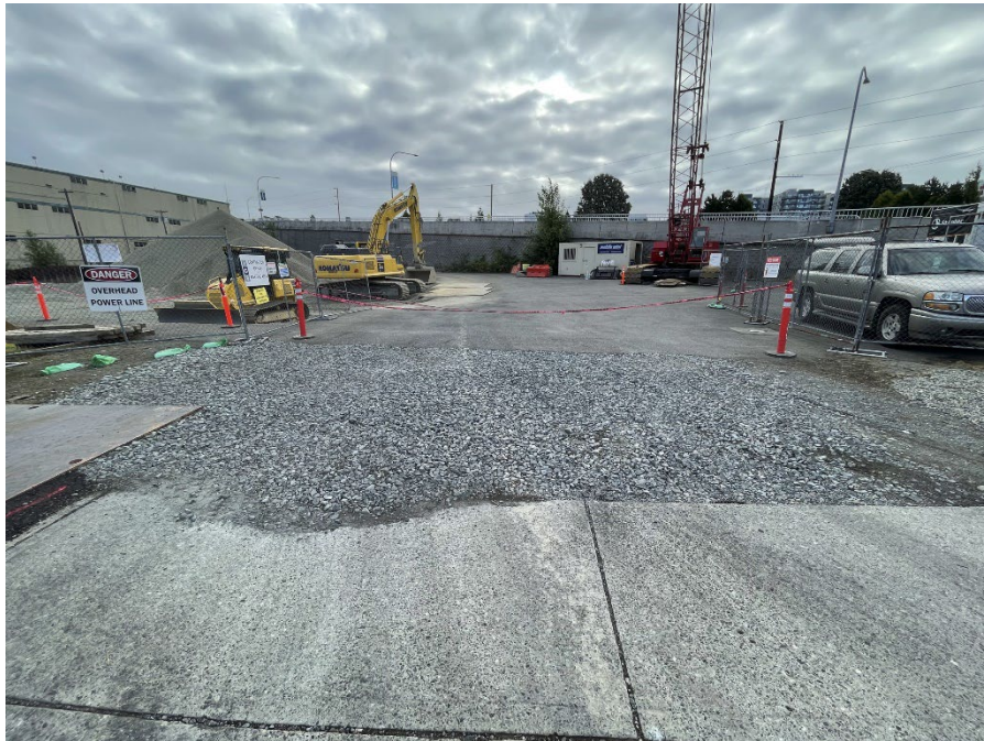
Photo 4. Quarry Spalls at Site Entrance.
