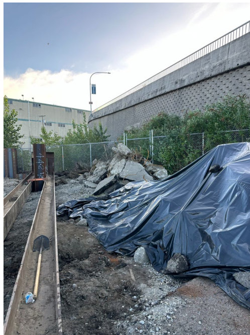
Photo 2. Cement Stockpiles Covered and Stored Away from Drain Inlets.
