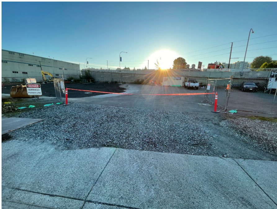
Photo 4. Quarry Spalls at Site Entrance
