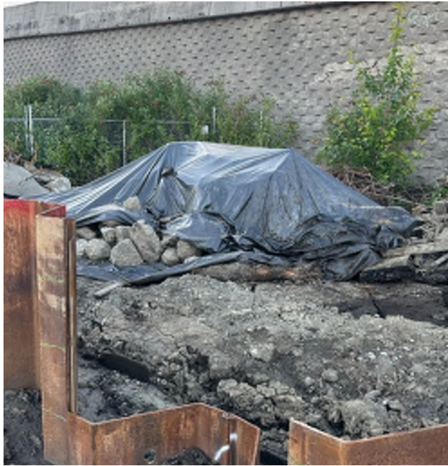
Photo 3. Cement Stockpile Covered and Stored Away from Storm Drain Inlet.
