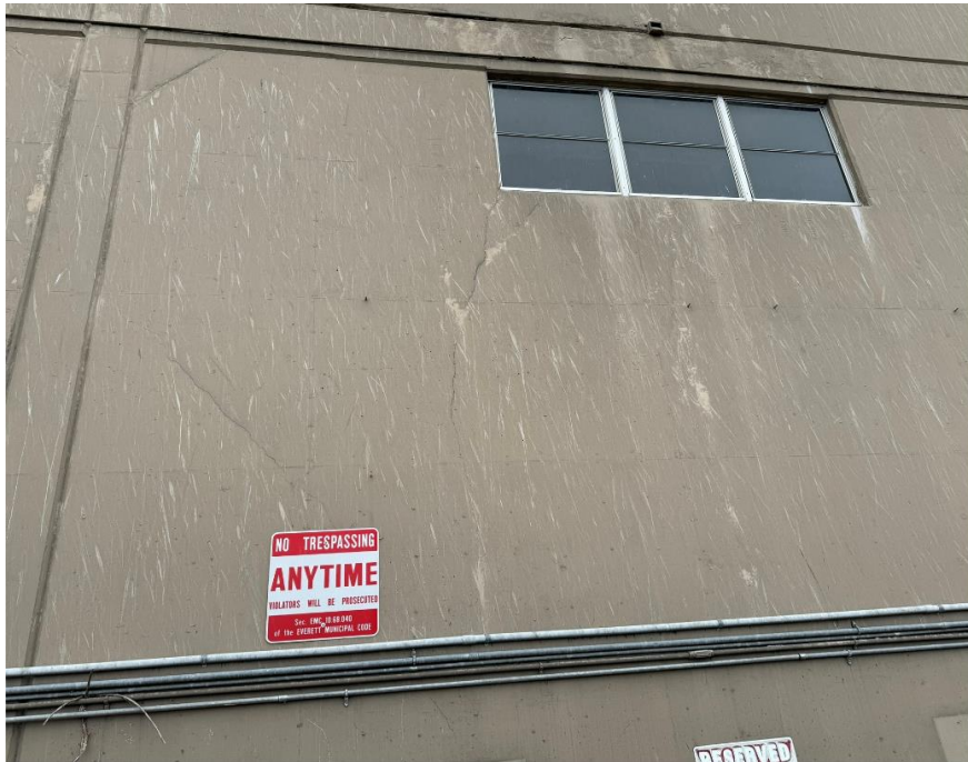
P2.07 – Cracking at panel corner and panel opening on west face of Kimberly Clark Building
