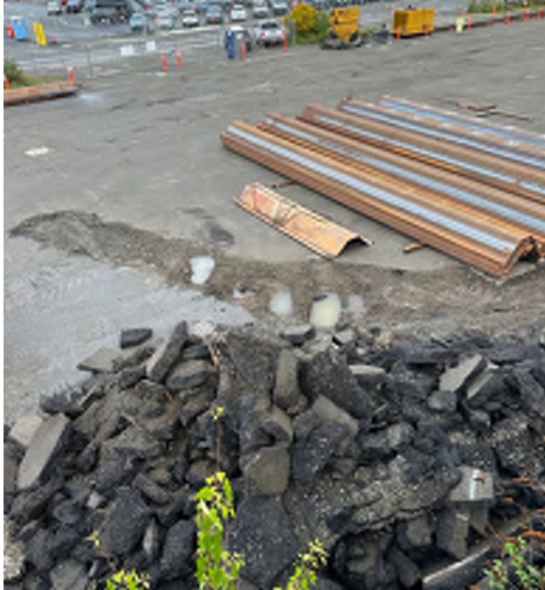
Photo 3. Stockpile Trench Catching Storm Water Runoff.
