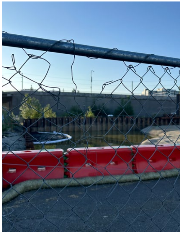
Photo 2. Wattle Placed Around Excavation to Keep Sediment From Leaving the Site.
