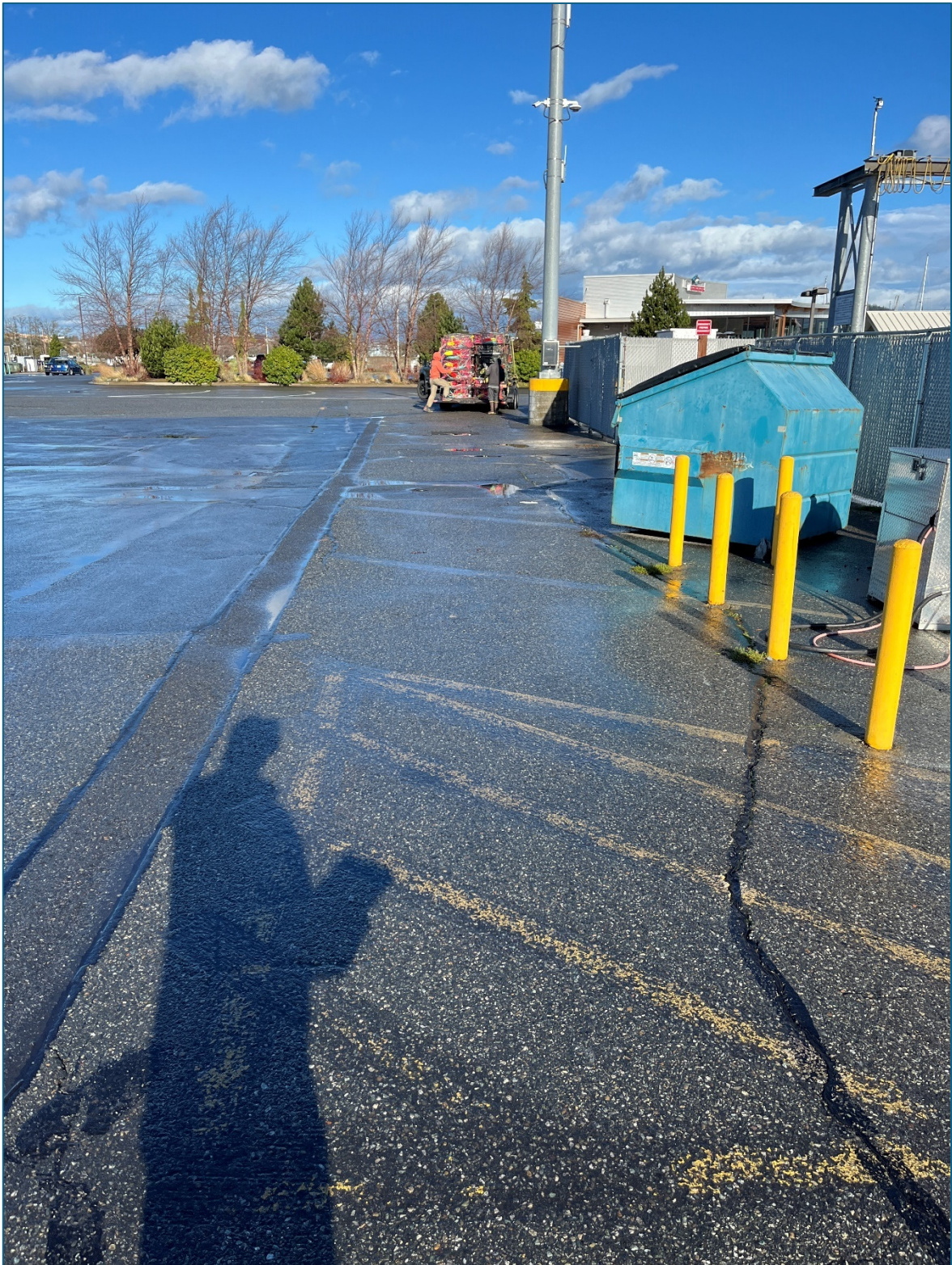
Figure 4: Photo monitoring point A3 looking N towards Anthony's Trailer Boat Launch
