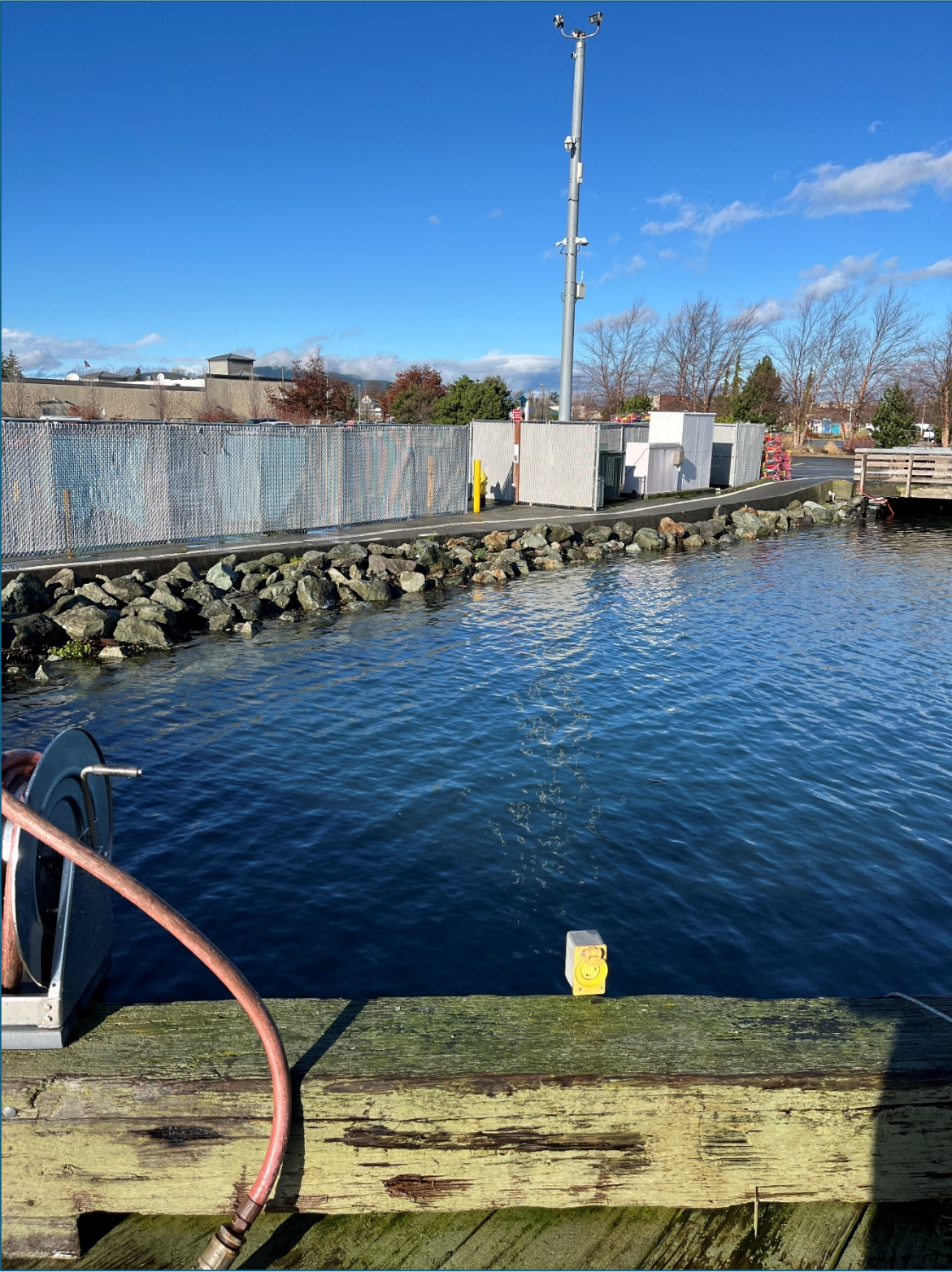
Figure 5: Photo monitoring point A4 looking NW towards Cap Sante Marina uplands, view occluded by trash enclosures and electrical infrastructure.
