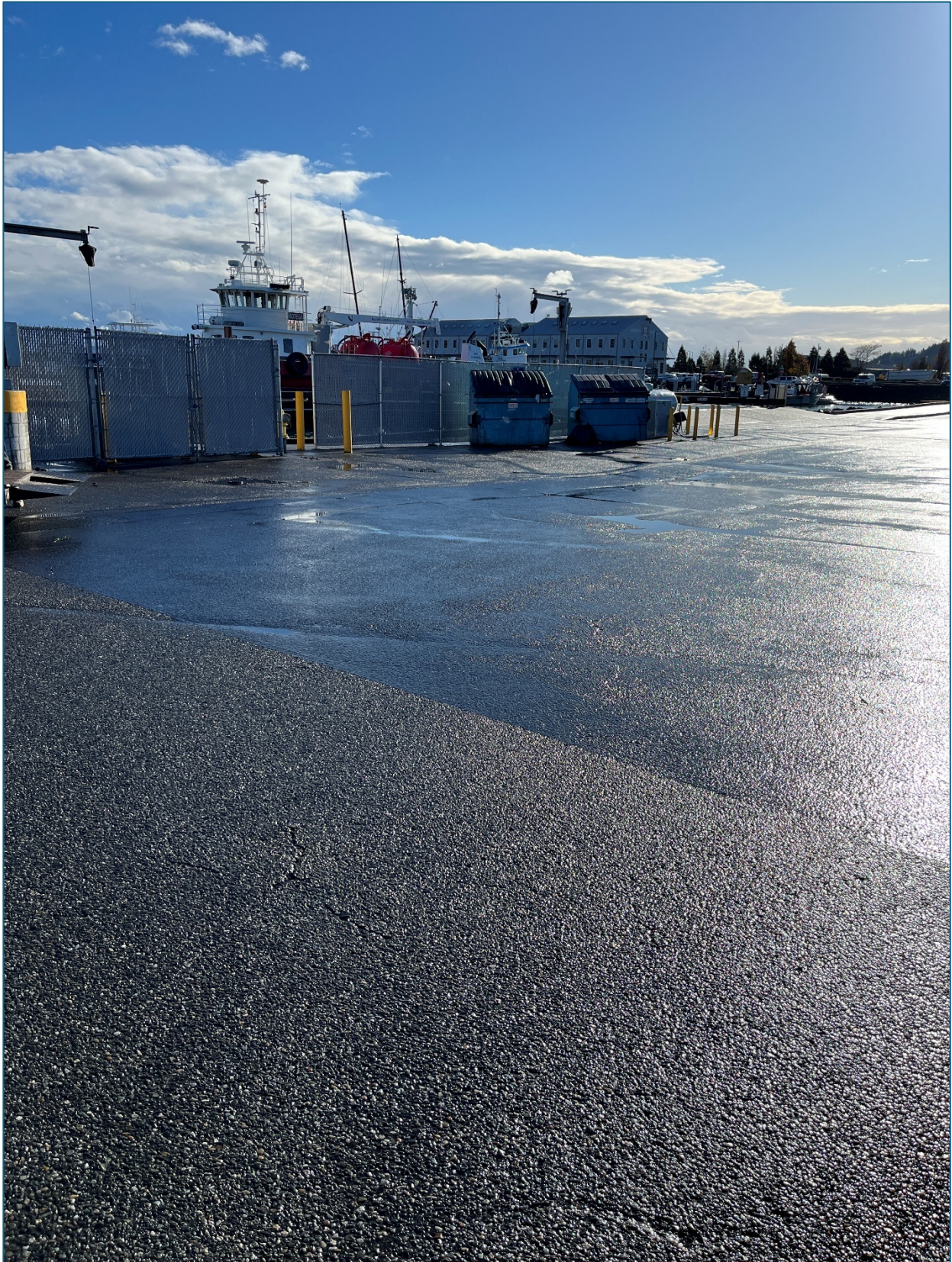
Figure 2: Photo monitoring point A1 looking SE towards T-Dock
