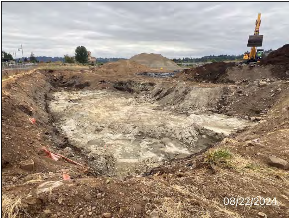
Photo 11: Excavation area along the proposed roadway area and southern portion of Building B, facing west, 8/22/24.
