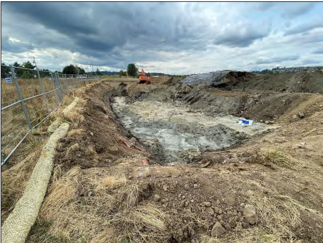
Photo 6: Excavation area along the proposed roadway area south of Building B, facing east, 8/15/24.
