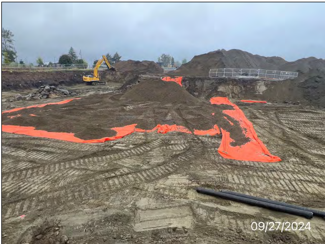
Photo 36: Laying out demarcation fabric and stockpiling structural fill within excavation, facing west, 9/27/24.
