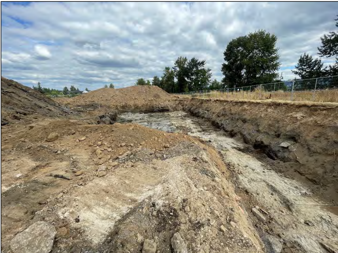
Photo 2: Excavation area along the proposed roadway area south of Building B, facing east, 8/12/24.
