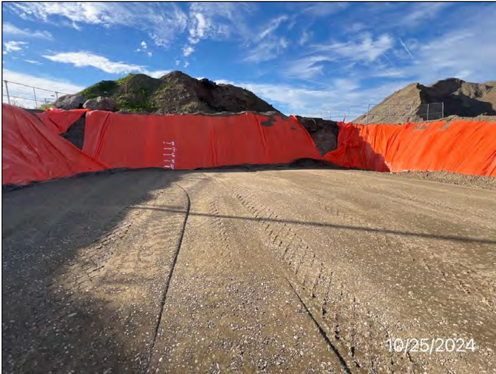
Photo 51: Replaced and compacted fourth lift within the southwestern corner of the excavation, facing west, 10/25/24.
