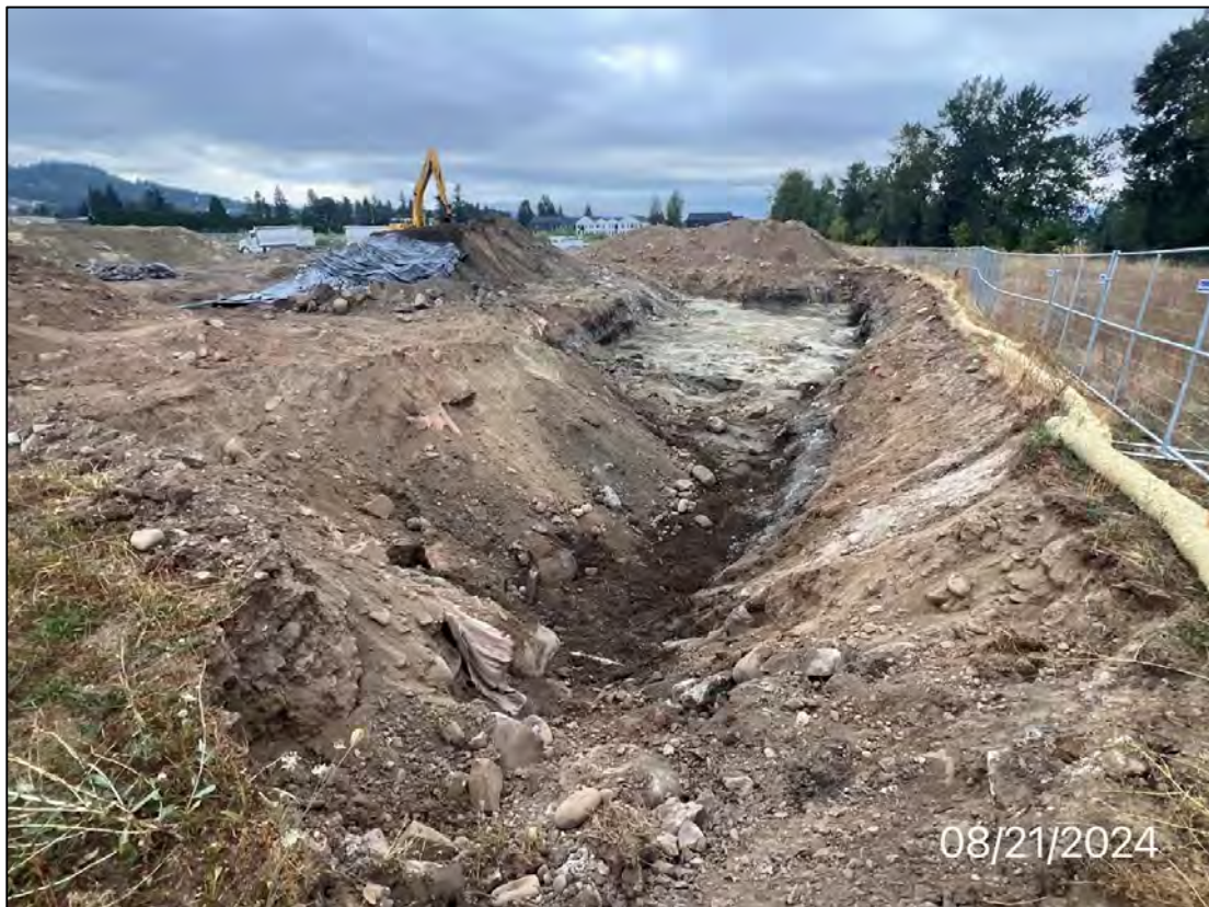
Photo 10: Excavation area along the proposed roadway area and southern portion of Building B, facing east, 8/21/24.
