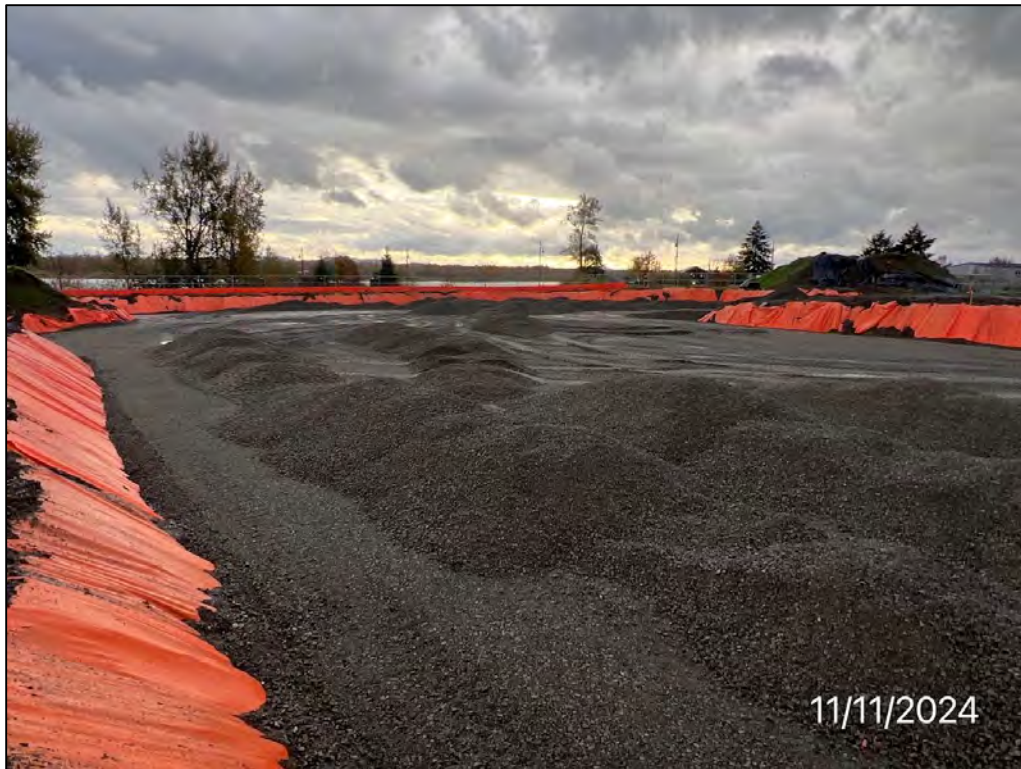
Photo 61: Stockpiling structural backfill within the excavation prior to spreading and compacting, facing southwest, 11/11/24.
