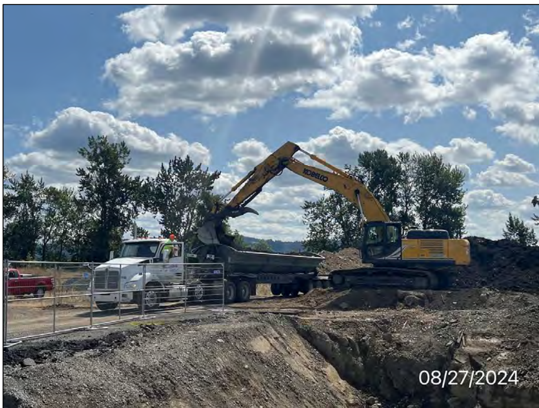
Photo 13: Loading impacted soil into haul truck for disposal off site, facing south, 8/27/24.
