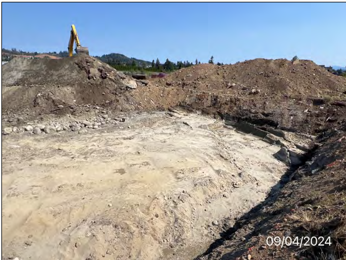
Photo 18: Excavation area in the vicinity of the roadway area and Building B, facing northeast, 9/4/24.
