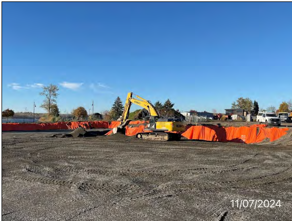
Photo 57: Saturated structural backfill being removed along the western portion of the excavation due to greater than optimal moisture content, backfill work did not occur on this date, facing west, 11/7/24.
