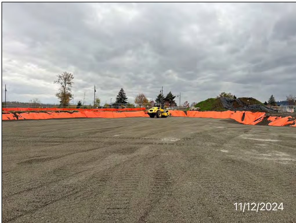
Photo 62: Compacting structural backfill within the southwestern portion of the excavation, facing southwest, 11/12/24.
