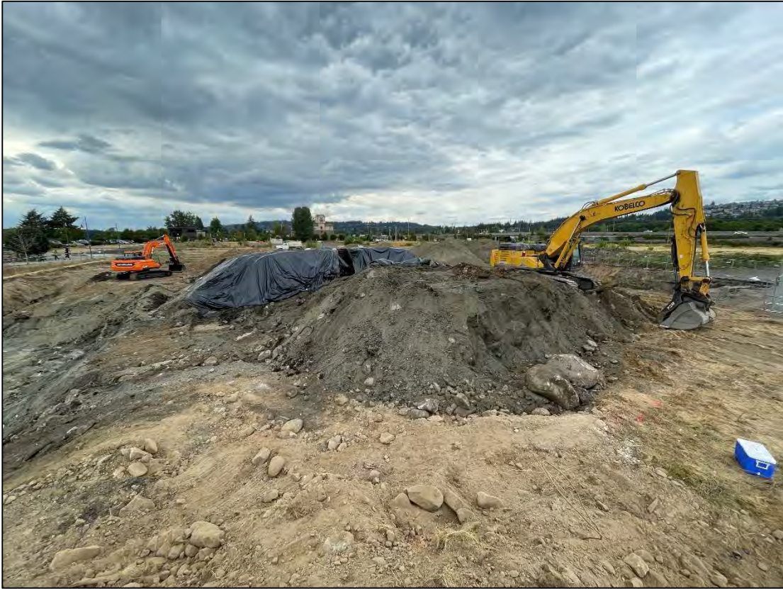
Photo 5: Stockpiled impacted soil staged for loading into trucks to be hauled off site, facing west, 8/15/24.
