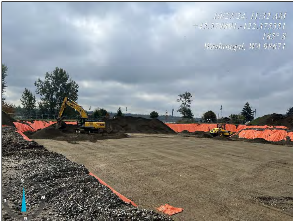
Photo 49: Recompacting the third and fourth lifts within the northern portion of the excavation after retesting the first and second lifts, facing south, 10/23/24.
