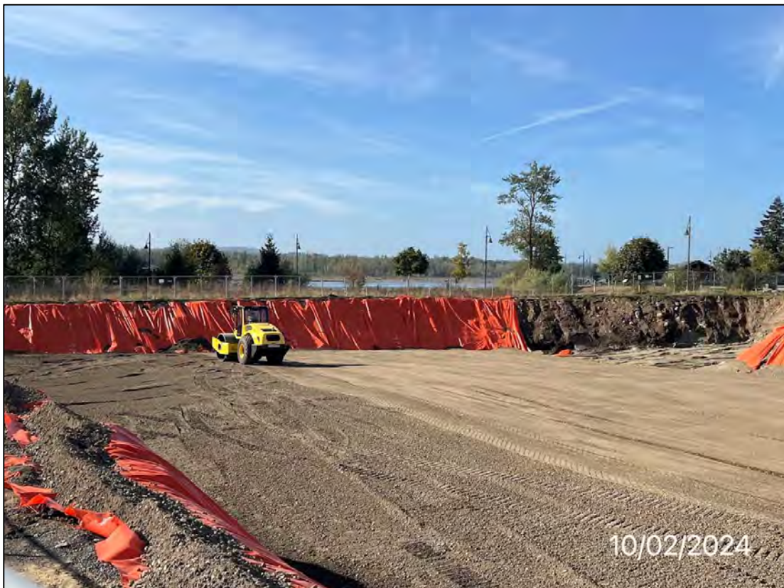
Photo 40: Compacting second lift, facing southwest 10/2/24.
