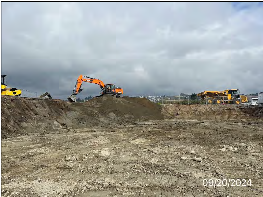
Photo 32: Excavating “organic” soils from northern portion of Building B, facing north, 9/20/24.
