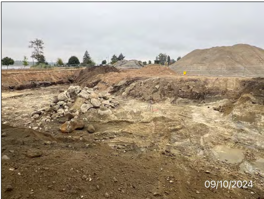
Photo 22: Boulder pile staged for removal from excavation, facing west, 9/10/24.
