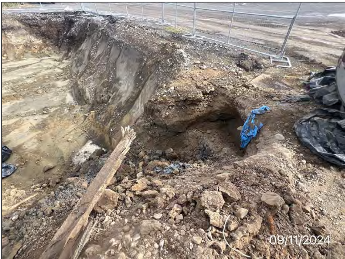
Photo 24: Excavation area in the vicinity of the UST, facing east, 9/11/24.
