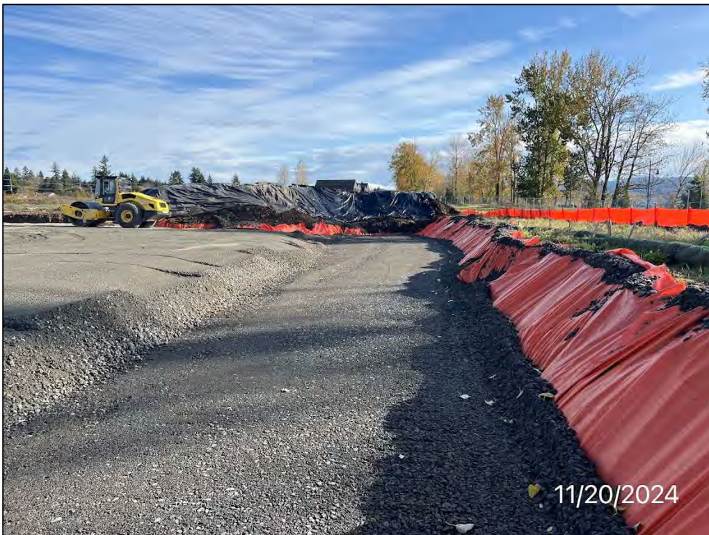
Photo 66: Conditions within the southern portion of the excavation on this date, facing east, 11/20/24.
