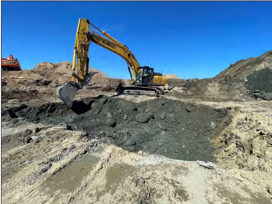
Photo 15: Excavation area in the vicinity of the southwest corner of Building B, removing impacted soils to a depth of approximately 15 feet bgs, facing north, 8/28/24.
