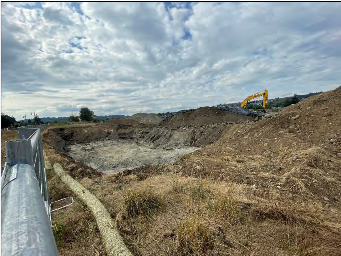
Photo 8: Excavation area along the proposed roadway area and southern portion of Building B, facing east, 8/16/24.
