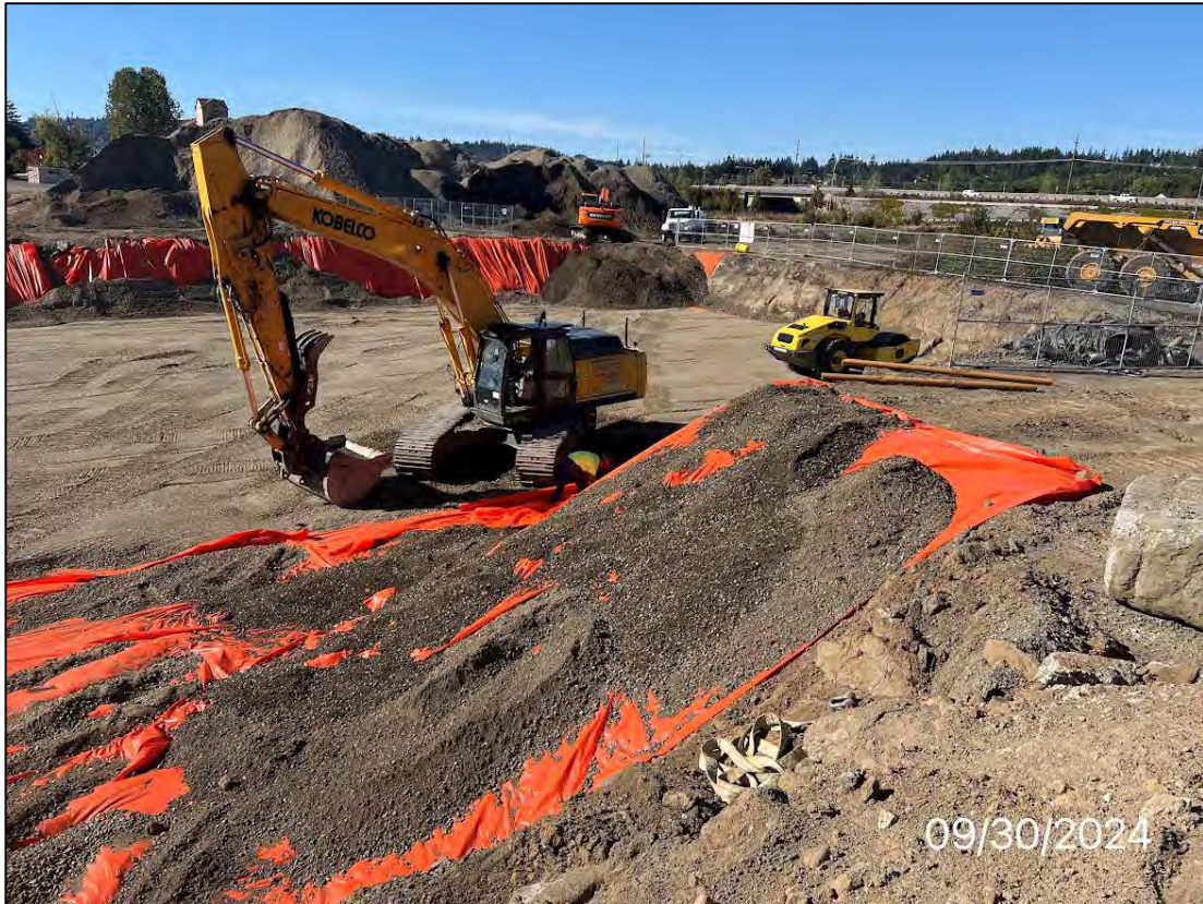
Photo 37: Lay out of demarcation fabric and the initial (<1 foot) lift of structural backfill in order to compact the underlying subgrade, facing northwest, 9/30/24.
