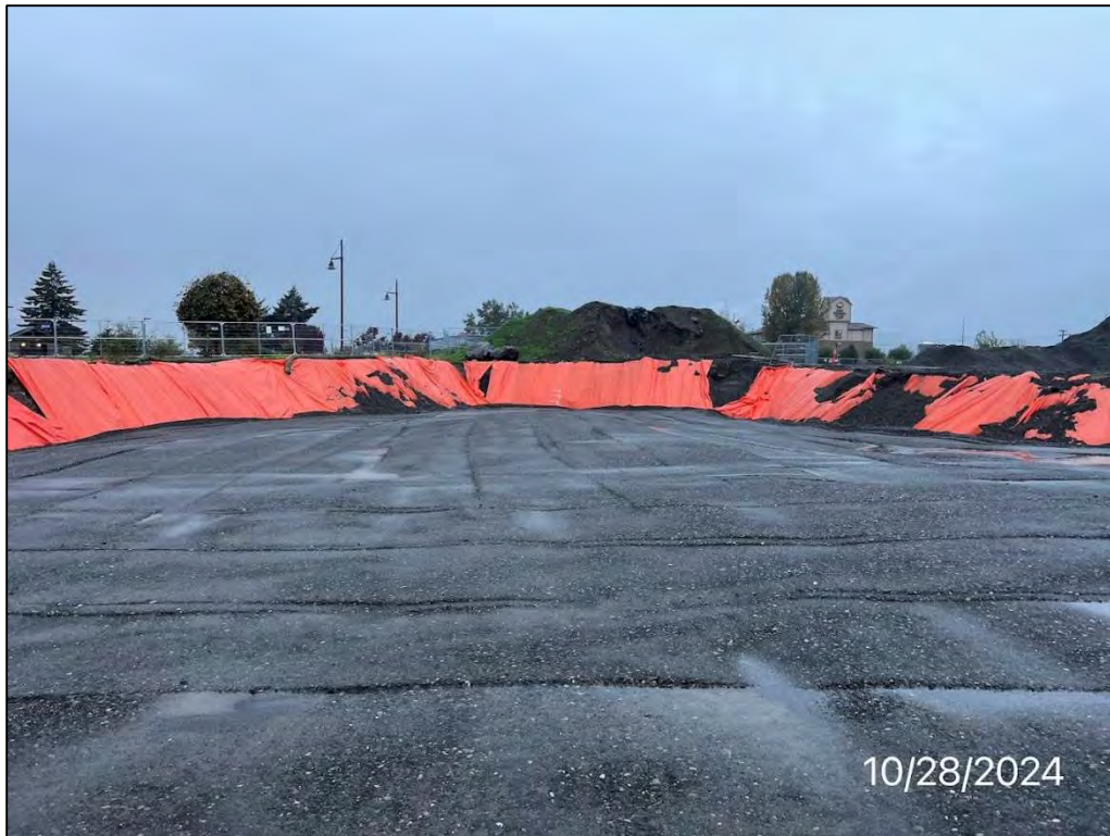
Photo 53: Precipitation on this date caused structural backfill to have a greater than optimal moisture content, backfill work was paused to wait for drier conditions, facing west, 10/28/24.
