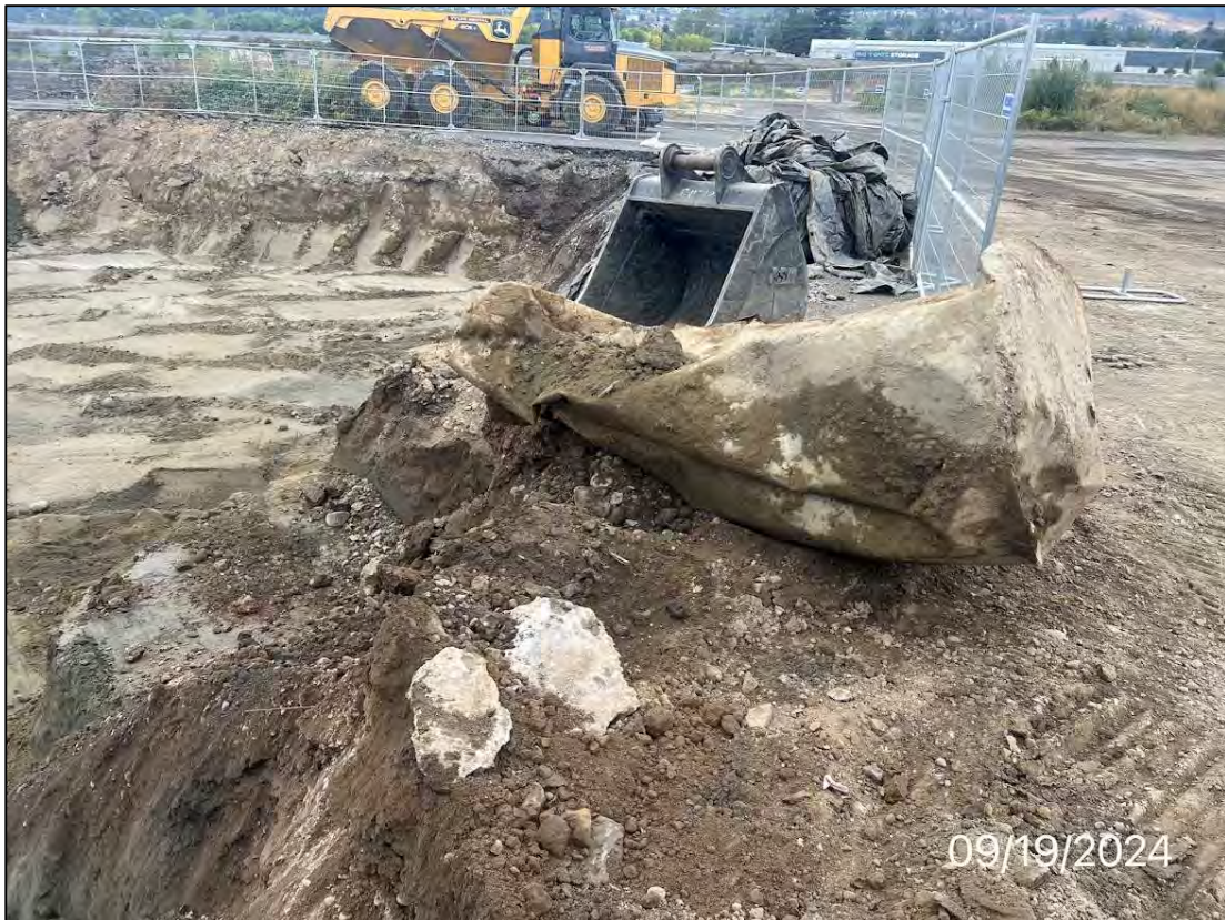
Photo 31: UST staged for removal from site, facing north, 9/19/24.
