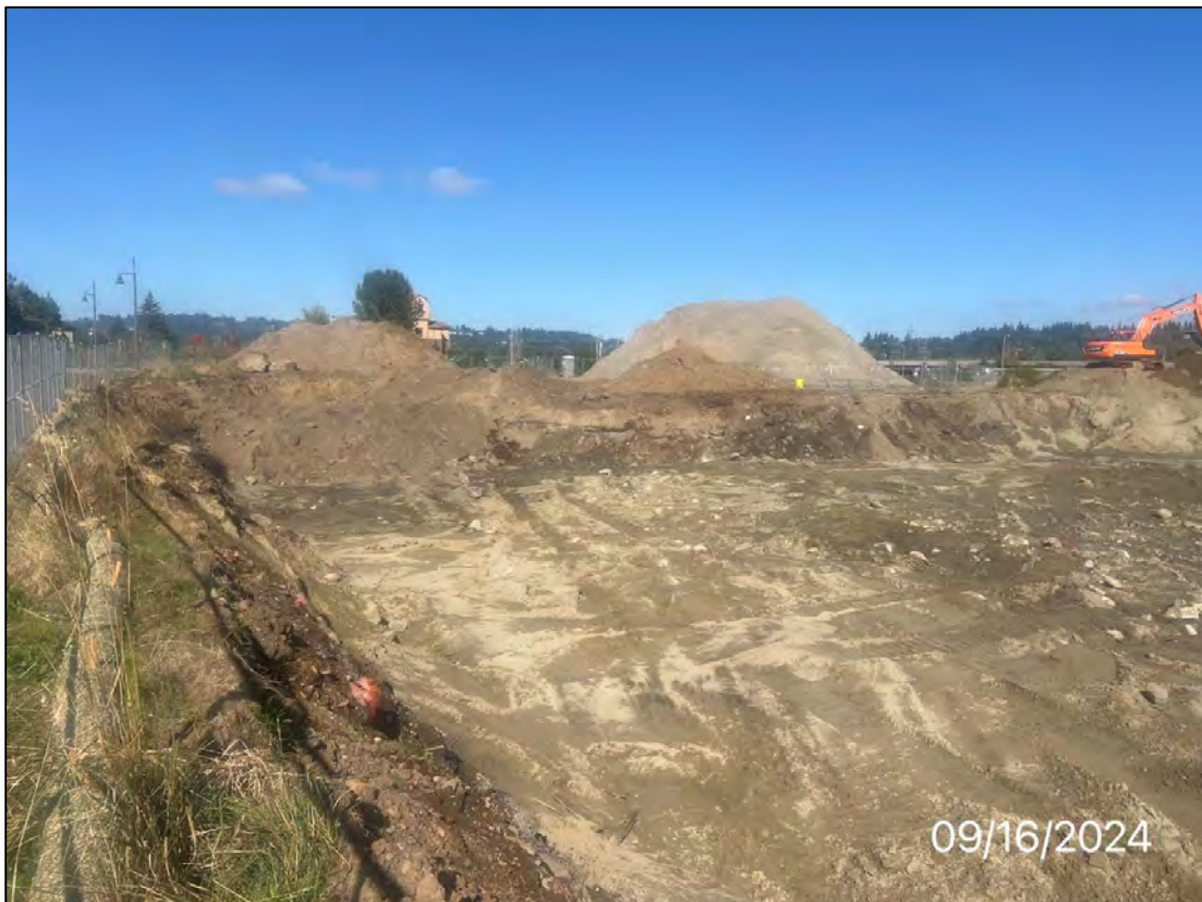
Photo 28: Excavation area looking west, facing east, 9/16/24.
