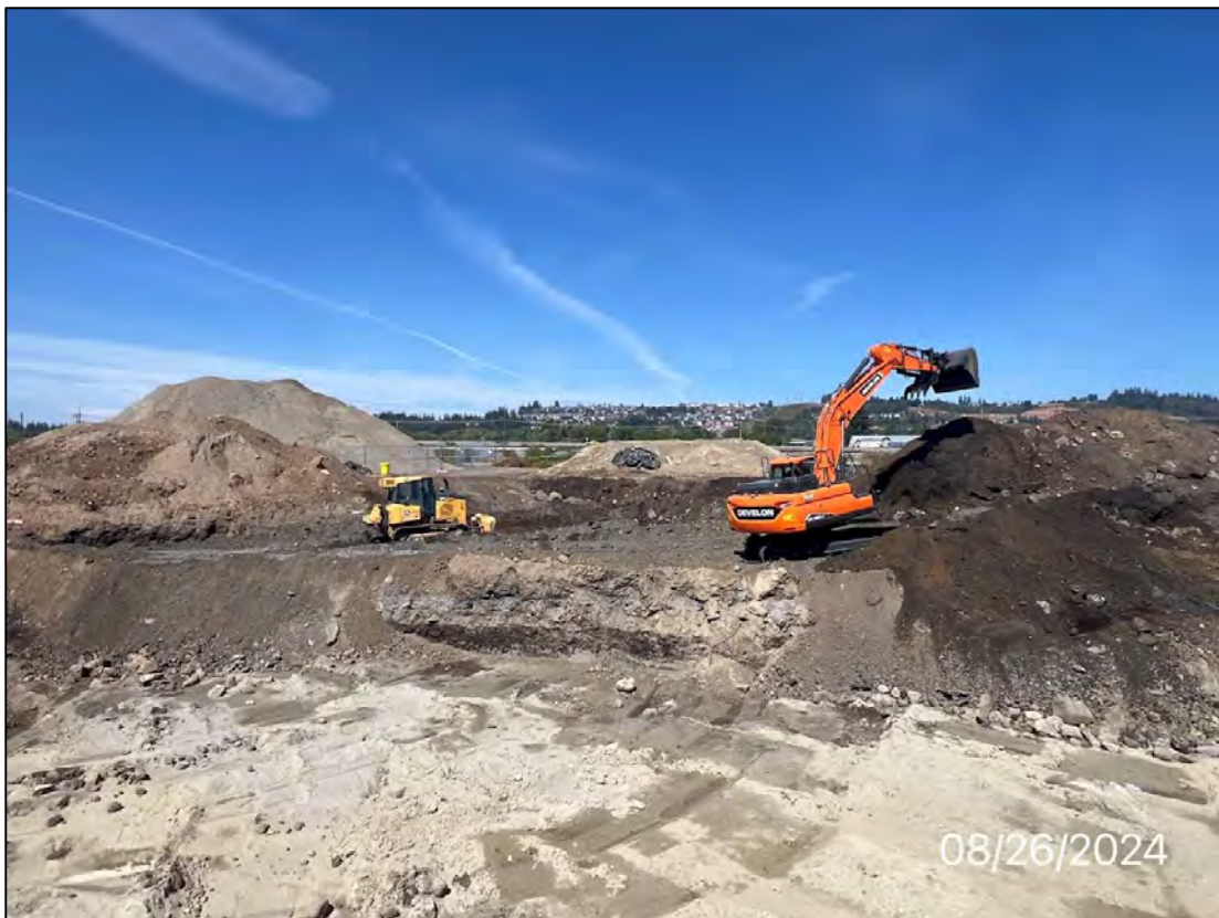
Photo 12: Excavation area along the southern portion of Building B, facing north, 8/26/24.
