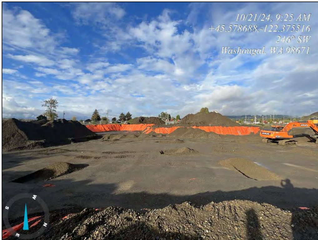
Photo 47: Pot holing in the northern portion of the excavation to retest the structural fill within the first two lifts, facing west, 10/21/24.
