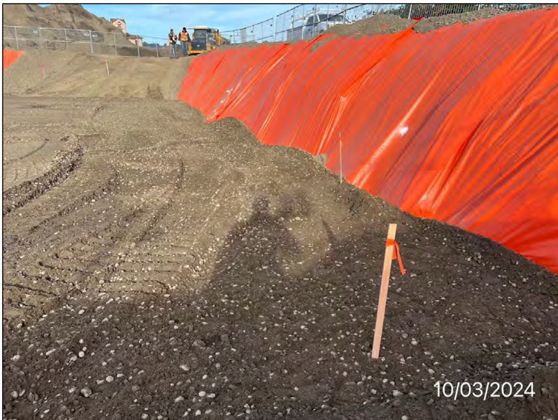
Photo 42: Survey stakes placed at edge of Building B show insufficient excavation boundaries to encompass the additional 15 foot zone of influence. White dot on demarcation fabric is Building B northeast corner, facing west, 10/3/24.
