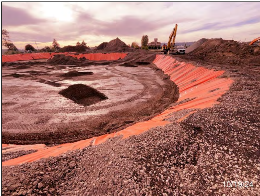
Photo 46: Pot holing within the northern portion of the excavation to retest the structural fill within the first two lifts. The third and fourth lifts were removed and stockpiled within the southern portion of the excavation, facing west, 10/19/24.
