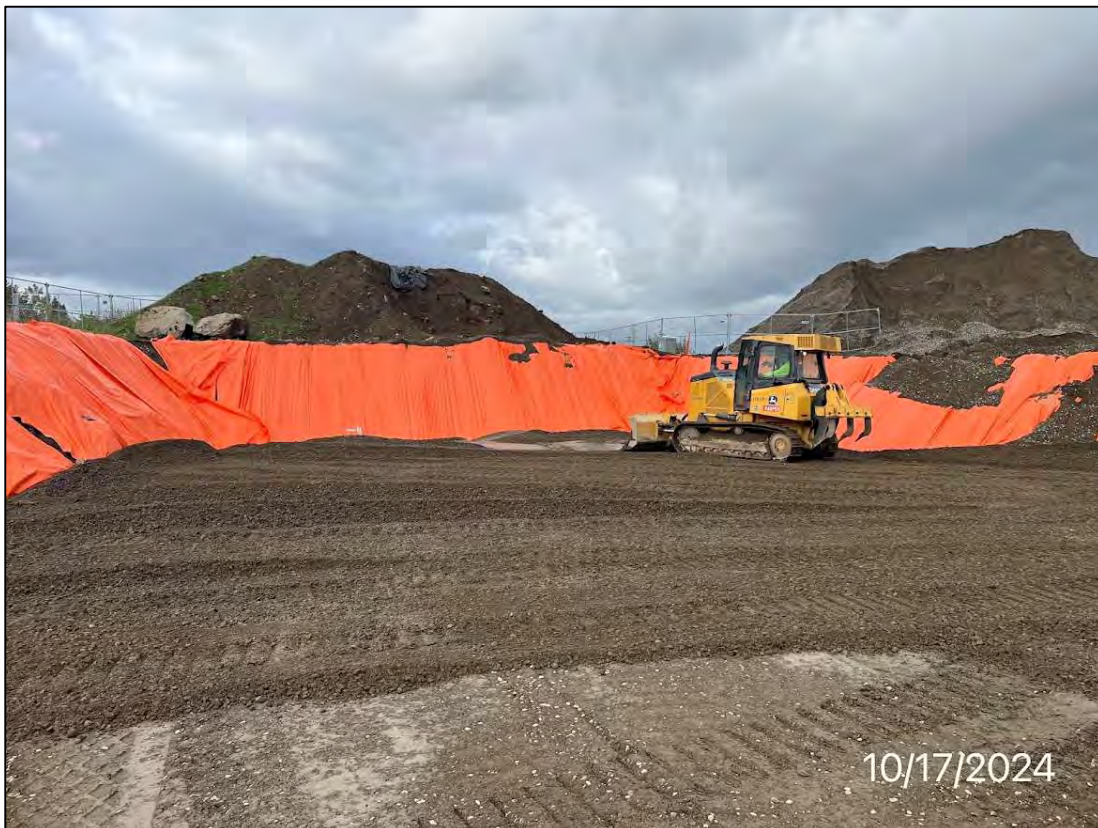
Photo 44: Swofford spreading structural fill in the southwest corner of the excavation, facing west, 10/17/24.
