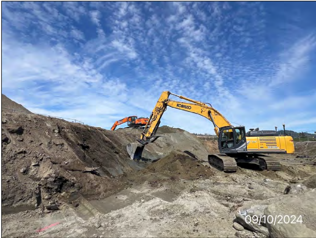
Photo 21: Excavating impacted soils from the west portion of Building B, facing north, 9/10/24.
