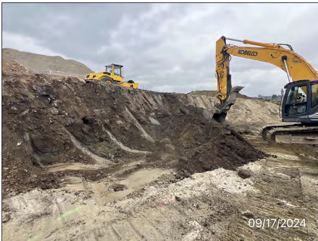
Photo 29: Excavating impacted soils from west excavation edge in the vicinity of Building A, facing east, 9/17/24.
