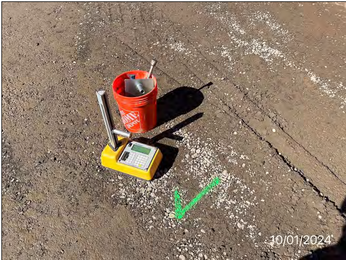
Photo 39: Compaction testing on first completed lift using nuclear density gauge, 10/1/24.
