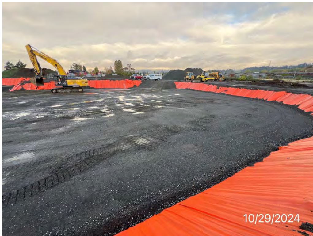
Photo 54: Continuous precipitation caused structural backfill to have a greater than optimal moisture content, backfill work was paused to wait for drier conditions, facing west, 10/29/24.
