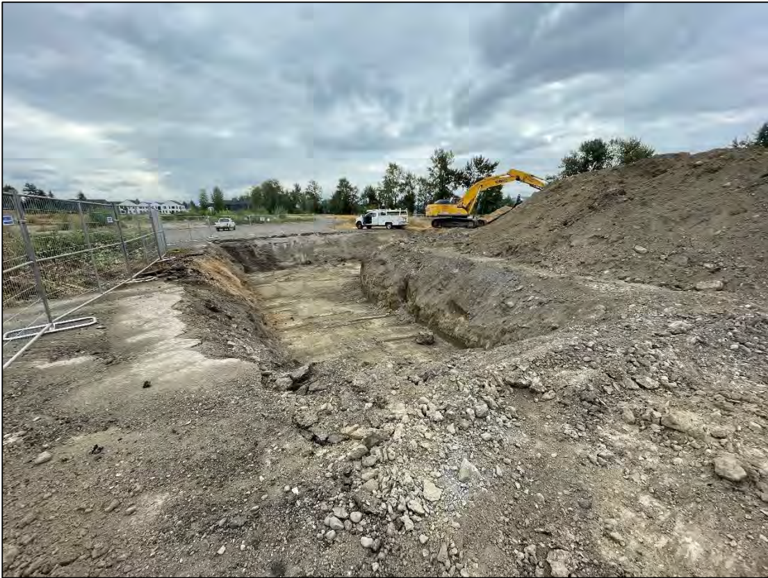
Photo 3: Excavation area along northern portion of Building B, facing east, 8/13/24.
