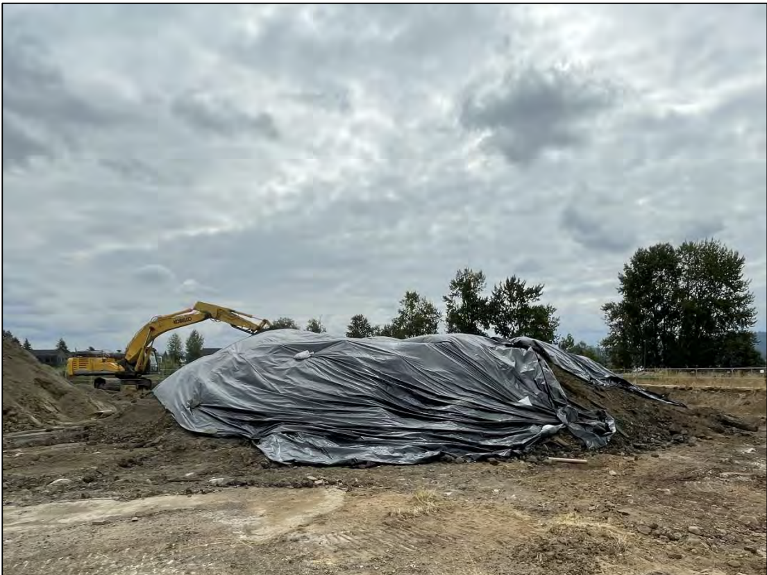
Photo 4: Stockpiled “organics” soil from the northern portion of the excavation, facing east, 8/13/24.
