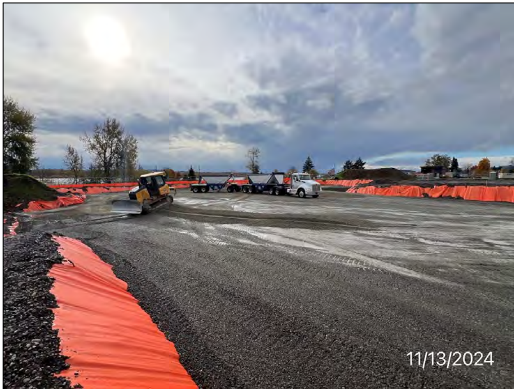
Photo 63: Loading structural backfill directly into the excavation, facing southwest, 11/13/24.
