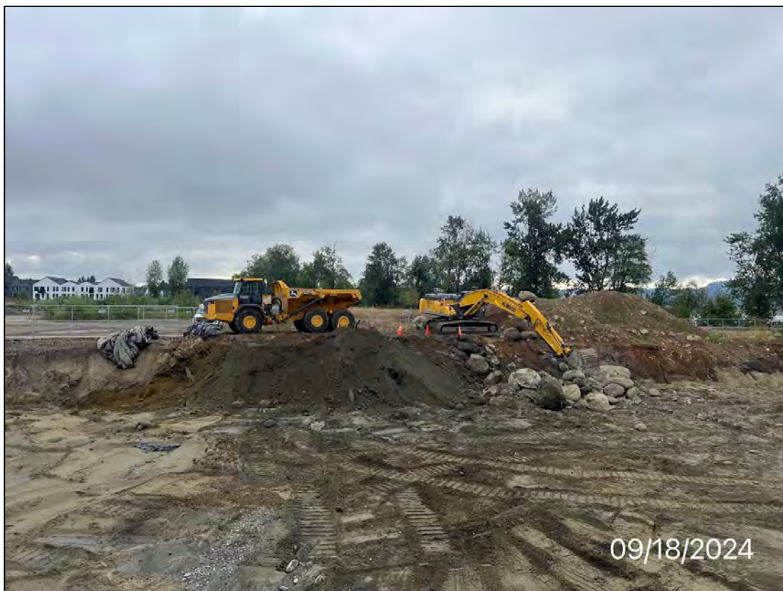
Photo 30: Loading boulders out of excavation, facing east, 9/18/24.
