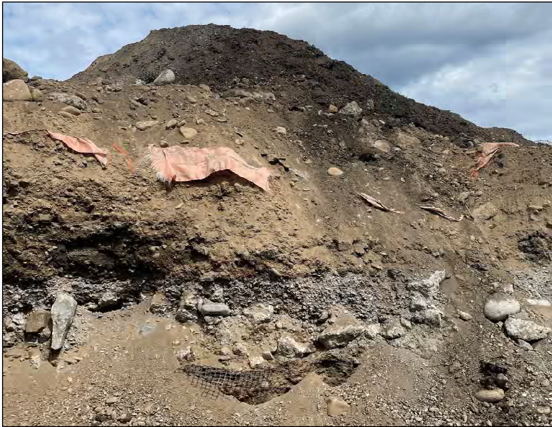
Photo 9: Subsurface materials exposed within excavation sidewall including, black geogrid (base) capped by crushed concrete and gravel-silt soils with orange demarcation fabric on top. Cap material can be seen exposed above the orange demarcation fabric, facing north, 8/16/24.
