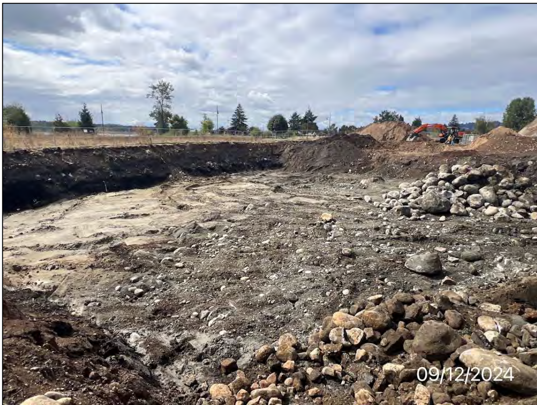
Photo 26: Excavation area, facing southwest, 9/12/24.
