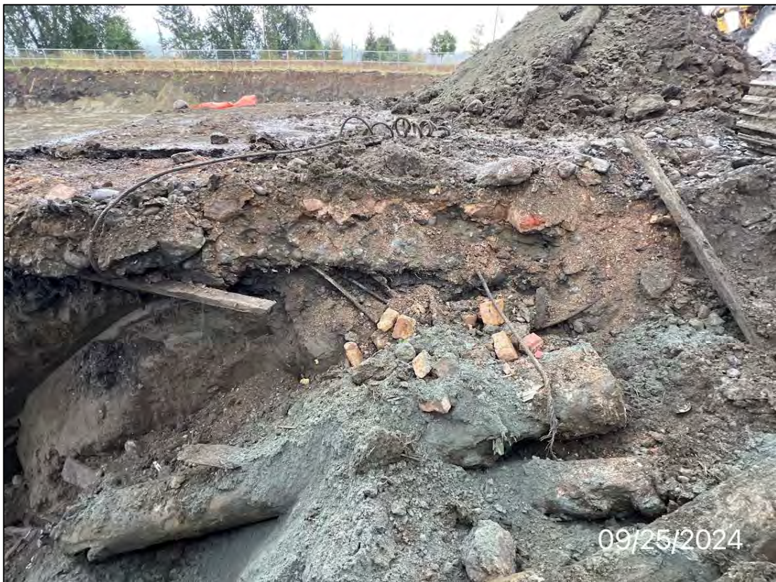
Photo 34: Timbers and fill debris in test trench dug along western edge of excavation in the vicinity of Building a, facing south, 9/18/24.
