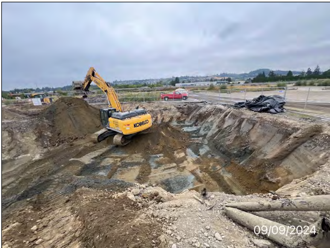
Photo 20: Excavating "organic" soils from the northern portion of Building B, facing west, 9/9/24.
