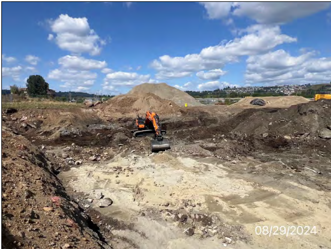
Photo 16: Excavation area in the vicinity of the southwest corner of Building B and roadway area, facing west, 8/29/24.
