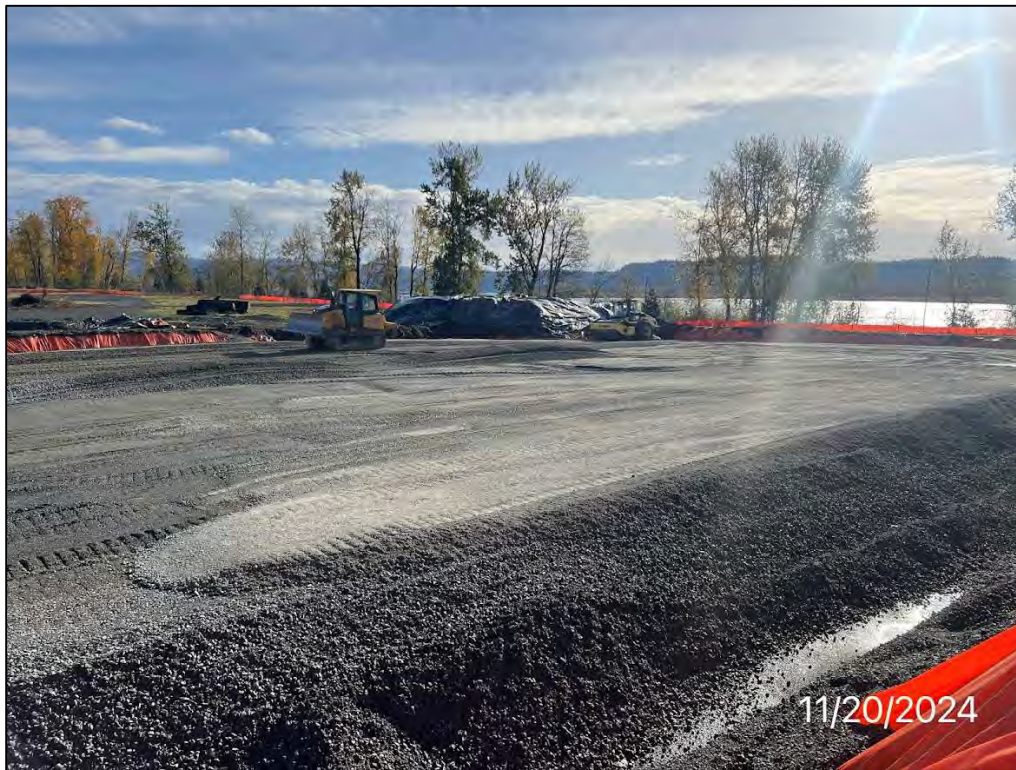
Photo 66: Conditions within the northern portion of the excavation on this date, facing southeast, 11/20/24.
