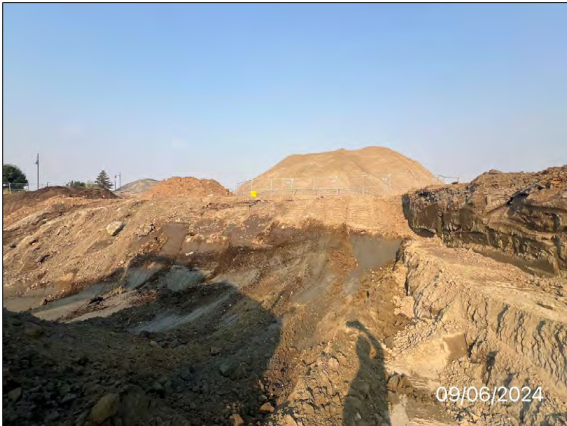
Photo 19: Excavation area in the vicinity of Building B, facing west, 9/6/24.
