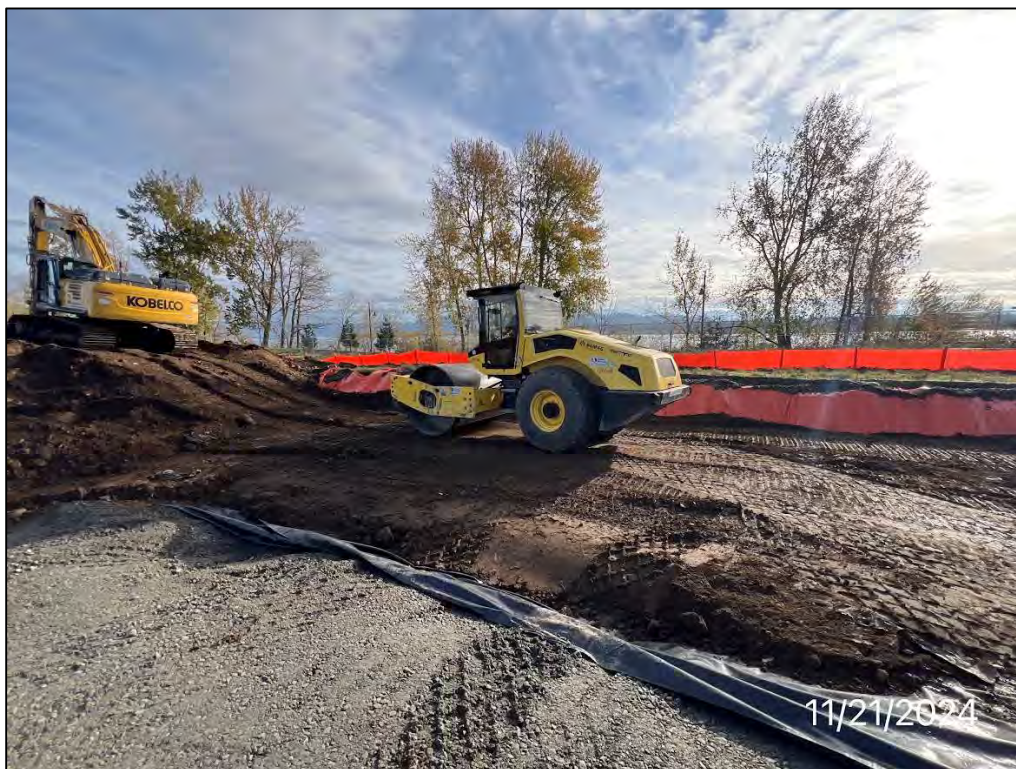
Photo 67: Swofford attempting to place and compact the cap material within the roadway in the southern portion of the excavation. Compaction of 95% was not able to be achieved and cap material was subsequently removed, facing south, 11/21/24.
