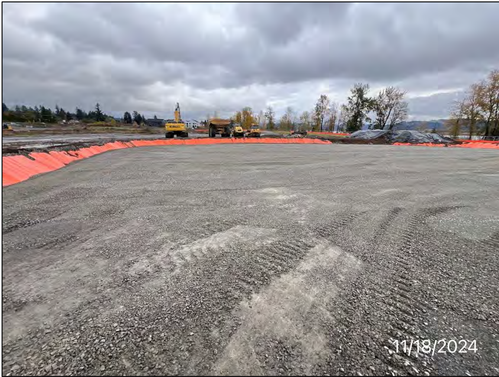
Photo 65: Conditions within the excavation on this date, facing southeast, 11/18/24.
