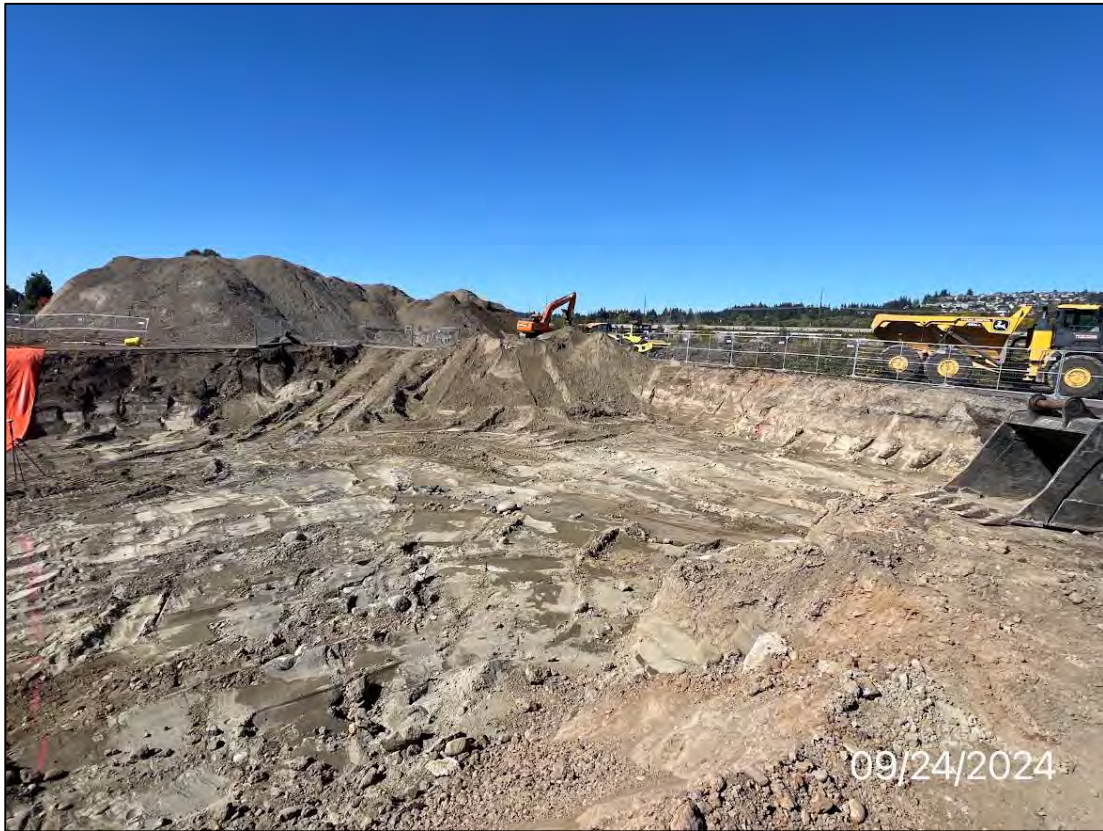
Photo 33: Excavation area in the vicinity of Building B, facing west, 9/24/24.
