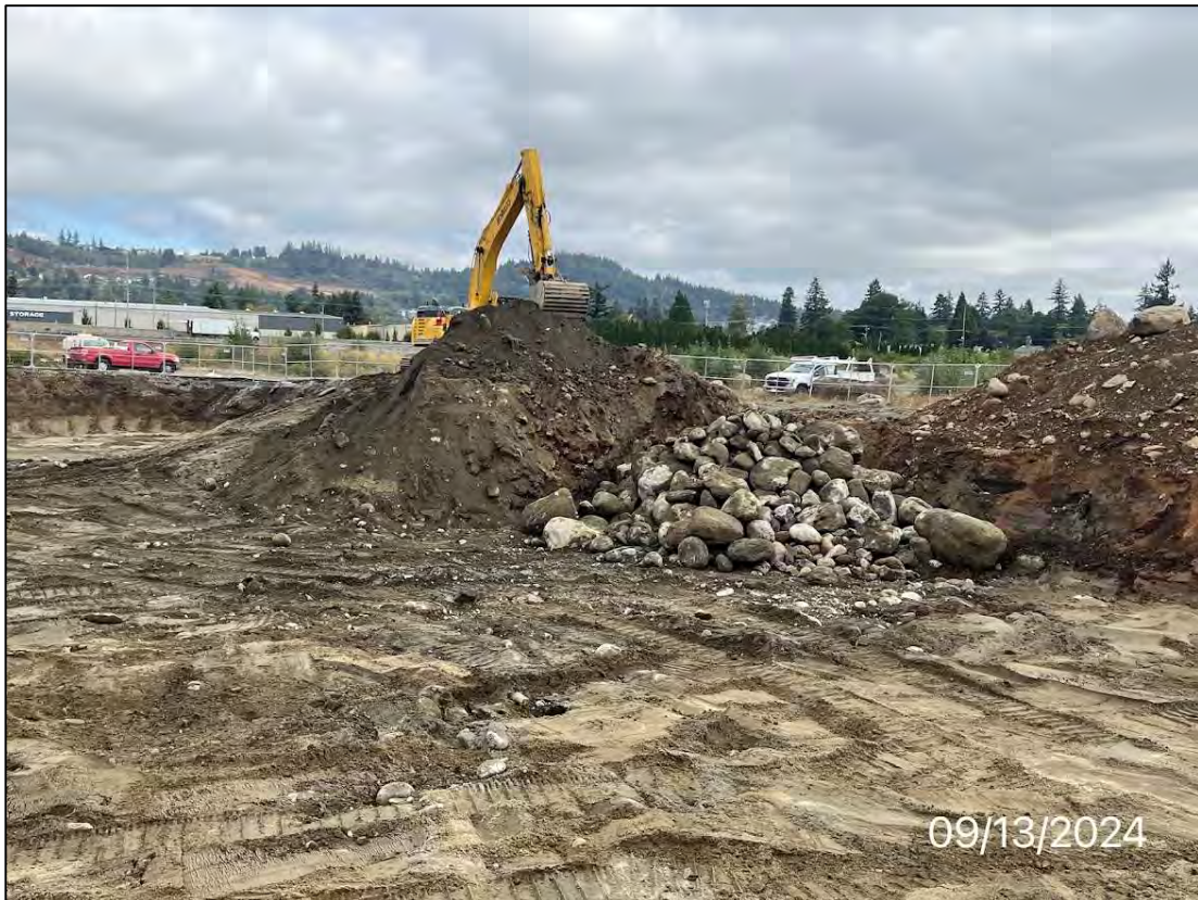
Photo 27: Impacted soil and boulders staged for loading out, facing north, 9/13/24.
