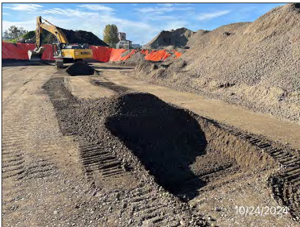
Photo 50: Pot holing within the southern portion of the excavation to retest the first and second lifts, facing west, 10/24/24.
