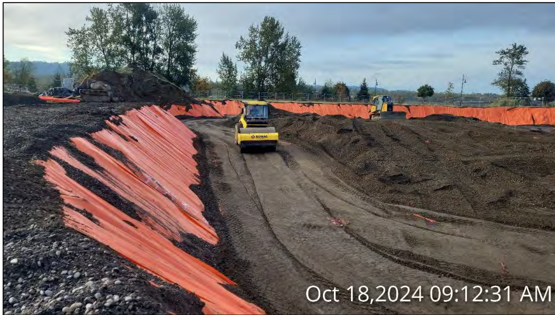
Photo 45: Swofford compacting structural fill in the extended portion along the northeastern part of the excavation, facing south, 10/18/24.
