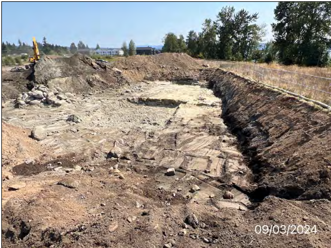
Photo 17: Excavation area in the vicinity of the roadway area, facing east, 9/3/24.
