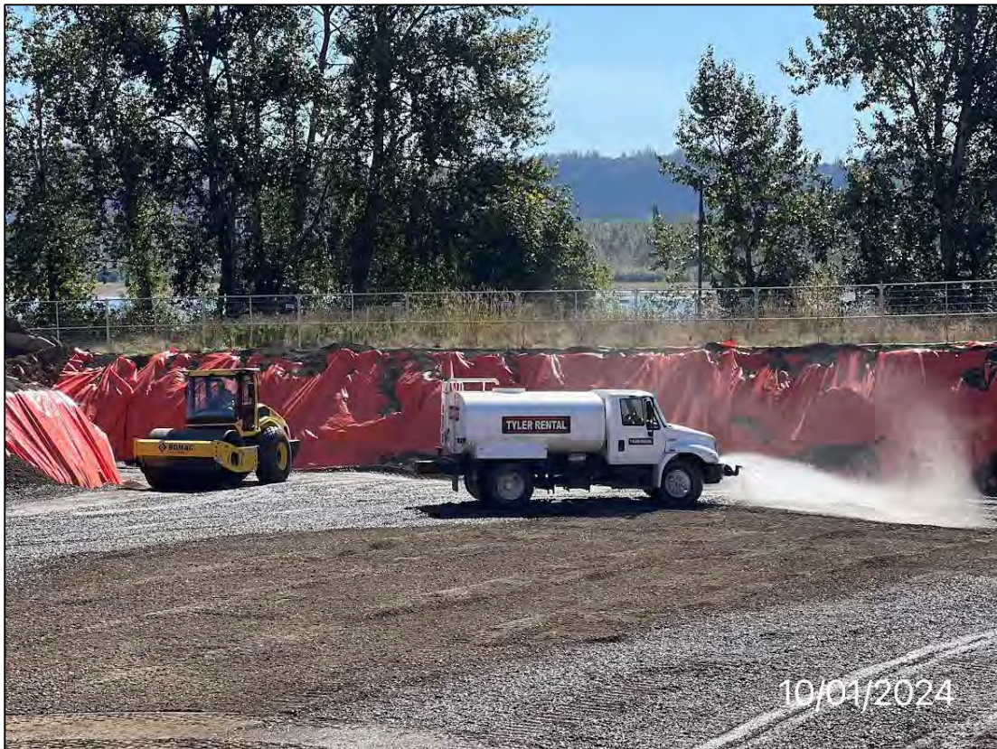
Photo 38: Moisture conditioning and compaction of the first lift. This lift was placed in two separate thin lifts in order to compact the underlying subgrade. Once the subgrade was observed to be compacted to an unyielding state, the second thin lift was placed, moisture conditioned and compacted, facing southeast, 10/1/24.
