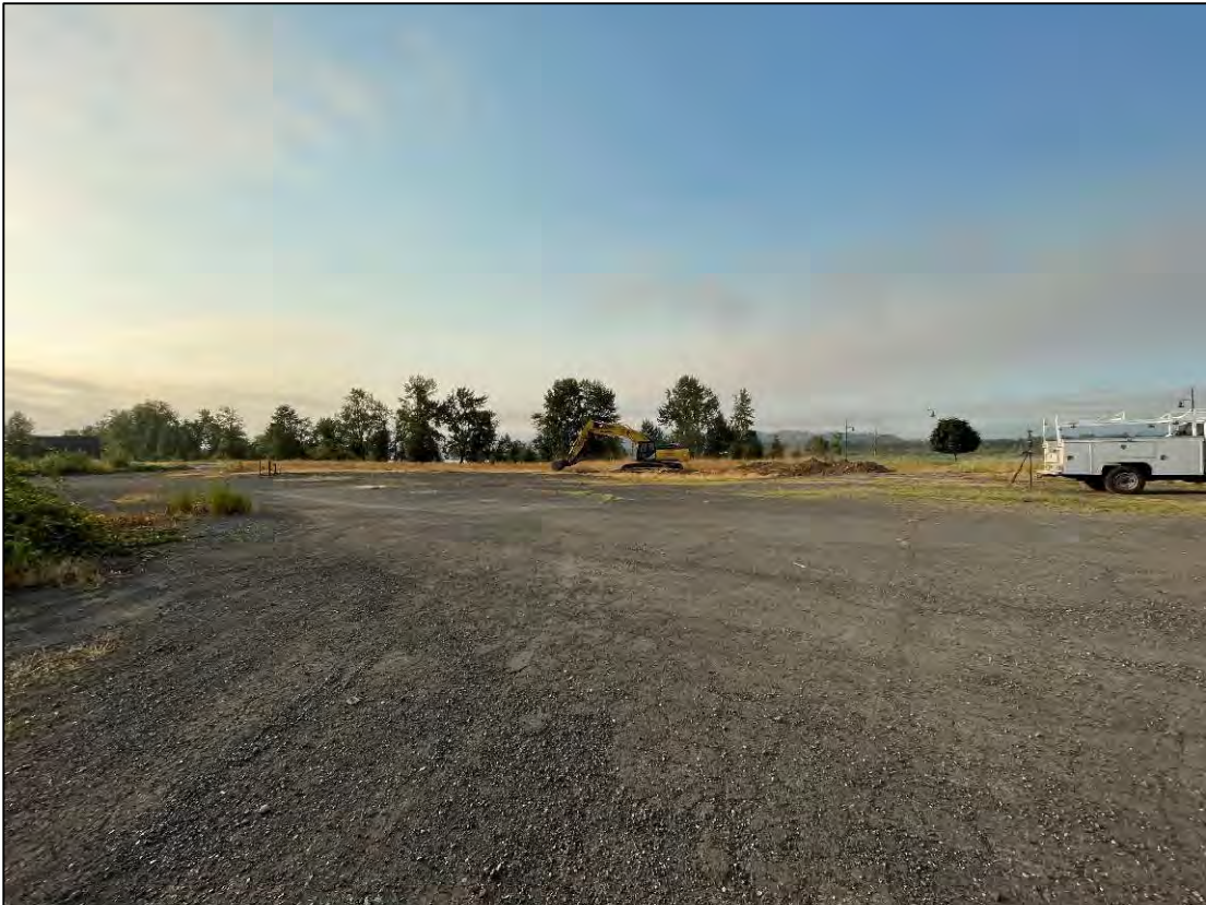
Photo 1: Site conditions upon start of project, facing south, 8/7/24
