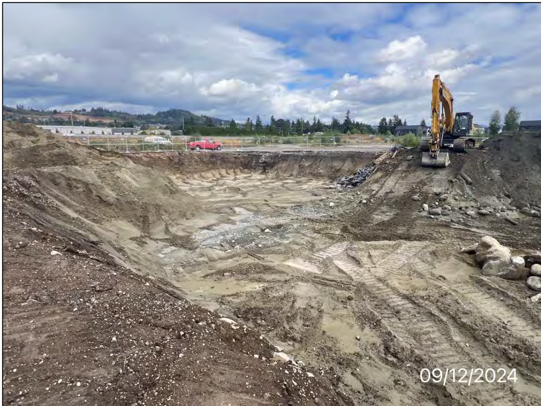
Photo 25: Excavation area, facing northeast, 9/12/24.
