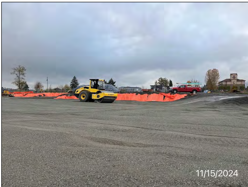
Photo 64: Compacting structural backfill in the northern portion of the excavation, facing west, 11/15/24.
