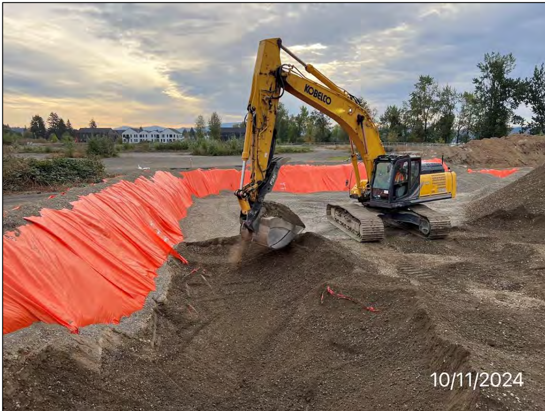
Photo 43: Swofford removing structural fill in order to extend the excavation north, facing east, 10/11/24.
