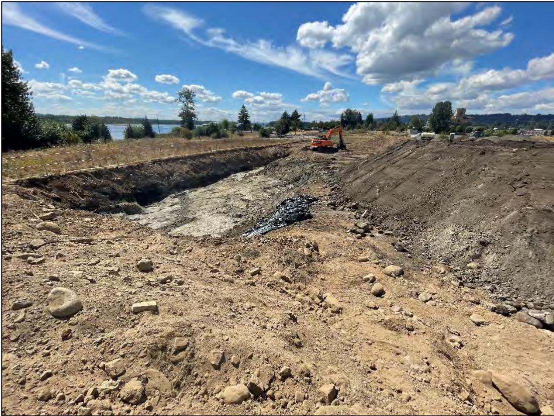
Photo 7: Excavation area along the proposed roadway area south of Building B, facing east, 8/16/24.
