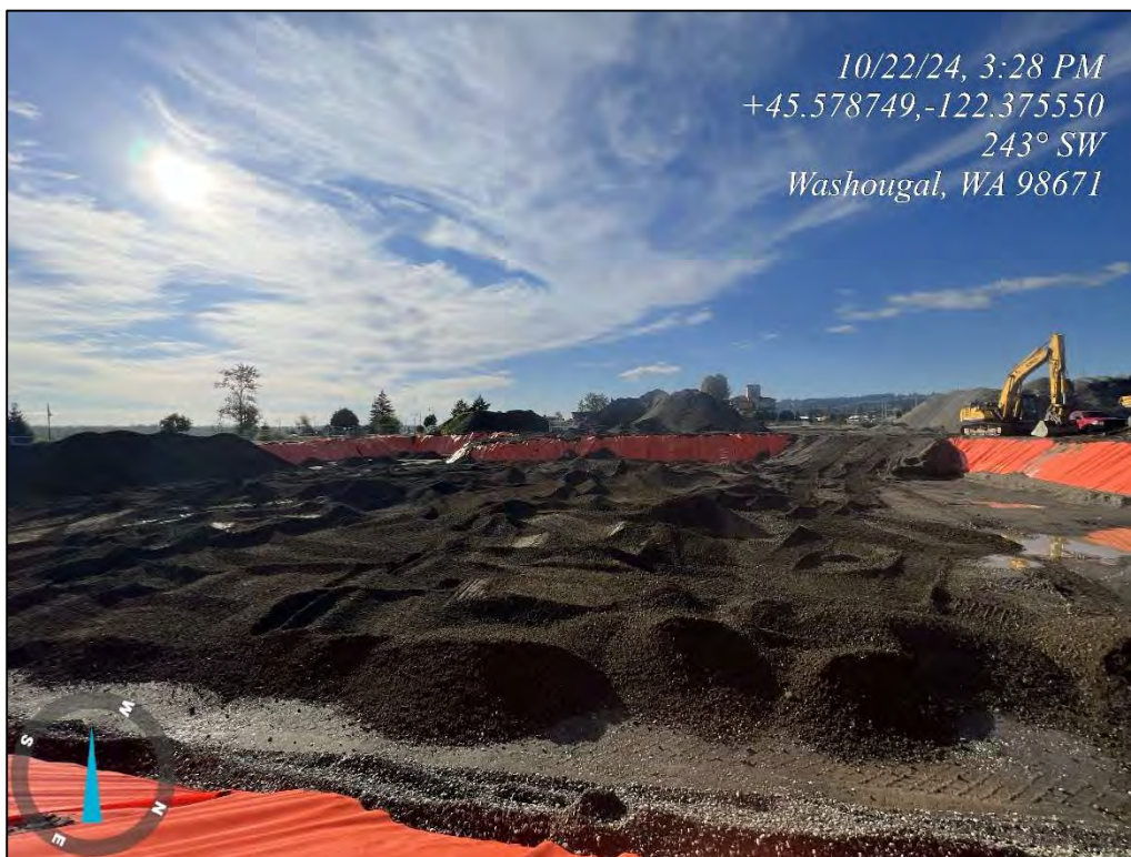
Photo 48: Replacing the third and fourth lifts within the northern portion of the excavation after retesting the first and second lifts, facing west, 10/22/24.
