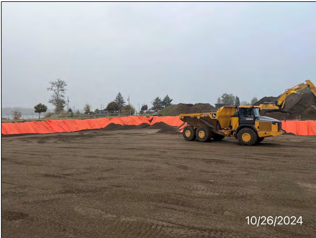
Photo 52: Loading structural backfill within the southwestern corner of the excavation, facing southwest, 10/26/24.
