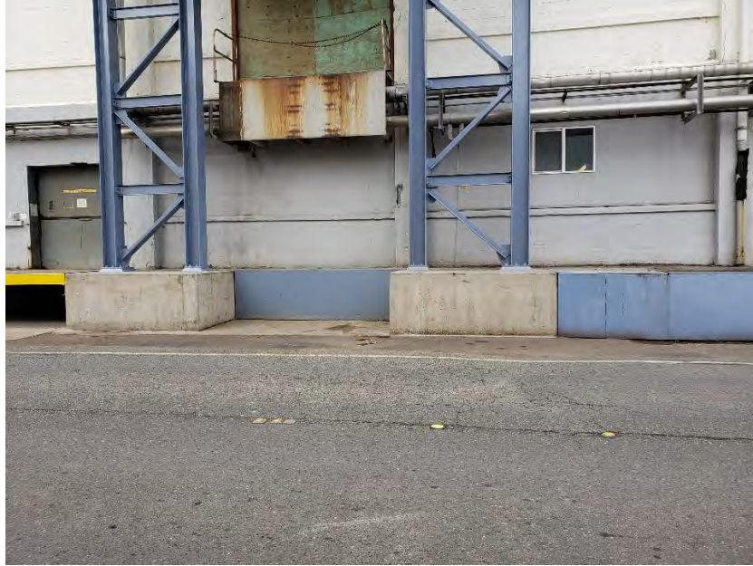
PHOTO 3 – AREA AFTER FOUNDATION WORK COMPLETED & NEW BRIDGE INSTALLED
