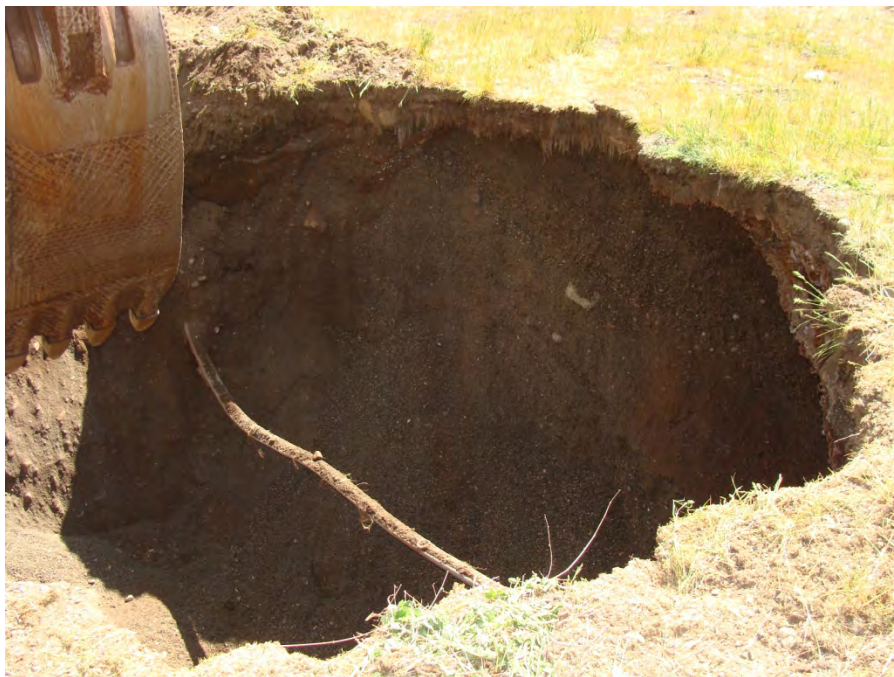
Test Pit 4 – Metal piping and layered debris observed during excavation (<5% debris).
