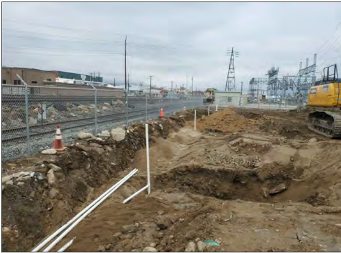
PHOTO 1 Backfilling.
