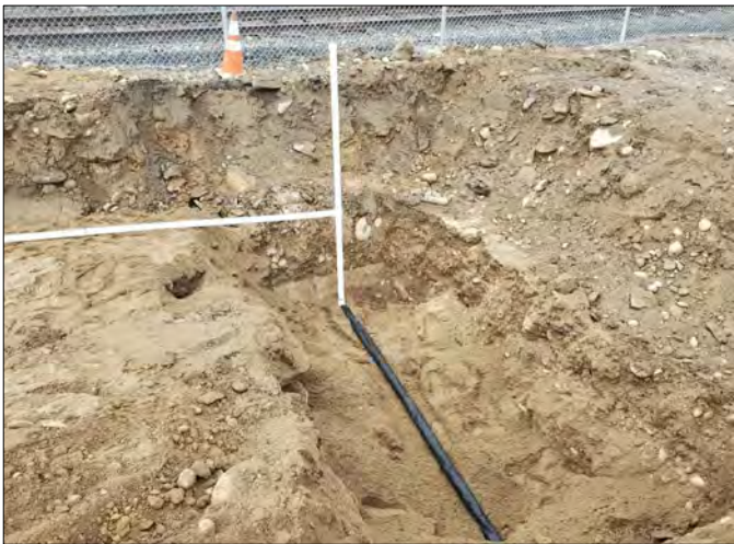
PHOTO 2 Conveyance piping installation.
