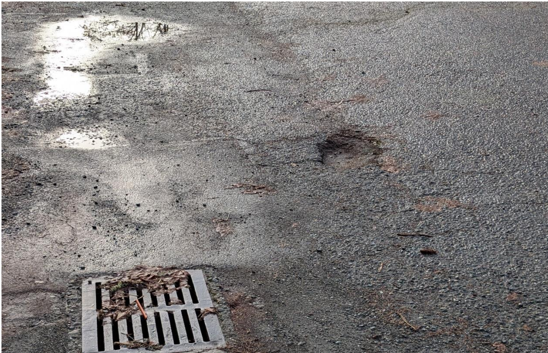
Photo Location 1. 12/23/2024 site inspection, pothole in photo above.
