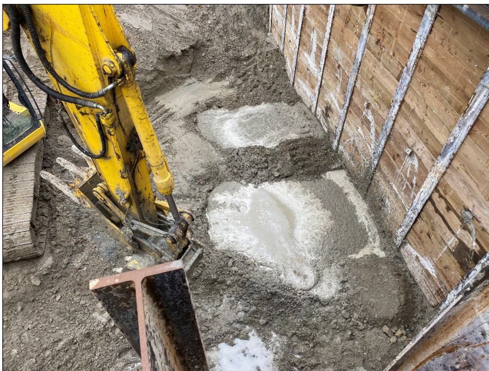
2. Slot trenches adjacent to Piles 6 and 8 filled with CDF.
