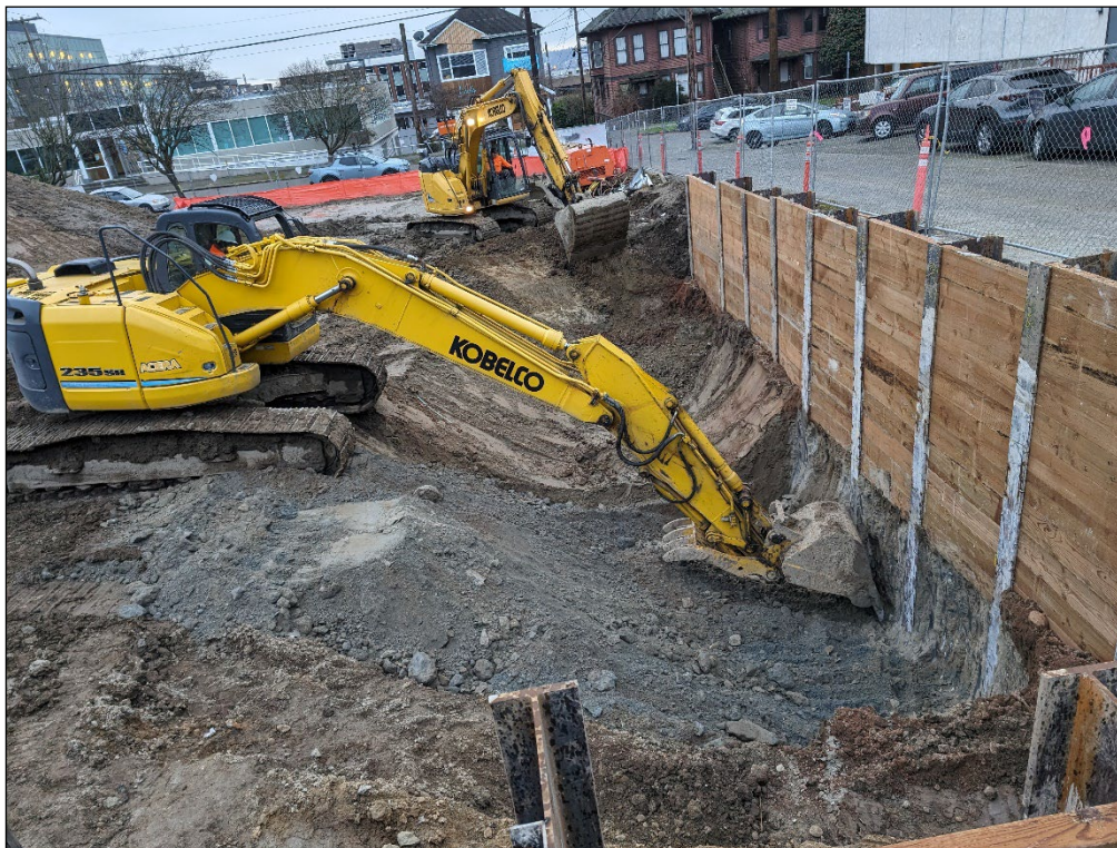
1. Excavation and lagging along western property boundary (looking south).
