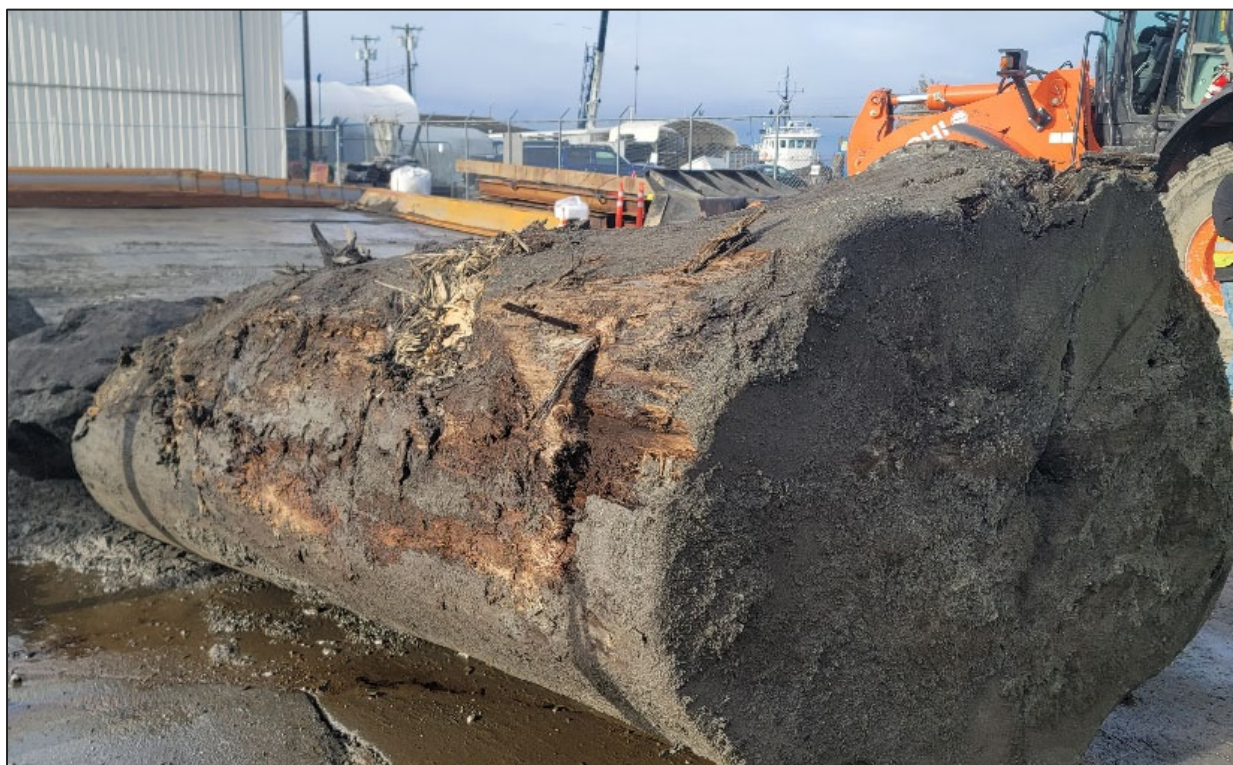
Photograph 18 Wood Debris Removed from Excavation
