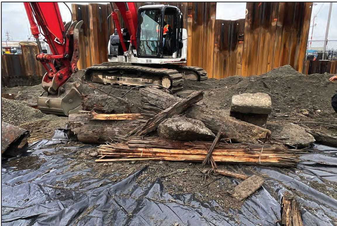
Photo 10. Large wood and concrete debris encountered at the north end of Phase-4 soil removal, view to the west.
