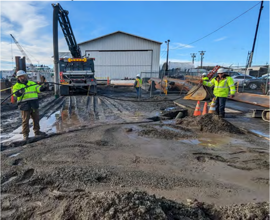
Exposure of ESR Water Line
