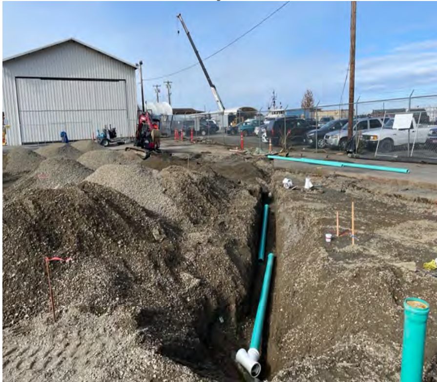
ESR Office Sanitary Sewer Line Install
