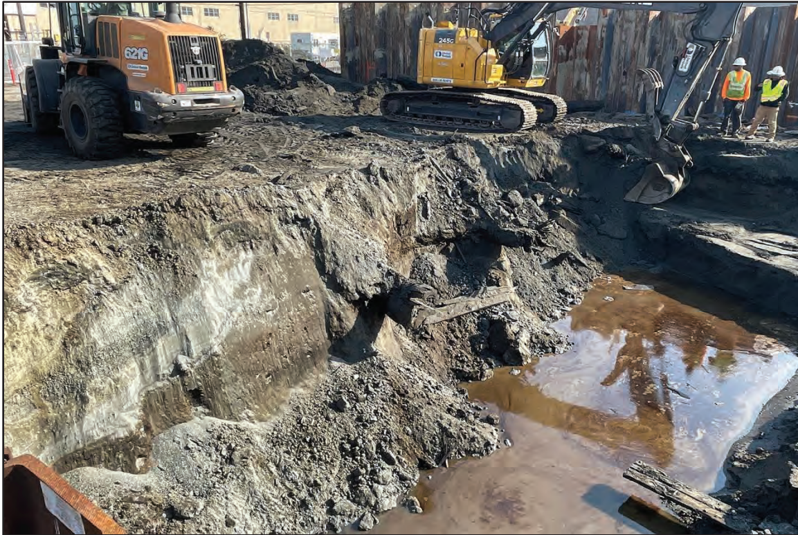
Photo 5. Phase-1 soil removal showing in-situ wood debris, view to the northeast. Note petroleum contamination of the flooded area.
