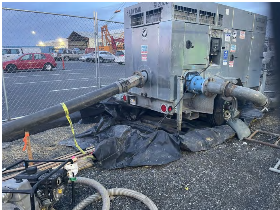
Photo 2. Pump located on southeast corner of site with repaired secondary containment system.
