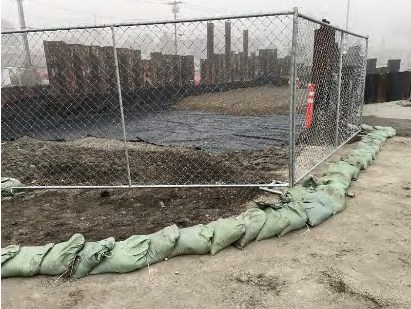
Photo 1. Newly installed onsite water/sediment flow path.
