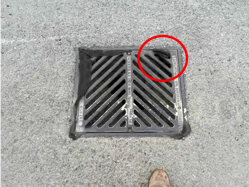
Photo 1. Catch basin with tear in Witches Hat
