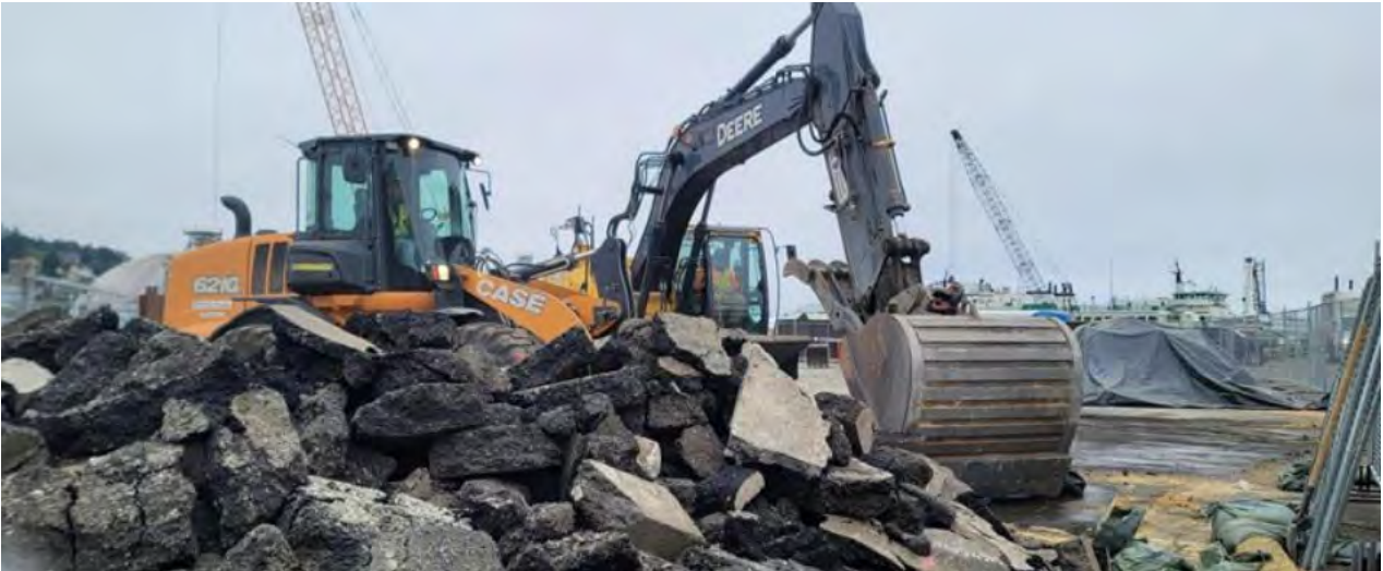
Asphalt Break Out and Export – 09/30/22
