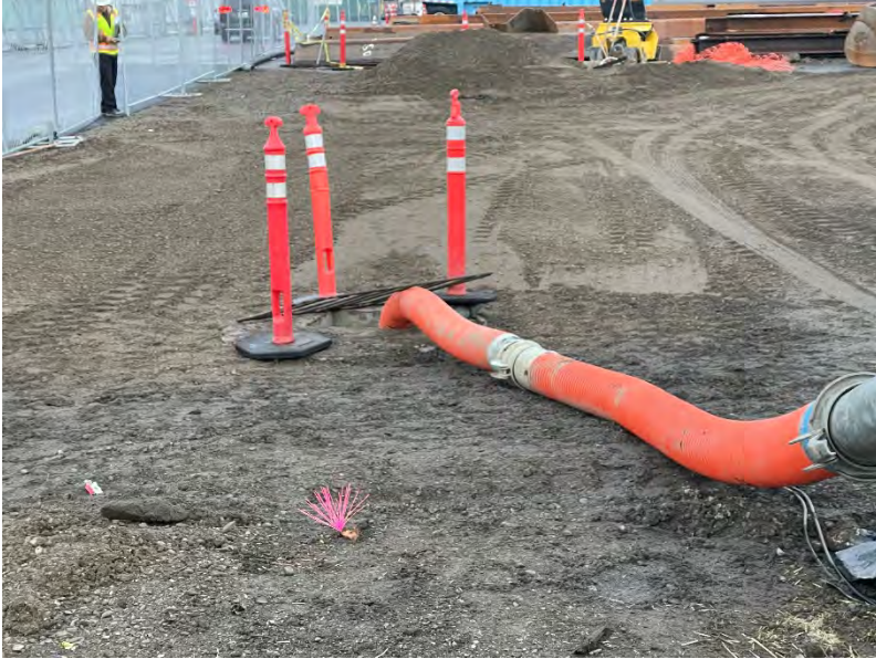
Photo 1. New permanent catch basin in need of insert
