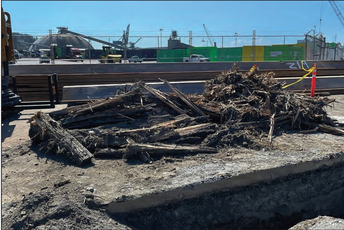
Photo 3. Typical large wood debris removed during exploratory trenching for Phase-1 and 2. Port of Everett facilities background, view to the south.
