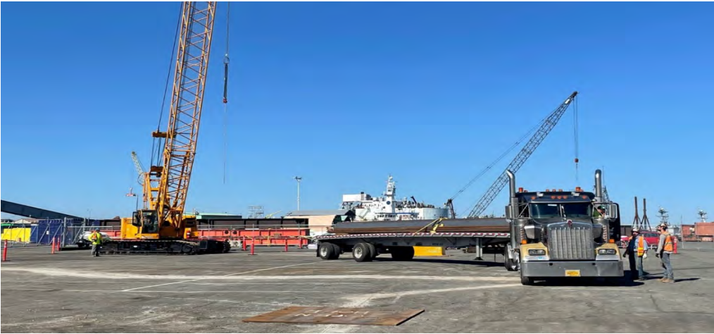
Sheet Pile Delivery
