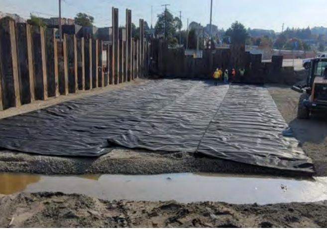
Aggregate Backfill and Liner
