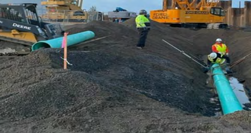
15-Inch Storm Line Installation
