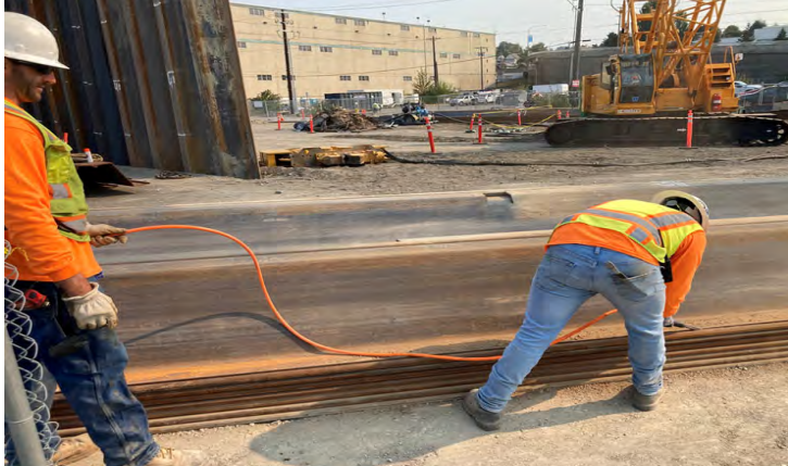
Sheet Pile Cleaning/Preparation
