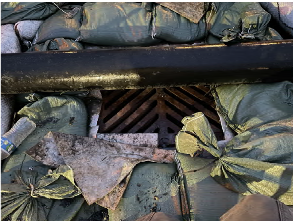
Photo 2. Functioning and protected onsite catch basin
