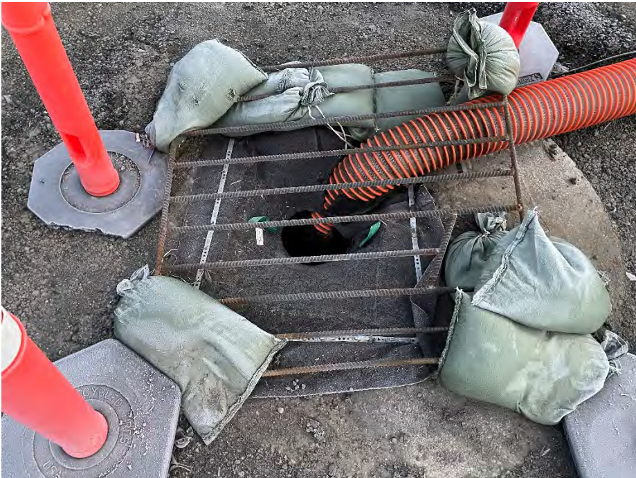
Photo 2. Functioning diversion pump to storm system
