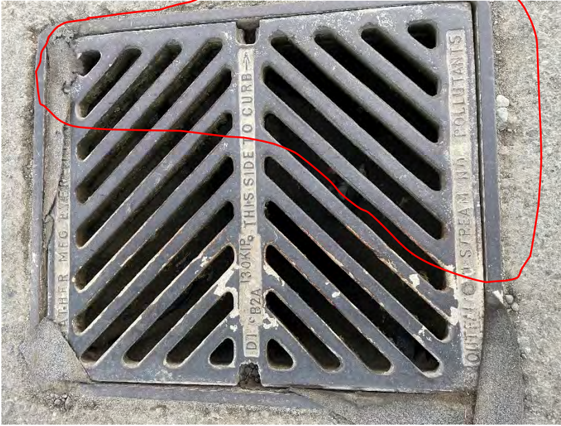
Photo 1. Catch basin Witches Hat with fallen corner circled in red
