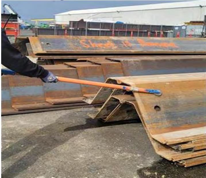
Use of Magnetic Rod to Direct Sheets
