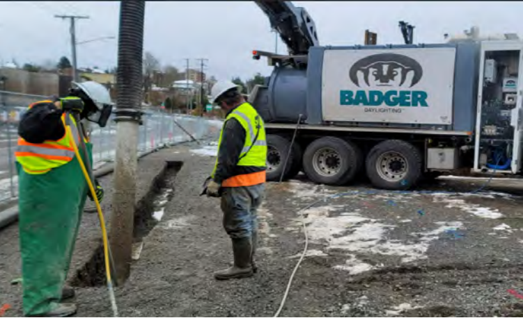
Stormwater Bypass Trench
