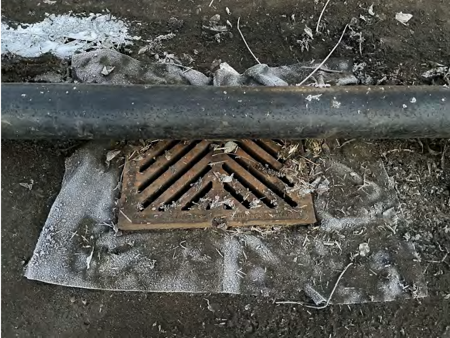
Photo 1. Functioning onsite catch basin
