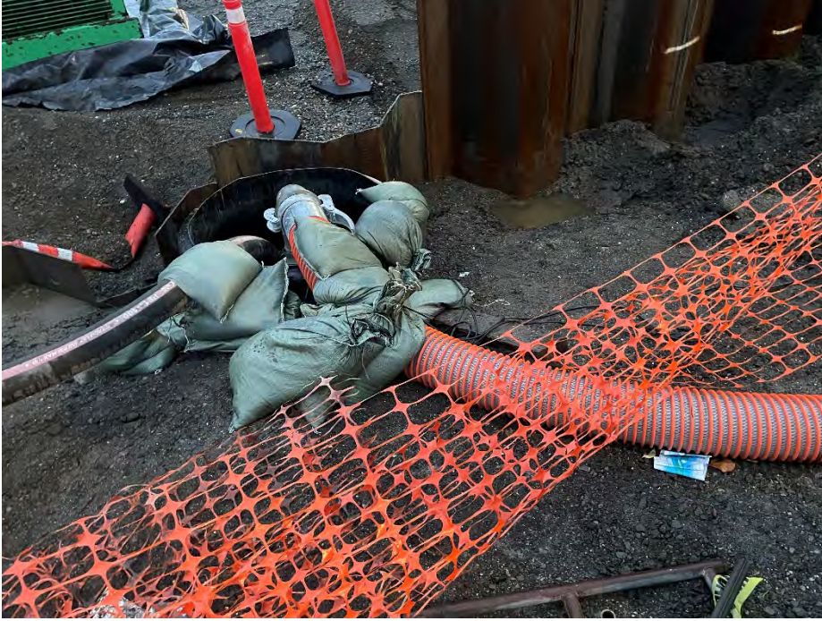
Photo 1. Federal Avenue sump with new 6" pipe
