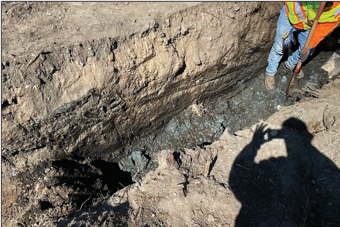
Photo 2. Typical undifferentiated stratigraphy for Phase-1 and 2 along the east side of Phase-1.
