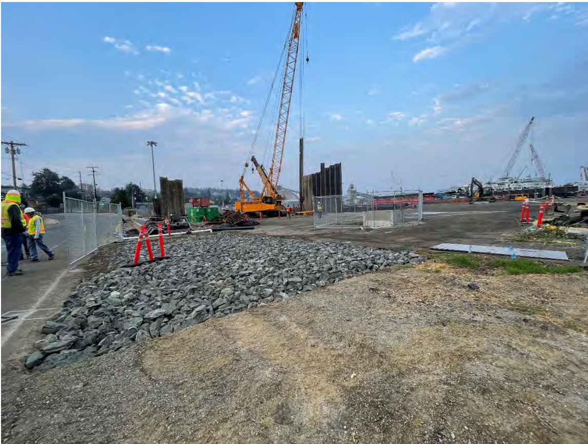
Photo 2. Newly installed construction entrance
