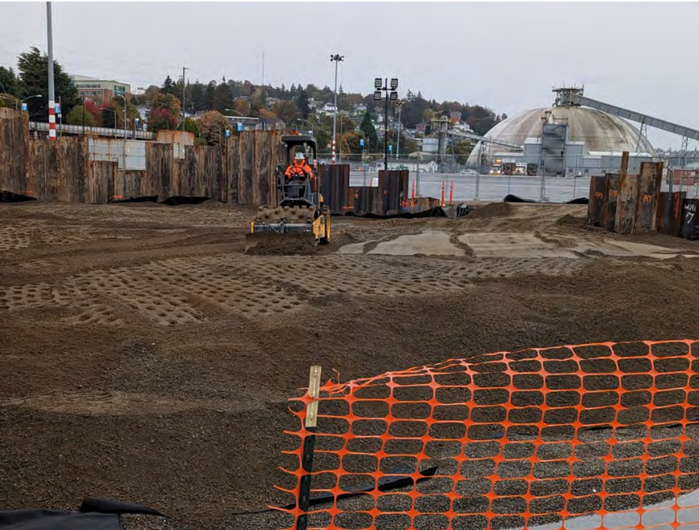
Fill compaction completed prior to asphalt base – 10/21/22
