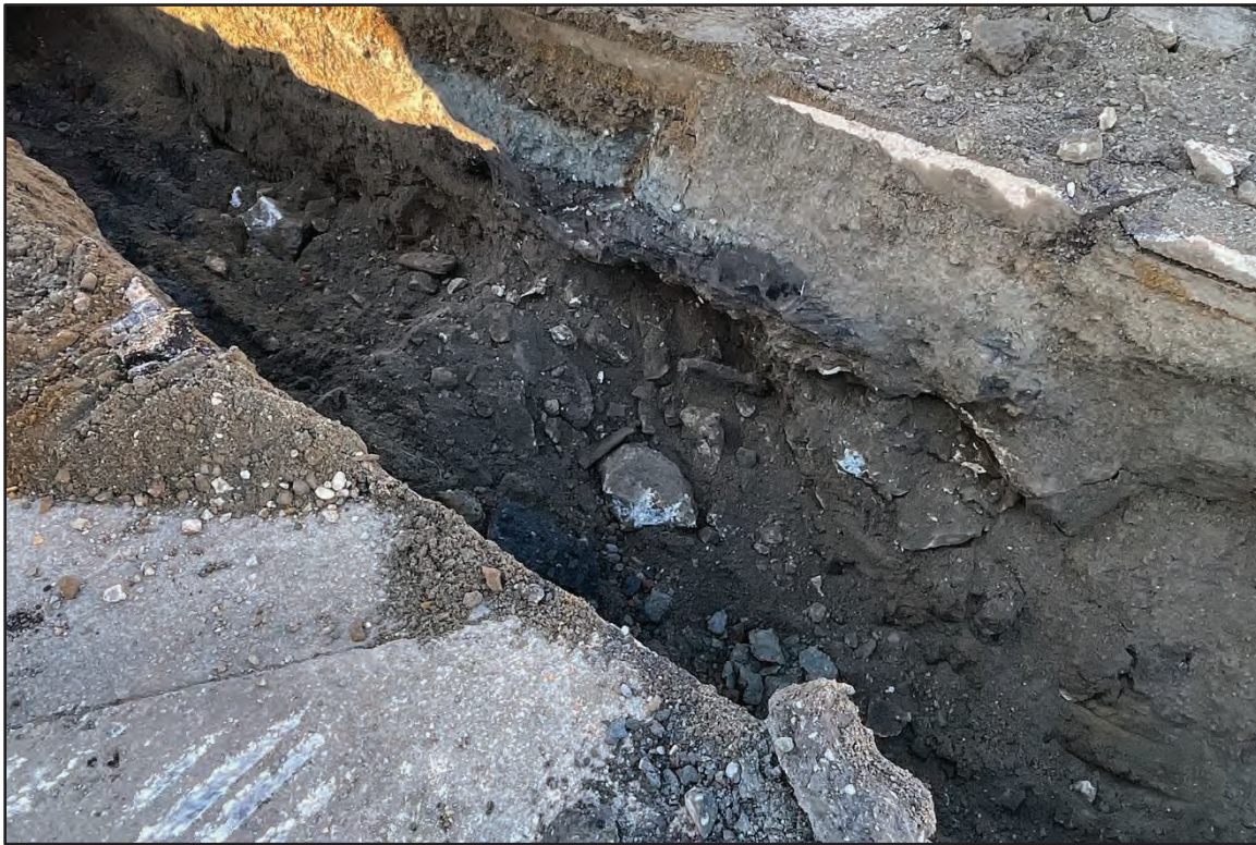
Photo 7. Phase-2 Trenching along the west side showing upper fill incidences and broken concrete.
