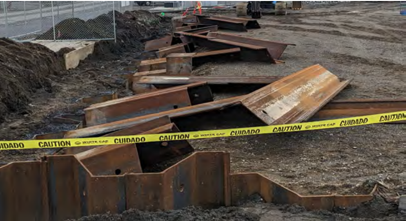
Barrier Wall Sheet Piles Cut to Grade
