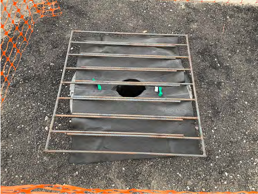
Photo 1. Newly installed onsite catch basin.
