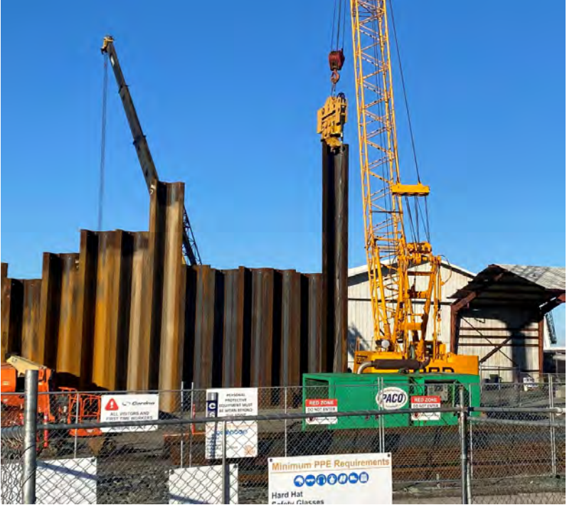
Phase 3 Shoring Install (New Sheets Right)
