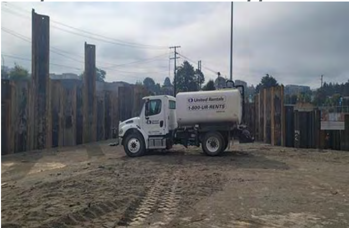
Asphalt Removal Dust Suppression
