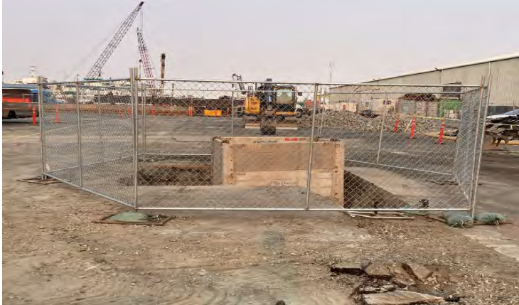
Storm Bypass Installation Trench Box
