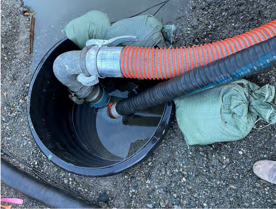
Photo 1. Federal Avenue functioning sump
