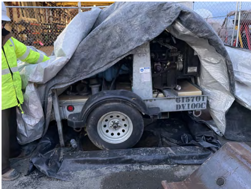
Photo 1. Pump located on northwest corner of site with newly installed secondary containment system.
