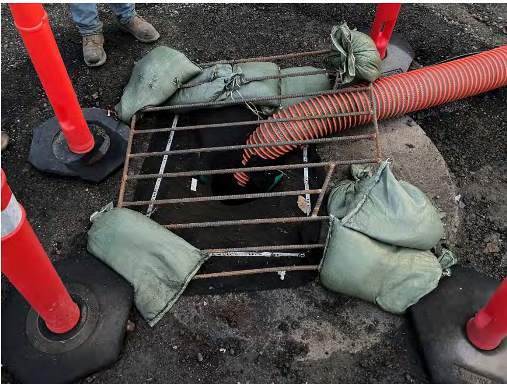
Photo 2. Functioning diversion pump to storm system
