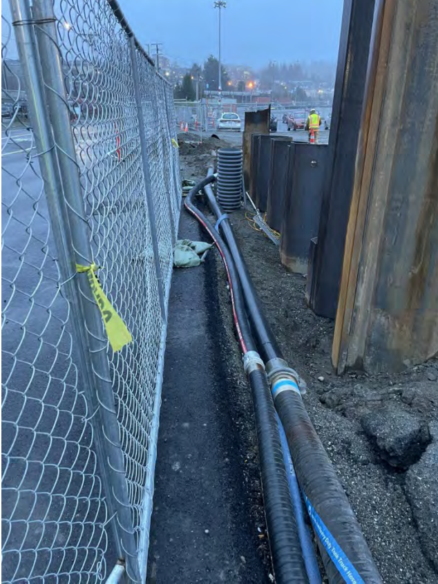
Photo 1. Diversion line to sewer system.
