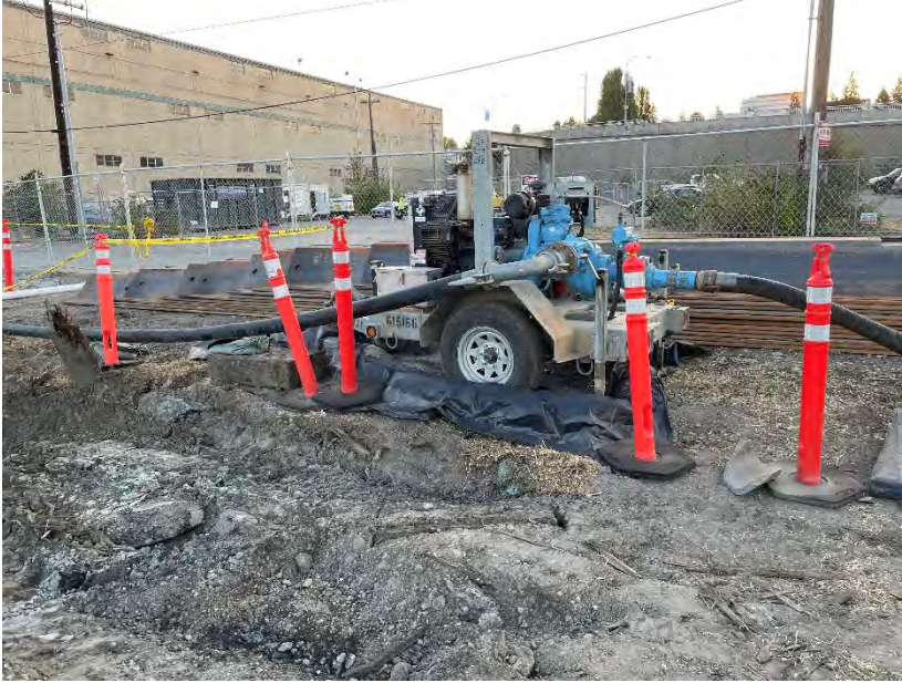
Photo 1. Pump with secondary containment
