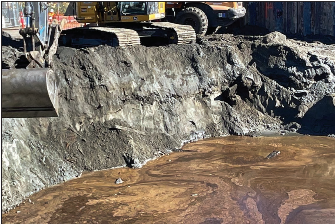
Photo 6. Phase-2 soil removal showing thin debris layer, view to the northeast. Note petroleum contamination of the flooded area.
