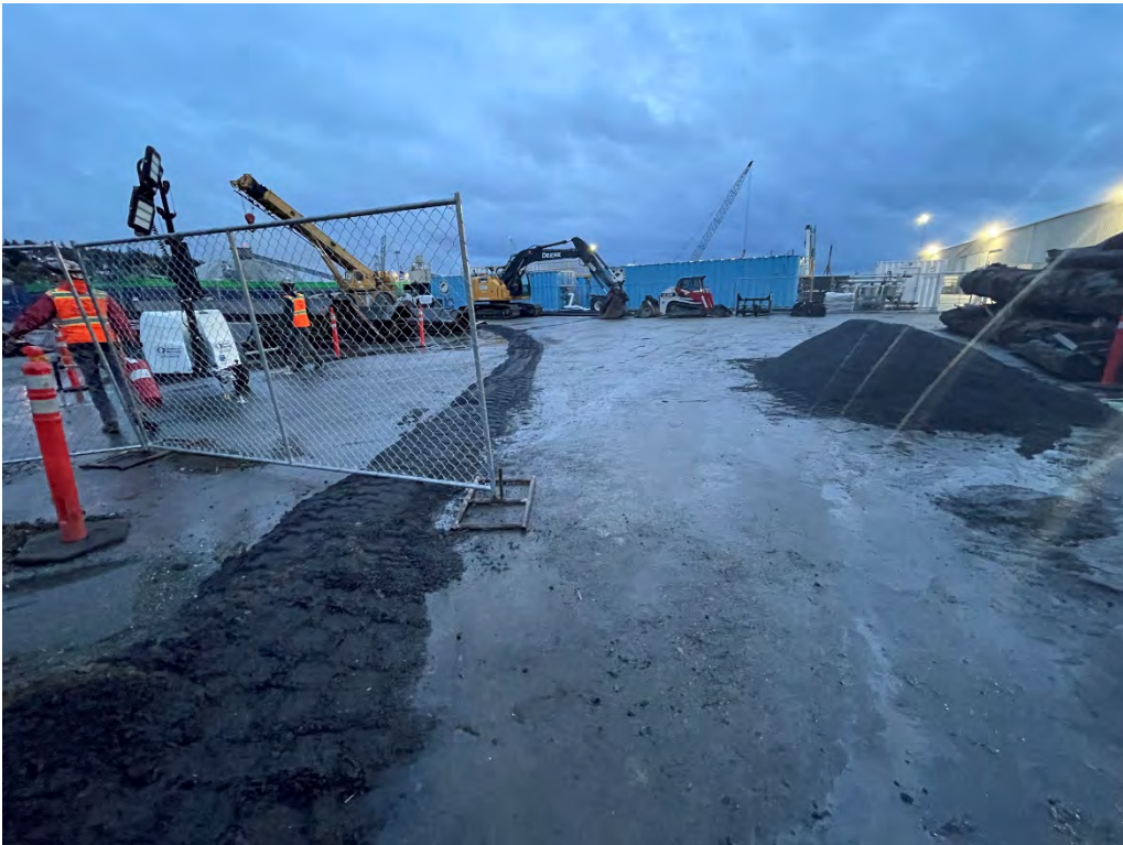
Photo 2. Newly constructed berm leading to onsite catch basin
