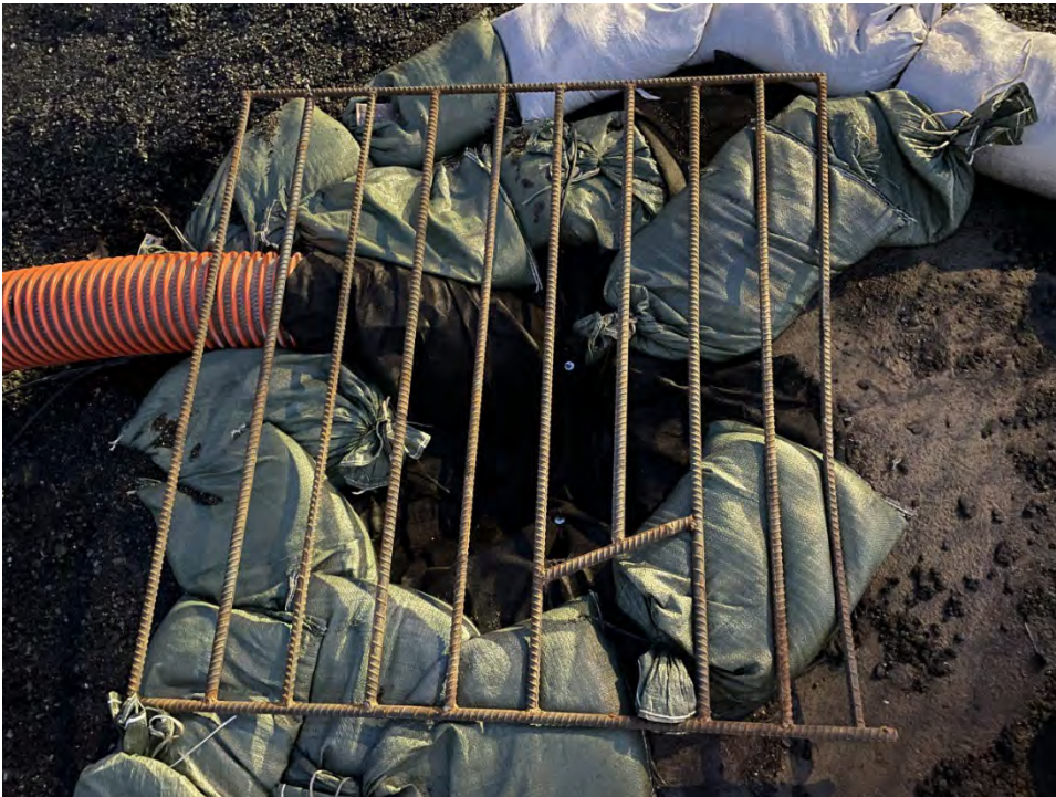
Photo 2. Functioning and protected onsite catch basin with diversion pump to septic
