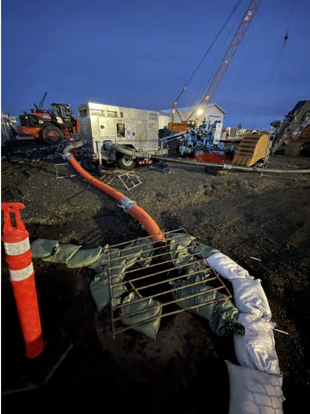
Photo 1. New diversion directed to septic system
