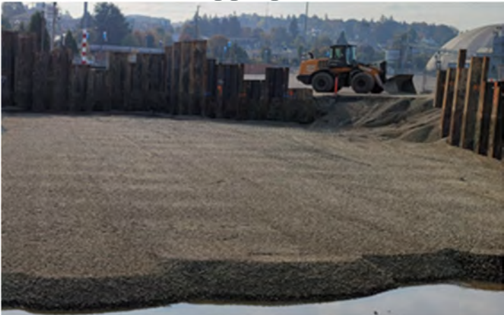
Phase 4 Aggregate Backfill
