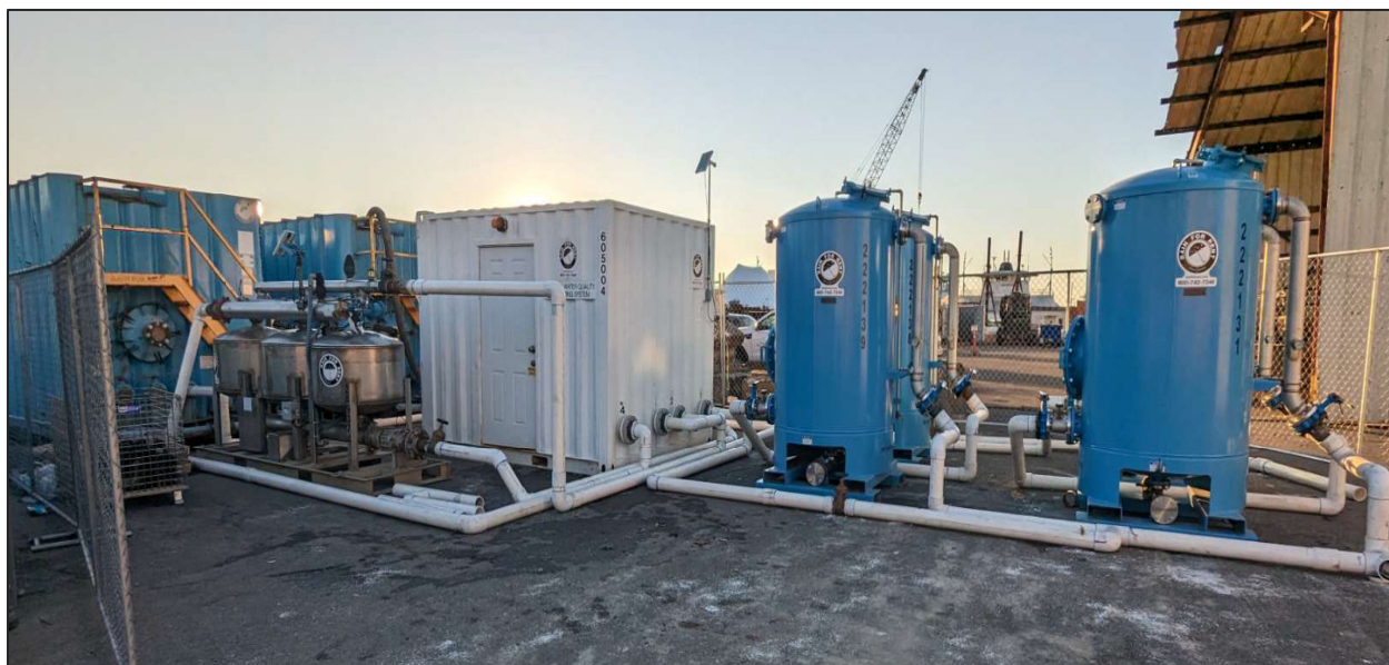
Photograph 1 Dewatering System Setup
