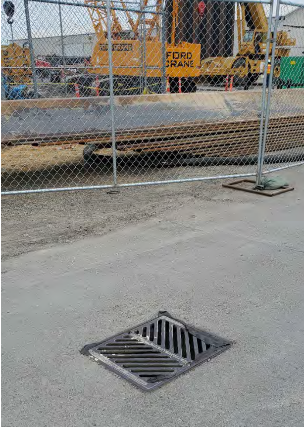
Photo 1. Catch basin w/ silt sock
