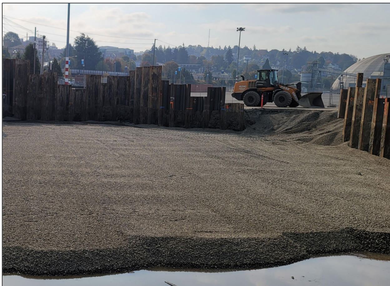
Photograph 11 Backfill Below the Water Table
