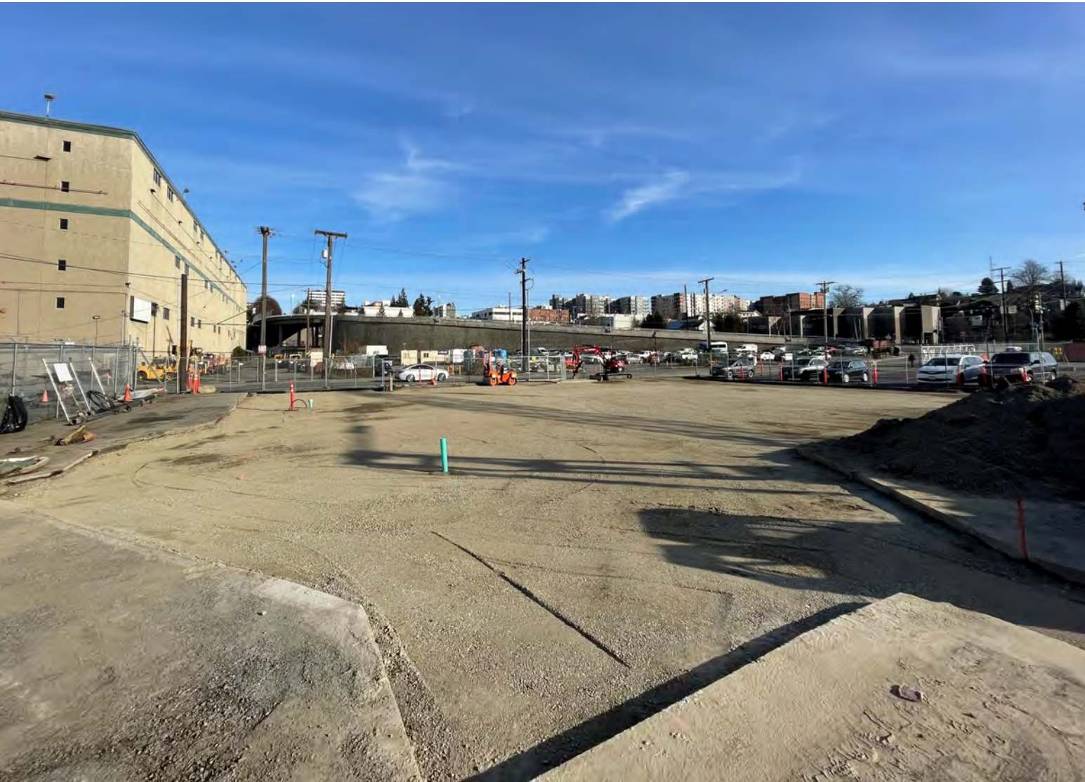
Final Grading with ESR Water and Sewer Connections Above Grade
