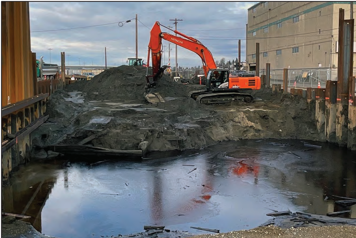
Photo 8. Phase-3 soils removal showing typical soils and milled wood concentration, view to the north.
