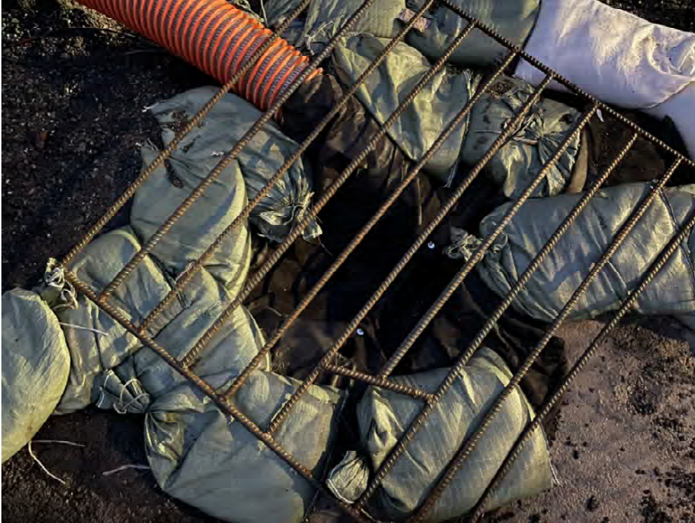
Photo 1. Onsite catch basin with new filter installed
