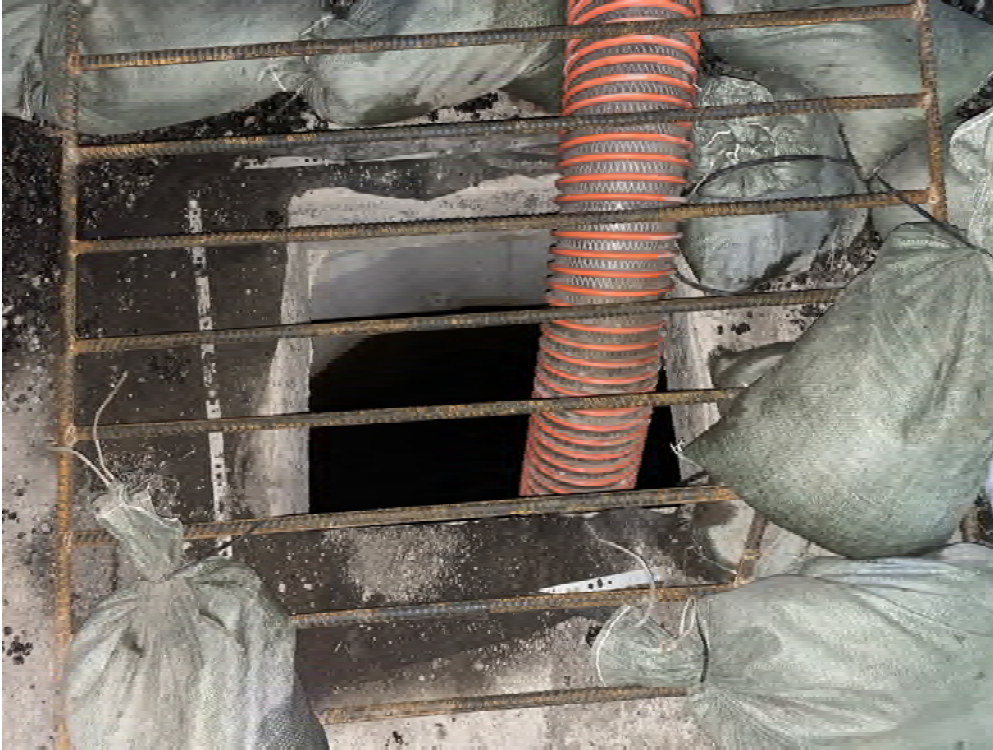
Photo 1. Onsite catch basin in need of filter
