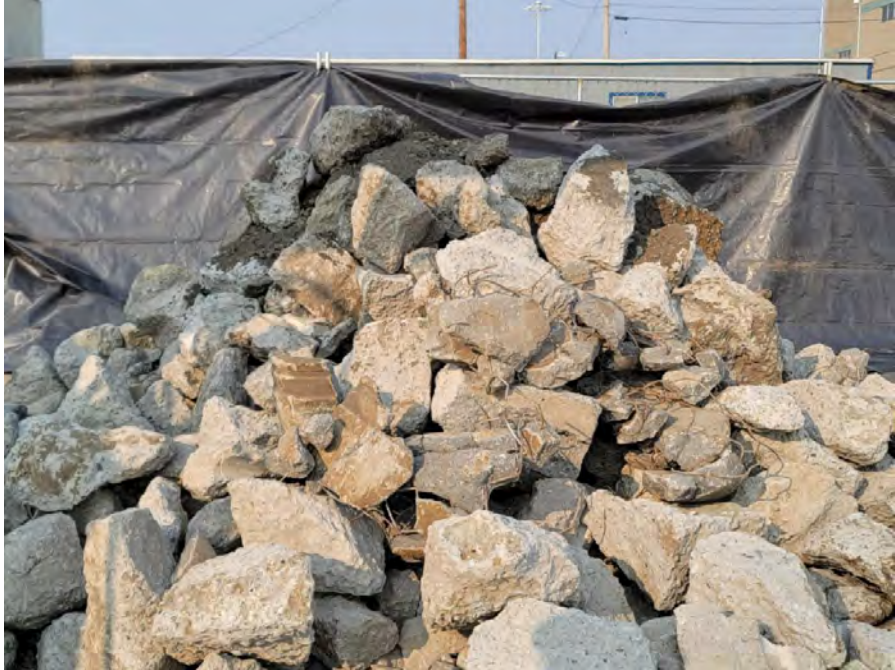
Concrete Footing Breakup
