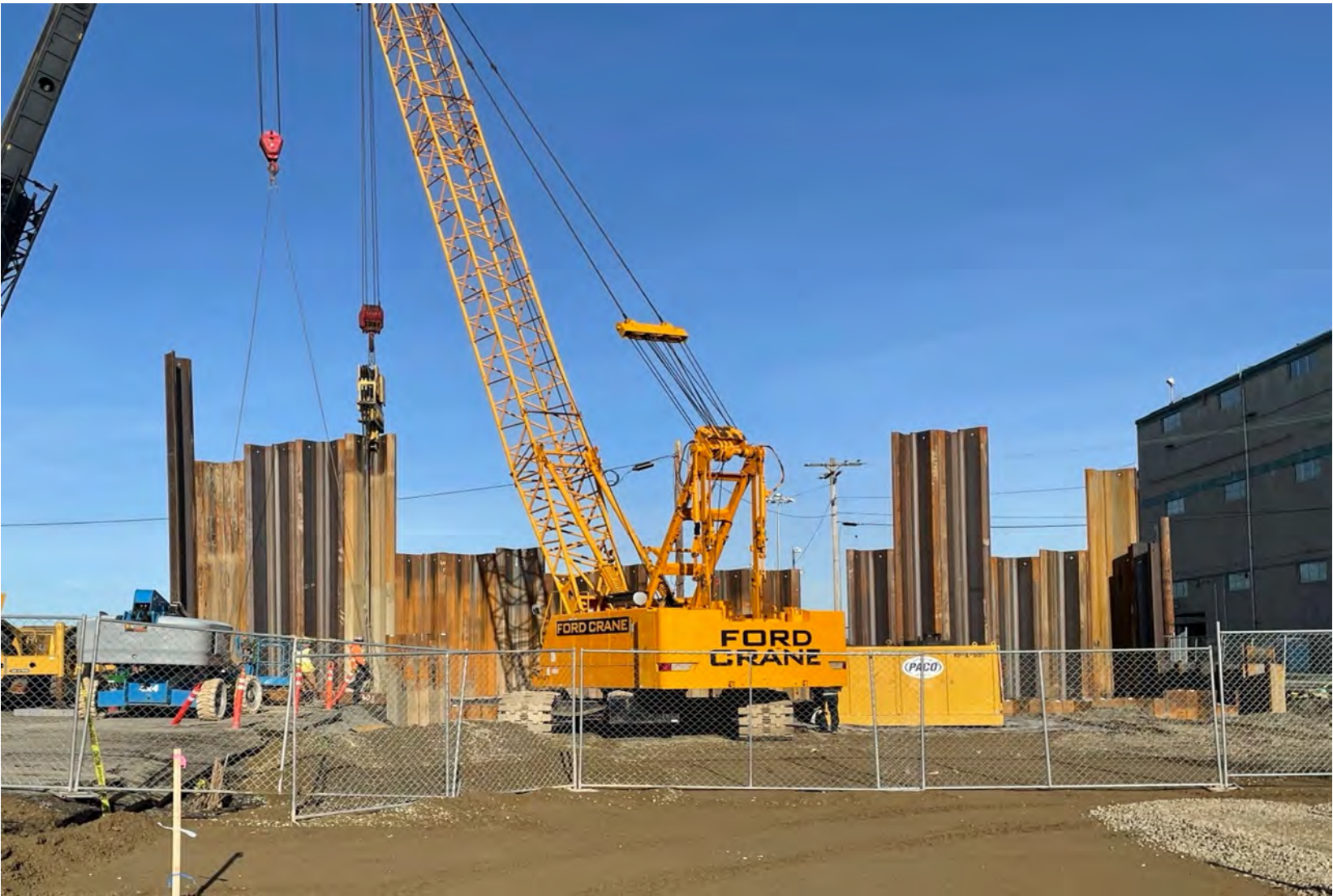
Phase 4 Shoring Installation
