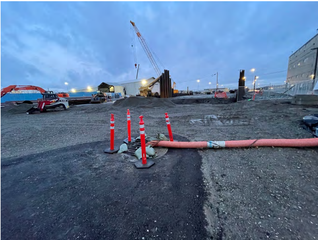
Photo 2. Drainage path (constructed w/ asphalt) leading to new permanent catch basin
