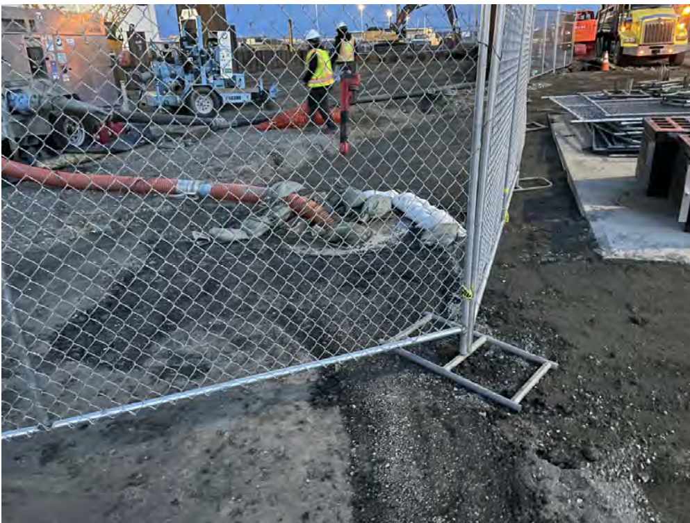
Photo 2. Onsite catch basin in need of filter
