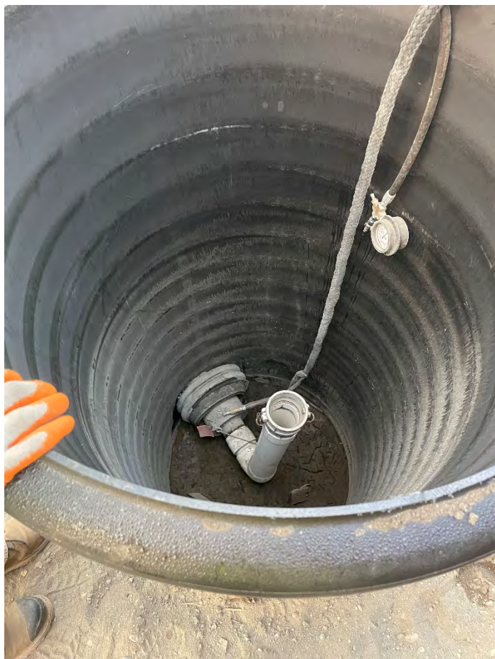
Photo 2. One of three new sump/catch basins currently being installed. Will cut down to grade and have high/low floats with filter to collect and filter groundwater/surface flow.
