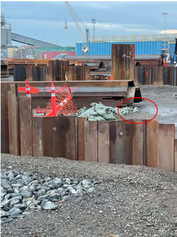
Photo 2. Decommissioned temporary catch basin
