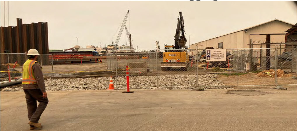
Construction Entrance with Aggregate Base
