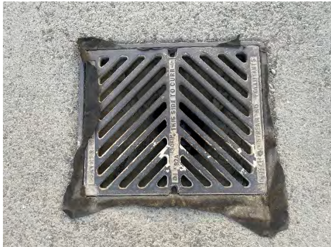
Photo 1. Catch basin with repaired filter.
