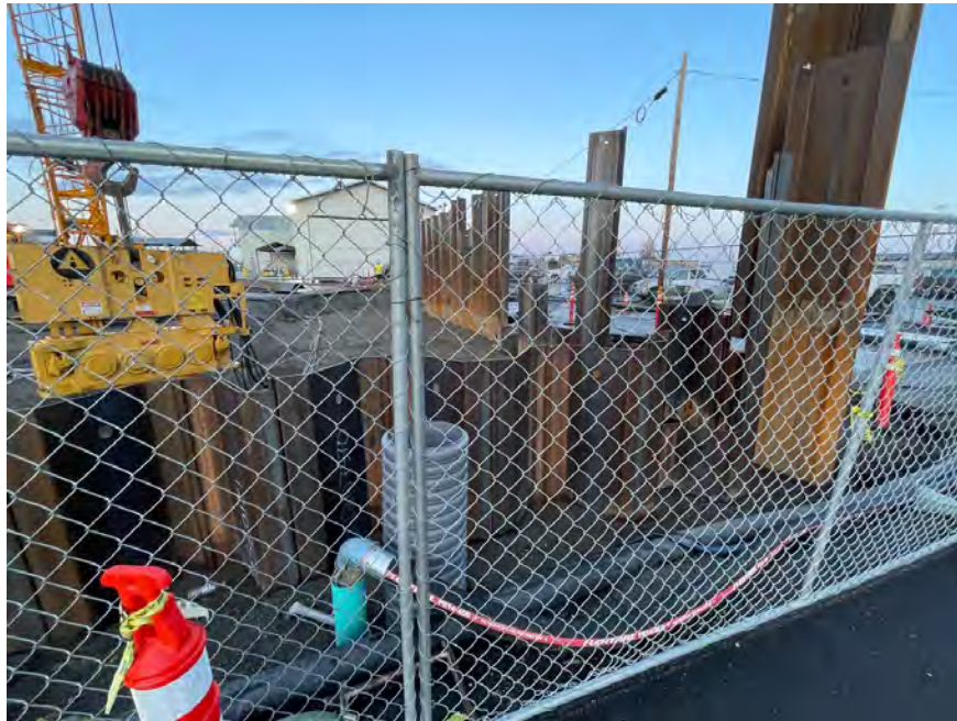
Photo 1. Diversion line to sewer system.
