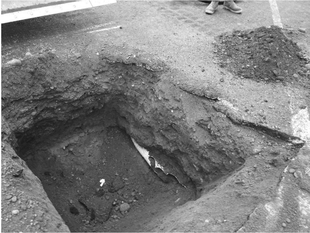
Photograph 3: Drain field test pit PH232-5, showing fill soils, piping, and native soil
