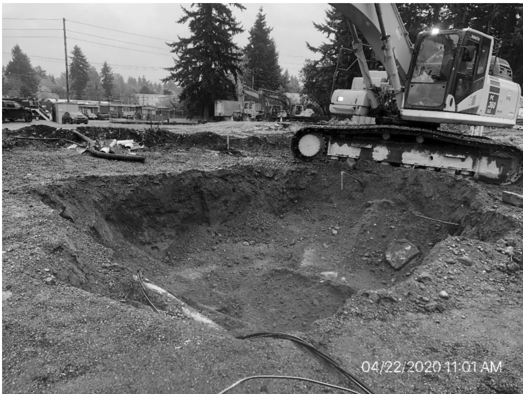
Photograph 6: Remedial excavation
