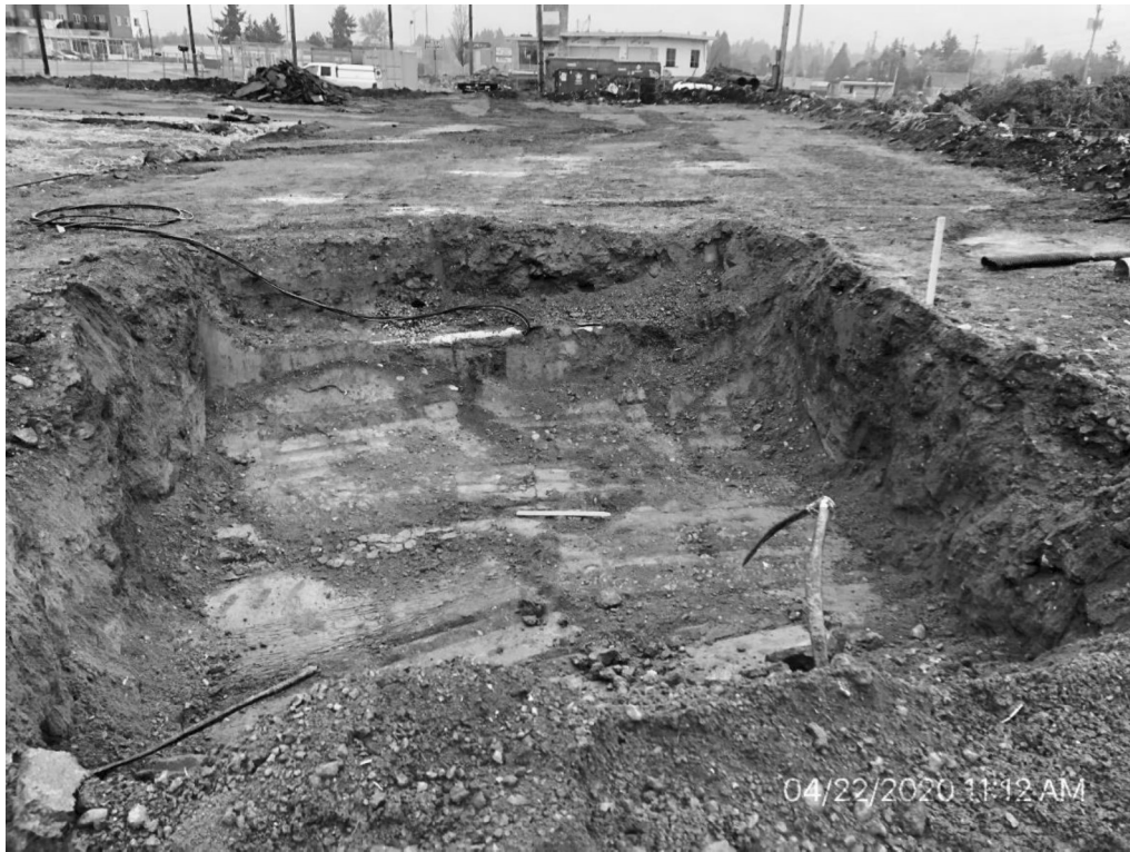
Photograph 7: Remedial excavation, final extent. Sample locations staked.
