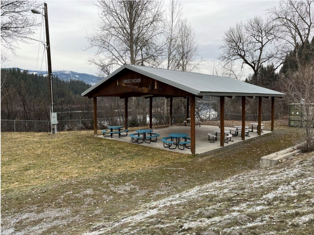
Photo 3: City Park and Structures - from the west
