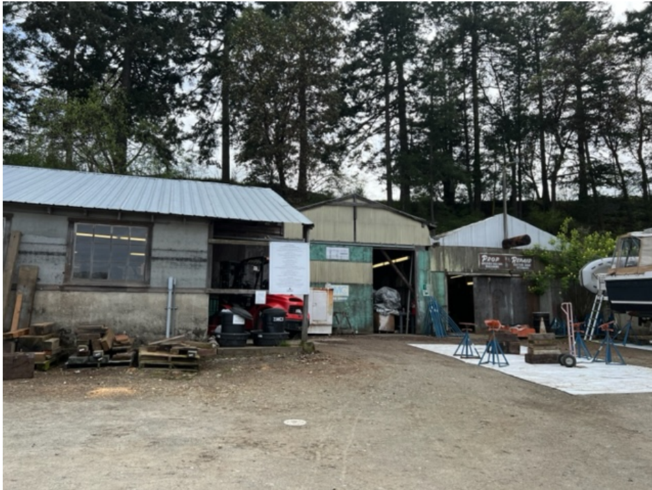
South side of Office Building and Bays 1 and 2
