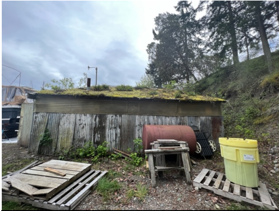
West side of Bay 3
