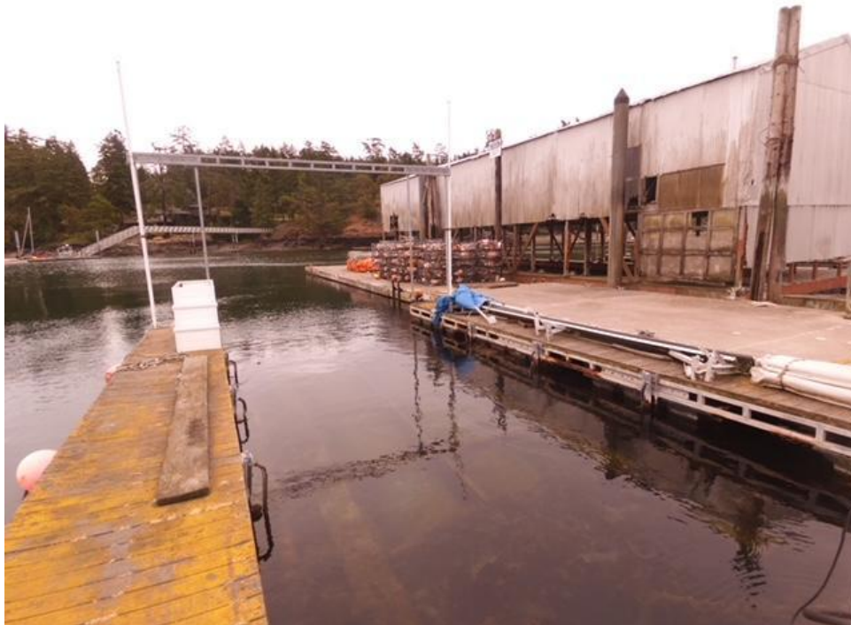
Figure 3. Looking east at survey area near covered moorage at the seaward edge of existing structures.
