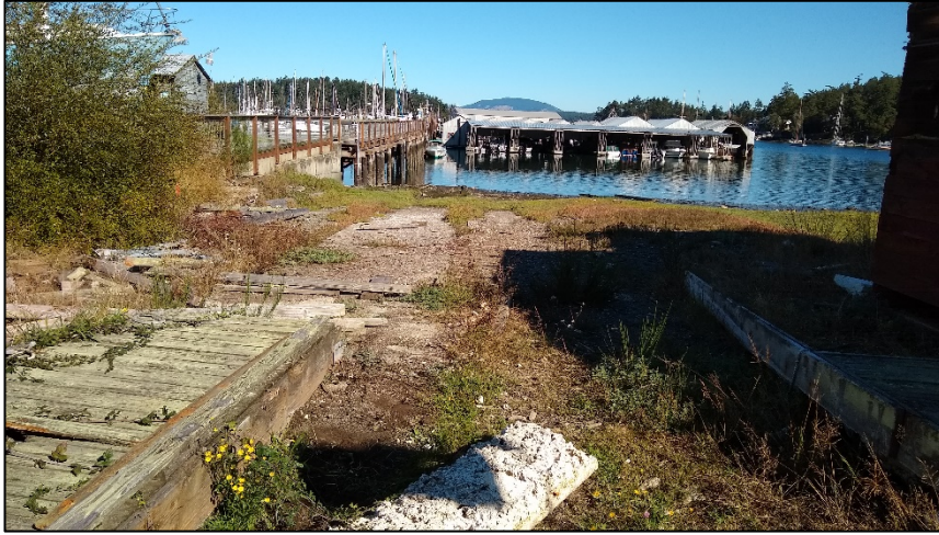
Photo 1. Concrete boat ramp at northwest portion of study area, facing north.
