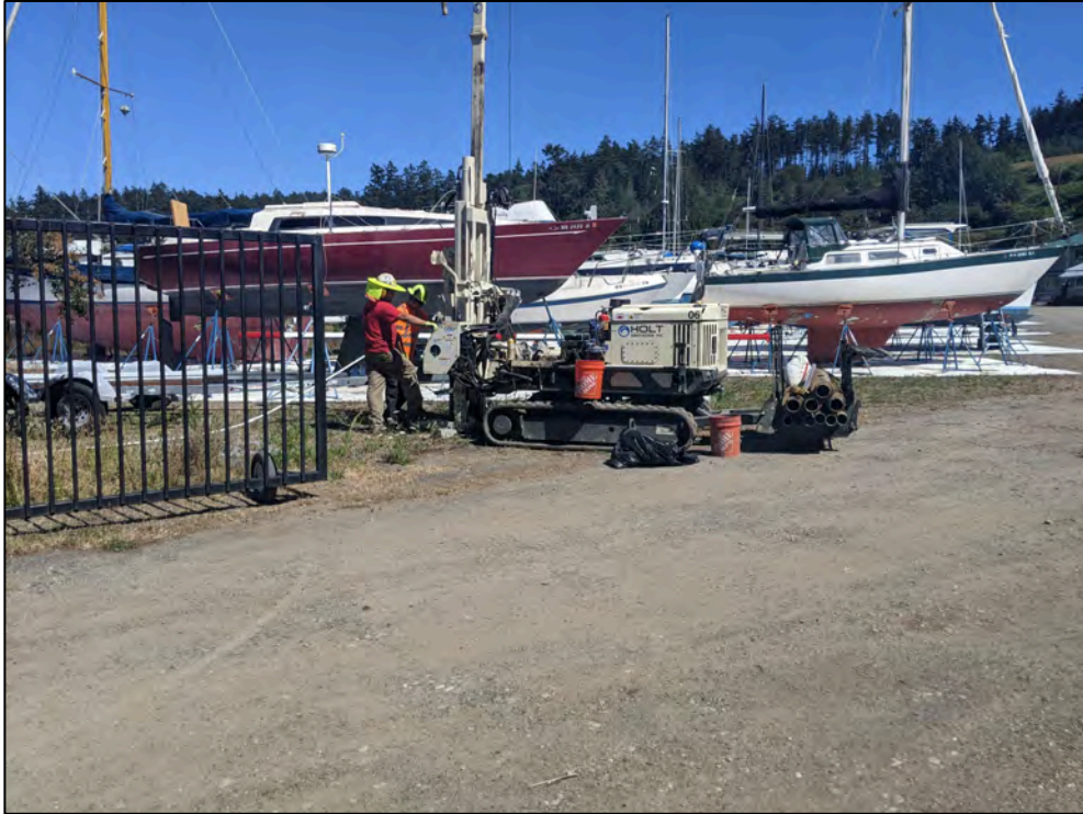
Figure 11. Boring BLWA-11 in progress, view to the northeast.
