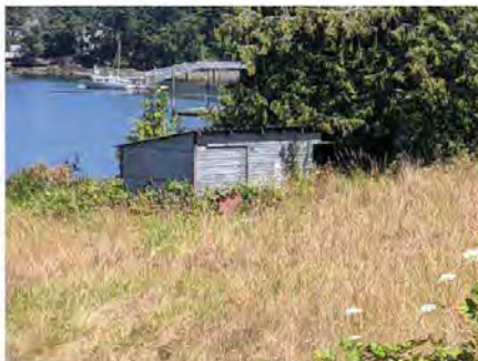
Southwest elevation of shed 1
