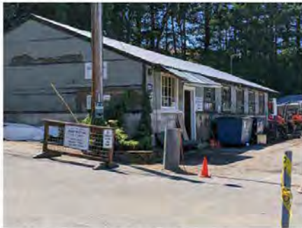
Northeast elevation of building
