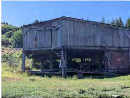
North face of building
