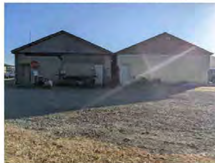
Southwest face of building
