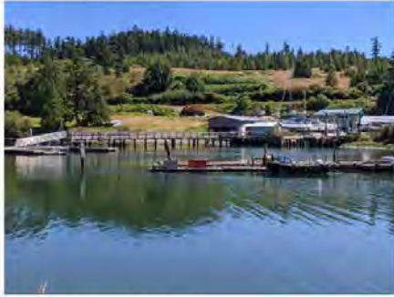
Pier overview at shoreline
