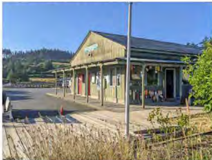
North elevation of building entrance (northeast end)
