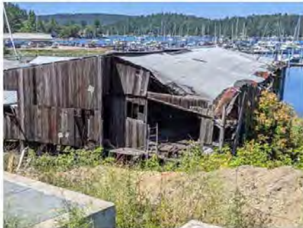
Southeast elevation of building
