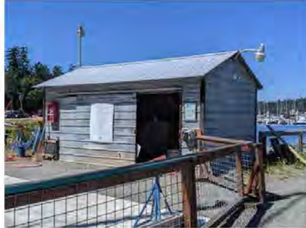
Southeast elevation of shed
