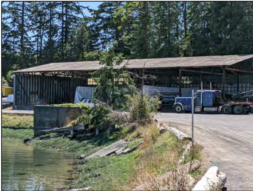
Figure 21. Image of the northeast elevation of the ca. 1970 Shipyard Cove Marina Storage Building (DAHP Property # 728944) at 1063 Turn Point Rd, view to the southwest.
