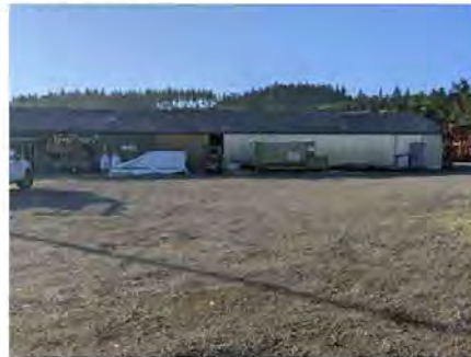
Northwest face of southeast half of building
