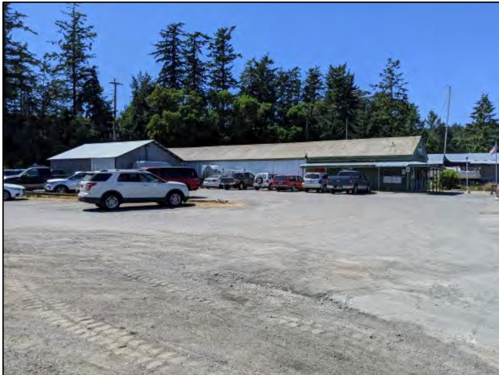
Figure 20. Image of the east elevation of the ca. 1970 Shipyard Cove Marina Office building (DAHP Property # 728943) at 1063 Turn Point Rd, view to the west.
