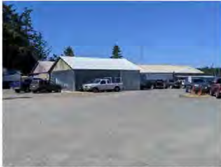
South elevation of building
