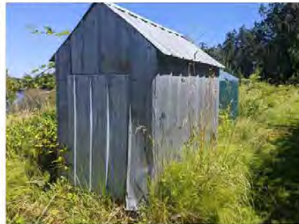
West elevation of Shed 2
