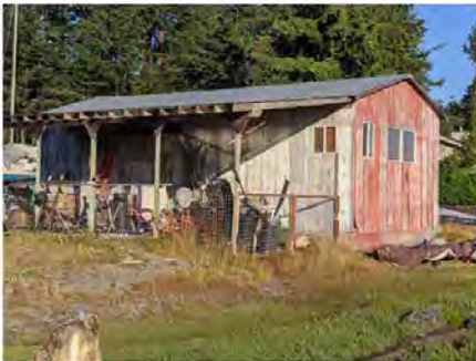
Northeast elevation of building
