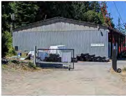
East face of building
