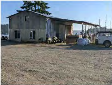
Southeast elevation of building
