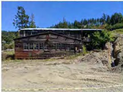
West face of building
