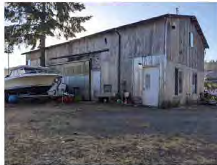
Southwest elevation of building
