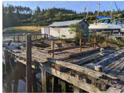
Northwest elevation of shed and relic pier
