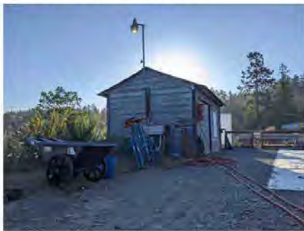
West elevation of shed
