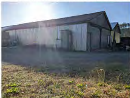
West elevation of building
