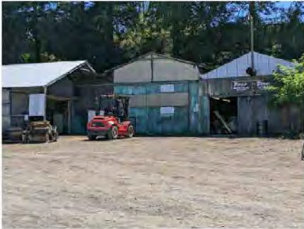
North face of wing
