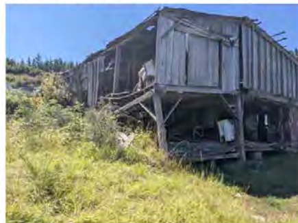
Northeast elevation of building
