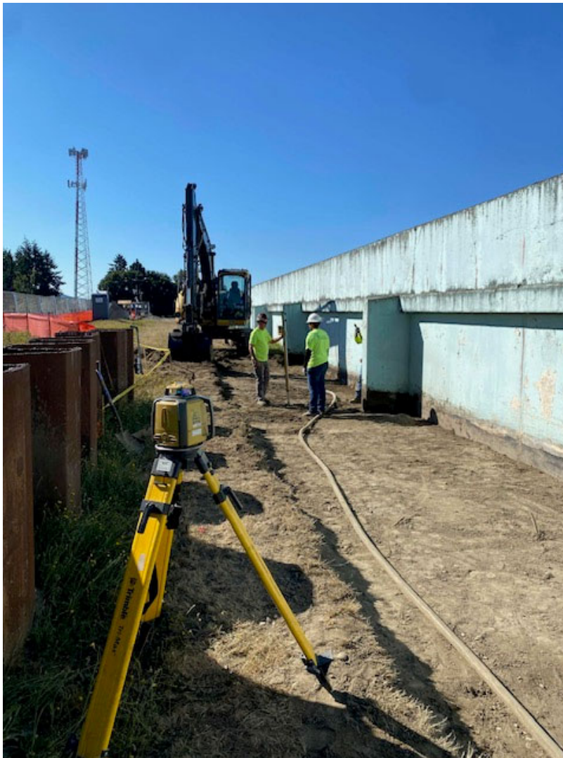
Photograph 5 PCB-Impacted Soil Excavation Adjacent to the Sedimentation Basin
