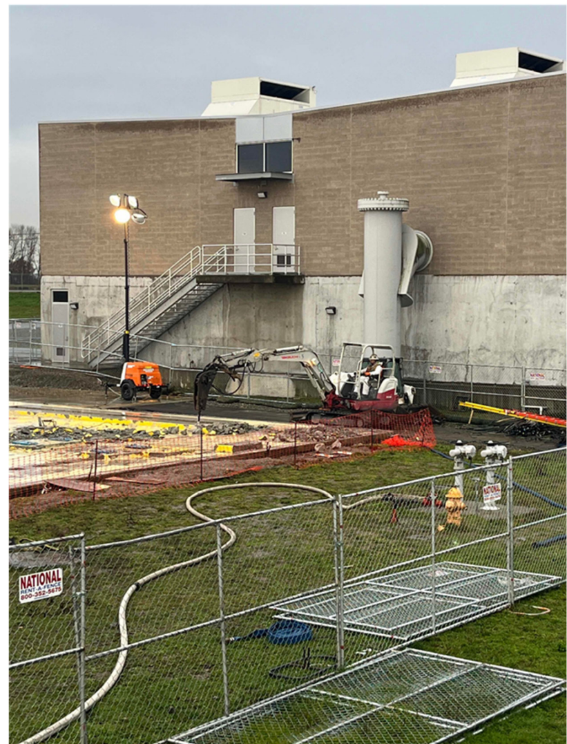
Photograph 14 Demolition of the Pedestals on the Pump Room Slab
