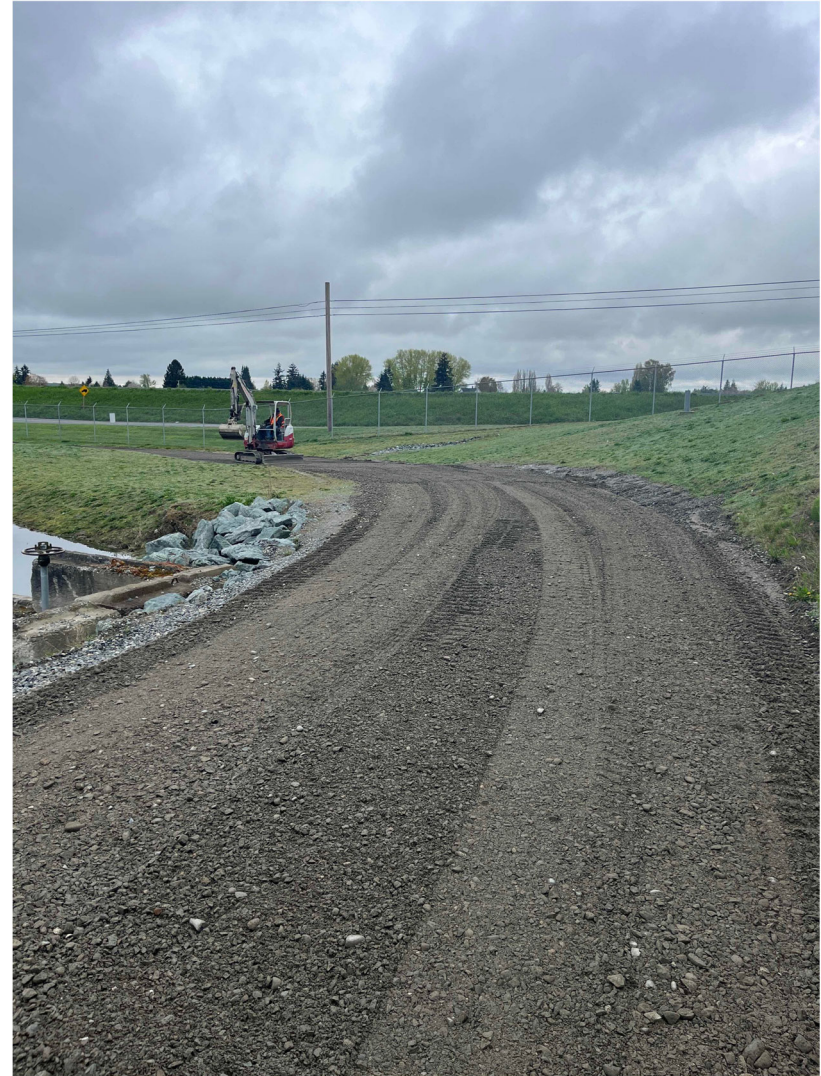
Photograph 18 Resurfacing the Gravel Roadway
