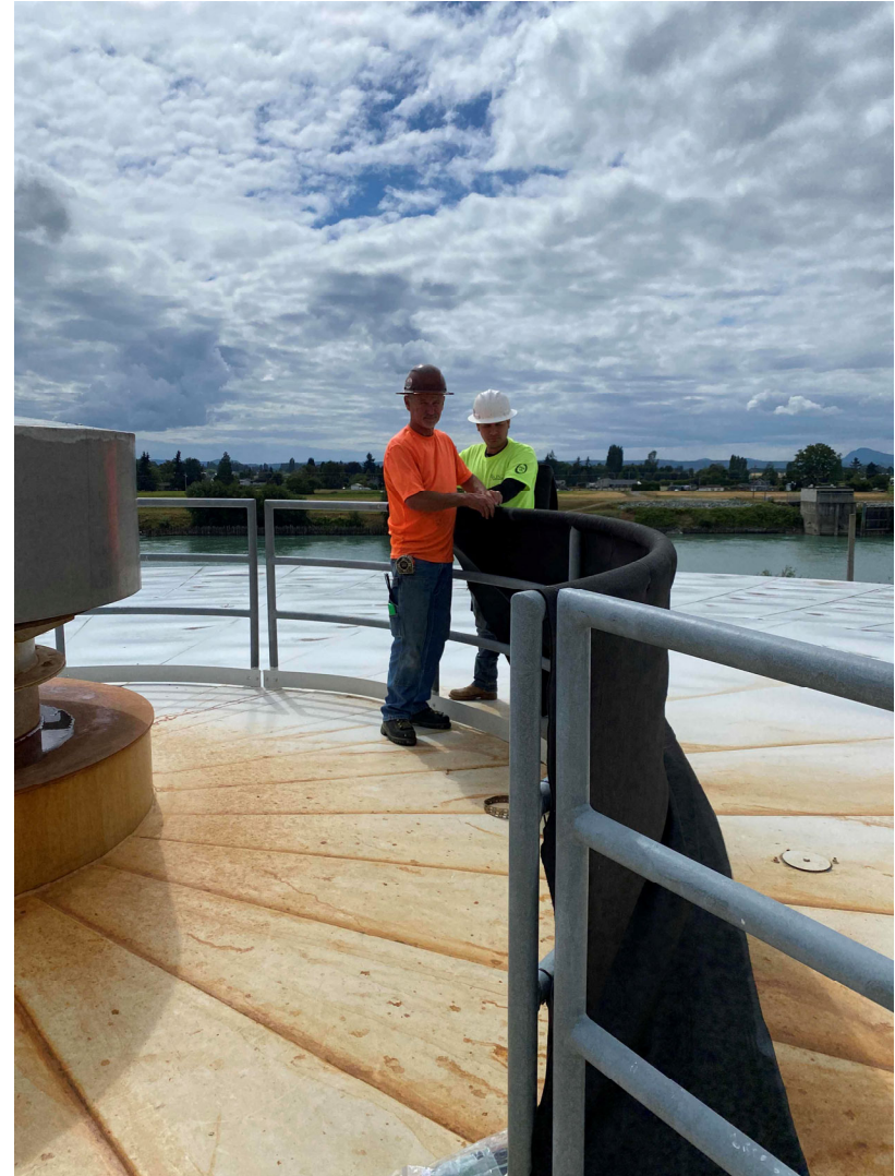
Photograph 4 3 Kings Installing Dust Protections on the Active Clearwell
