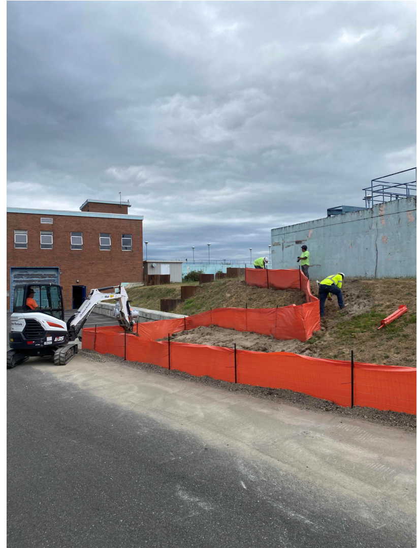
Photograph 2 3 Kings Installing Silt Fencing
