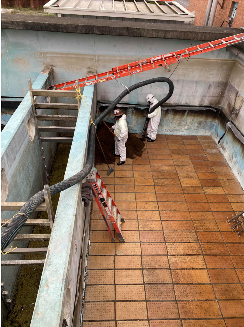
Photograph 8 Filter Media Removal with the Vacuum Unit
