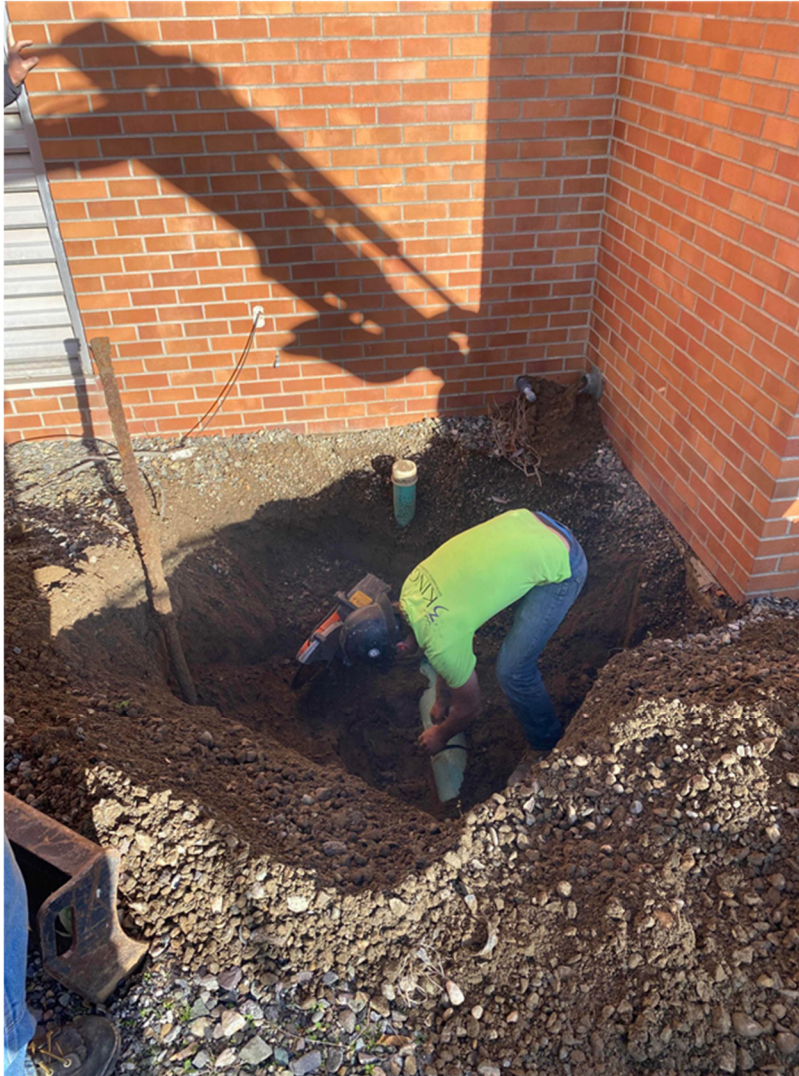
Photograph 6 3 Kings Disconnecting the Sanitary Sewer Line
