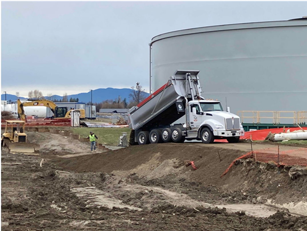
Photograph 12 Backfill of the Sedimentation Basin
