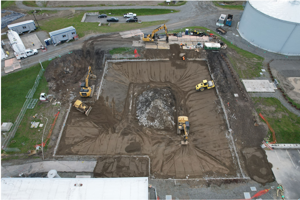
Photograph 16 Backfilling of the Filtration Basin and Administration Building
