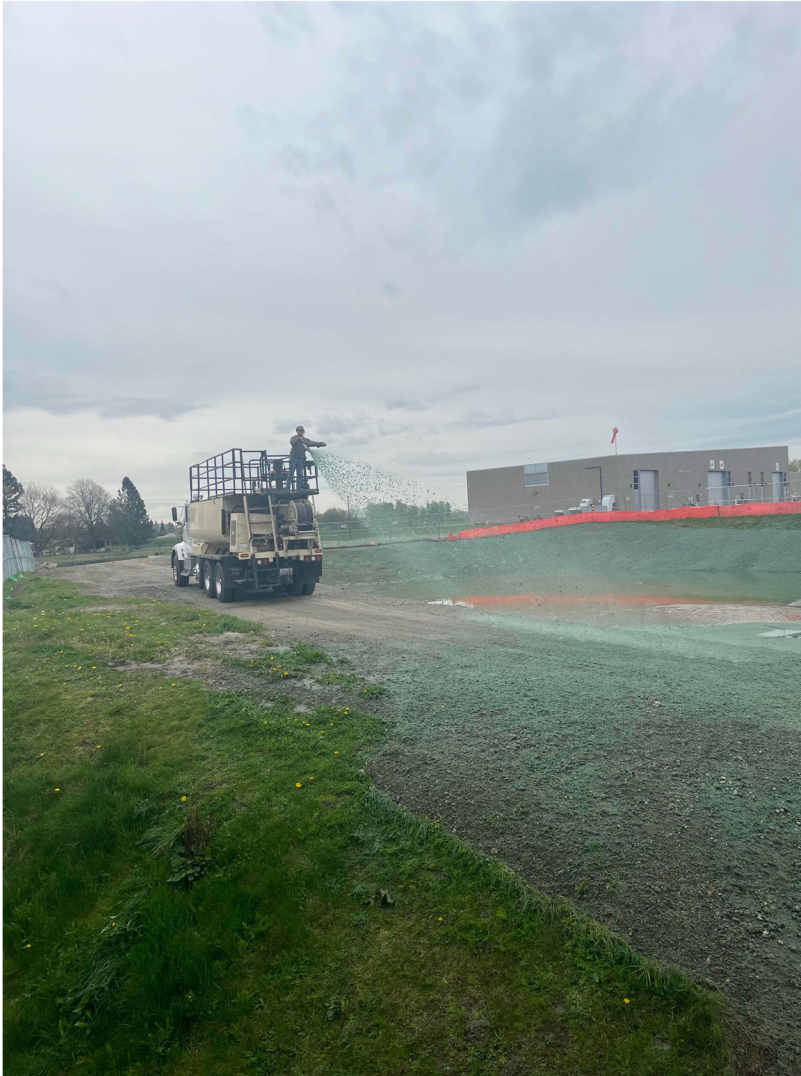
Photograph 17 Hydroseeding the Sedimentation Basin
