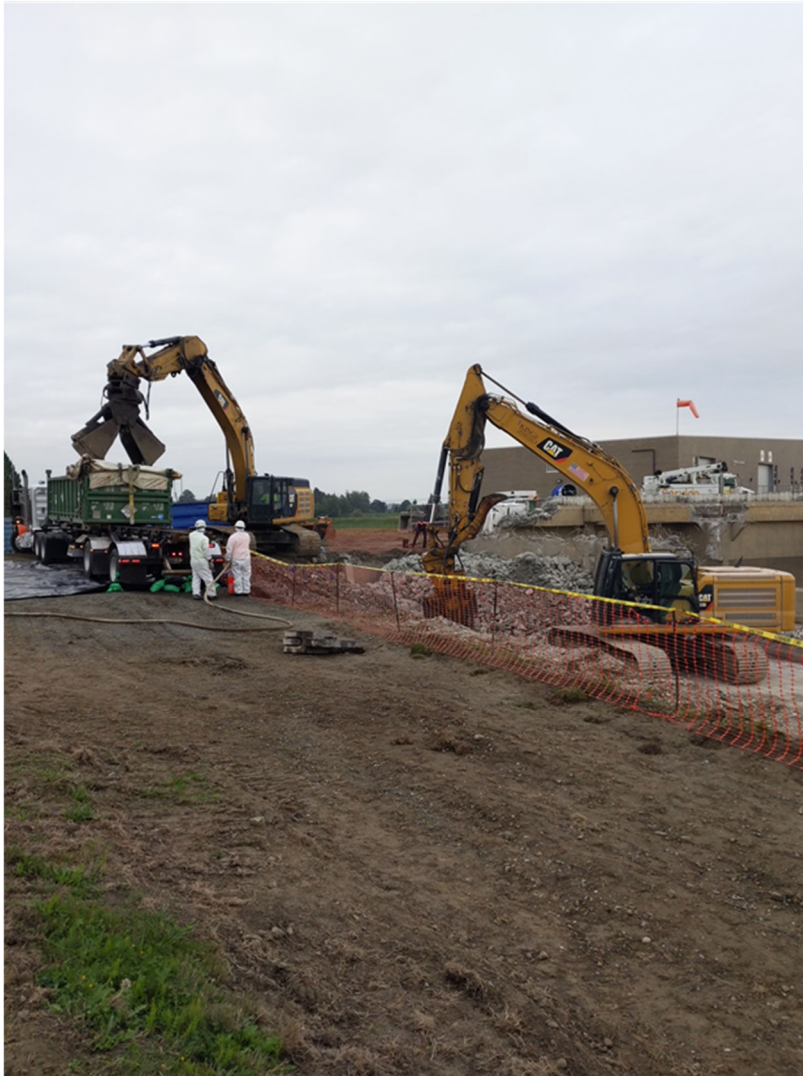
Photograph 11 PCB BPW Demolition Debris Loadout
