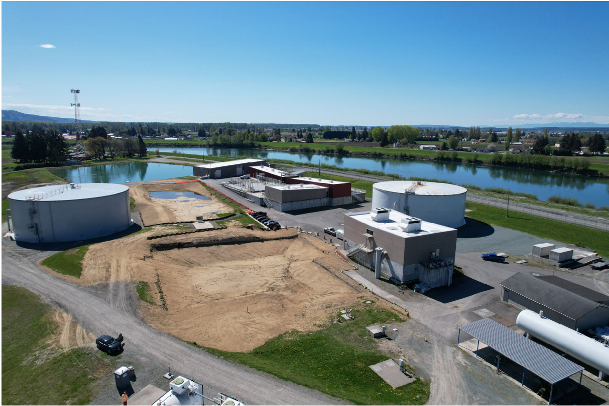
Photograph 19 Final Site Conditions at 3 Kings Demobilization on April 18, 2024
