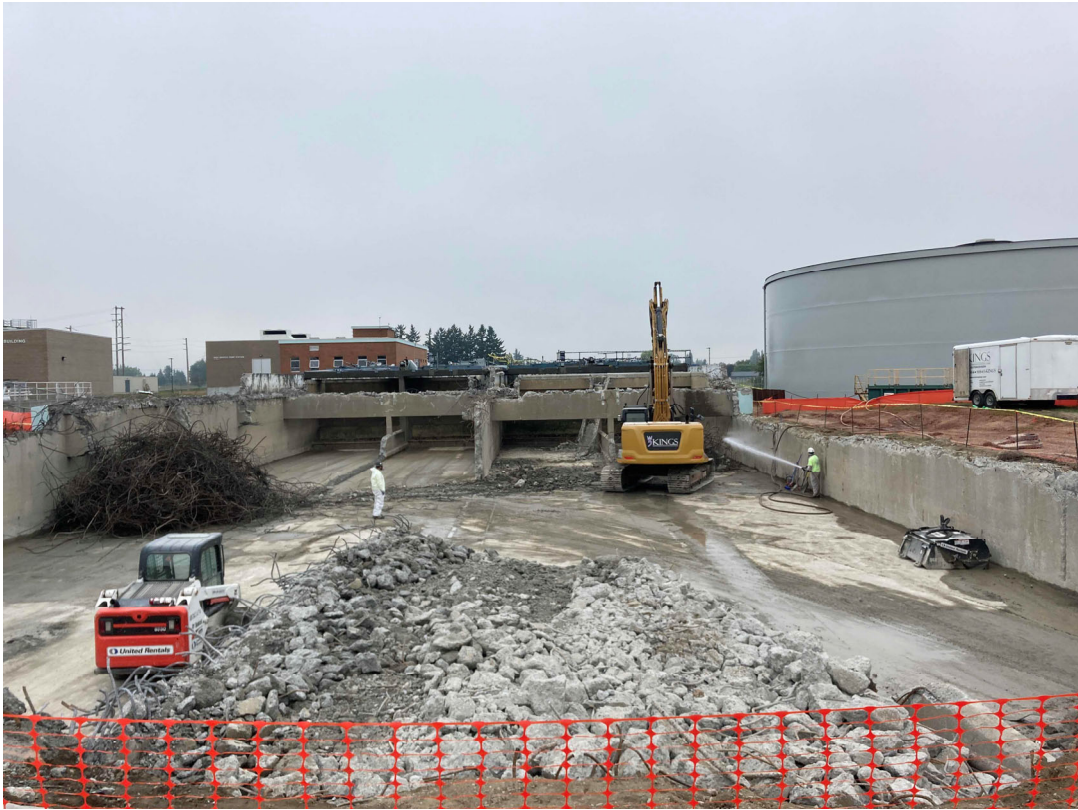
Photograph 10 Sedimentation Basin Demolition
