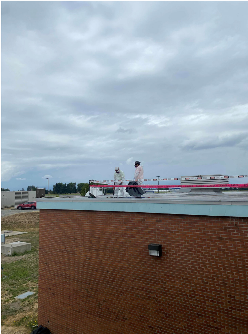
Photograph 7 Abatement of Asbestos Caulking Around the Roof Drains
