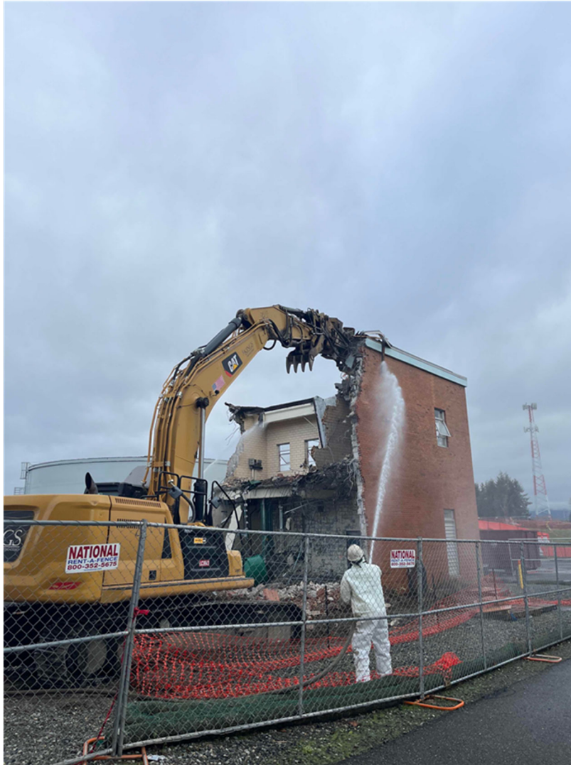
Photograph 13 Demolition of the Administration Building
