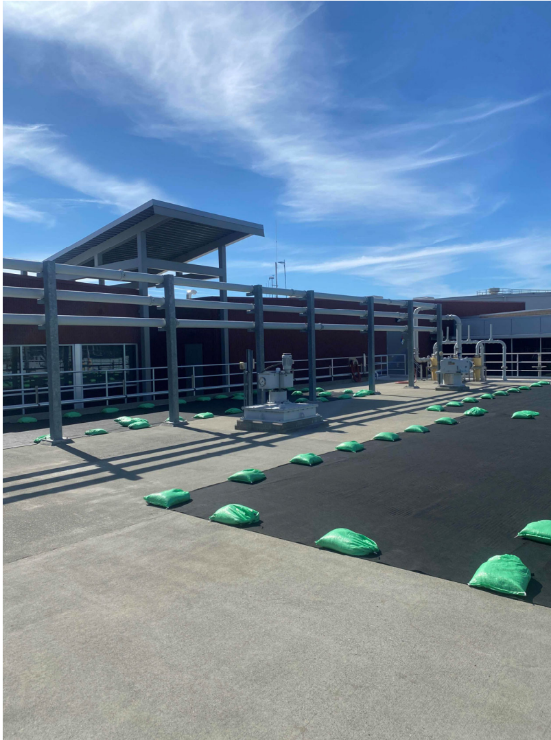
Photograph 3 Dust Protections Installed on the Active Sedimentation Basin
