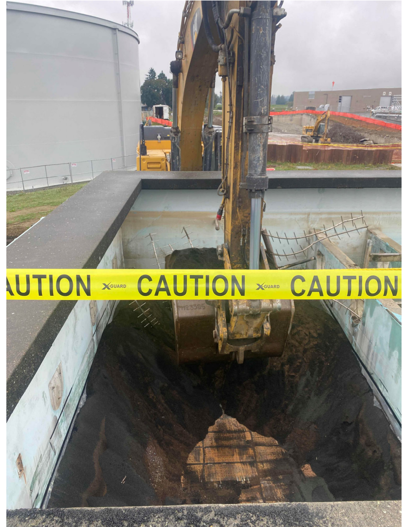
Photograph 9 Filter Media Removal with the Excavator
