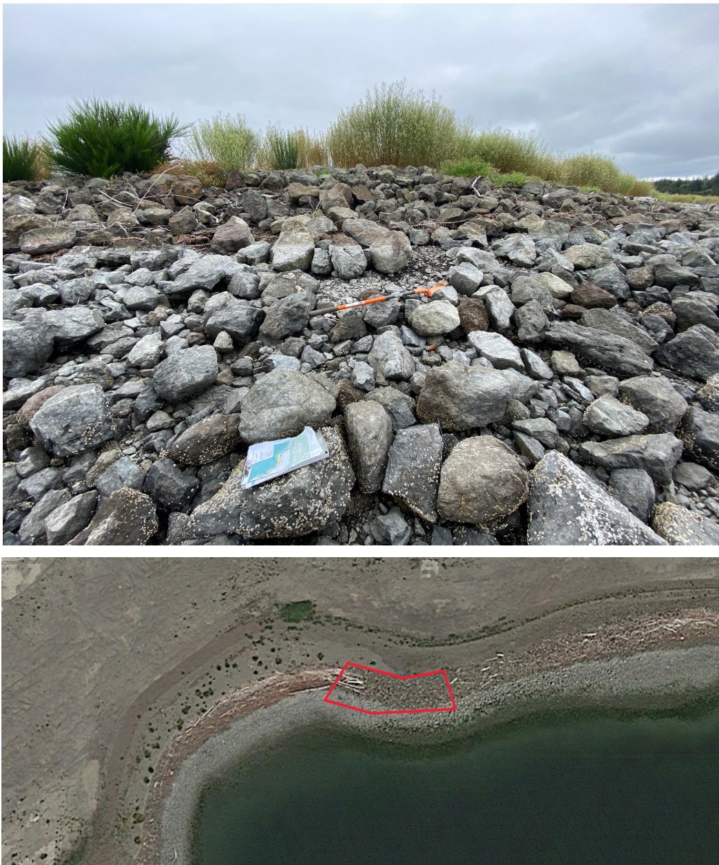
Figure 7 SMA-2 Repair Area 5 and Aerial View of SMA-2 2020 Repair Area
