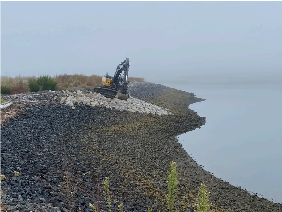
Figure 8 Repaired SMA-2 Intertidal Cap
