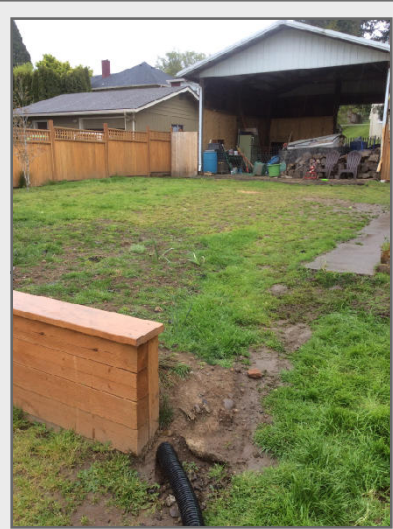
1 Former blacktop driveway exclusion area
