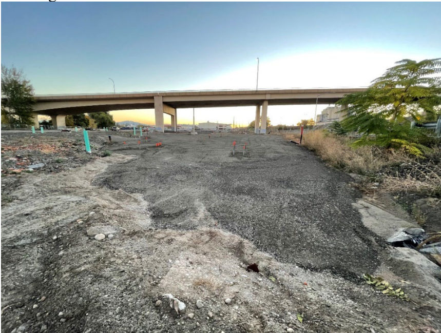
Photograph 4. View of proposed Building 2B footprint with building footprint excavation backfilled and stormwater cover placed and compacted. Looking east. Stormwater collection depression is in foreground.
