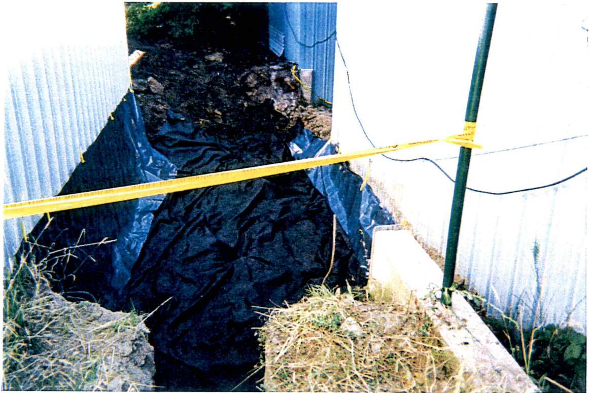
Photograph 3 - Site Following PCS Excavation with Migration Barrier Installed. View North.
