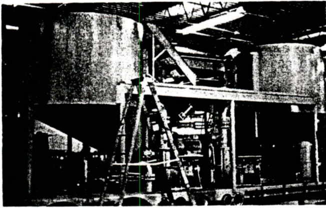
Fig. 7. Colloidal mixing plant equipped with two 6-cu-yd capacity mixing chambers. (Courtesy of Great Lakes Construction Co., Spring Lake, Mich.)
