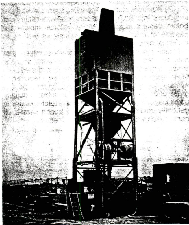
Fig. 8. Paddle mixing plant. Cement scale, surge hopper, and storage silo located above two 6-cu-yd capacity mixing chambers.
