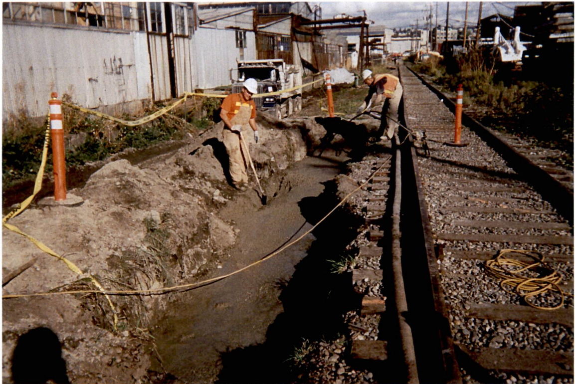
Photograph B-3 Protection of water line with concrete.
