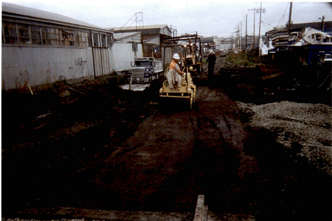
Photograph B-4 Compaction of fill beneath railroad tracks.
