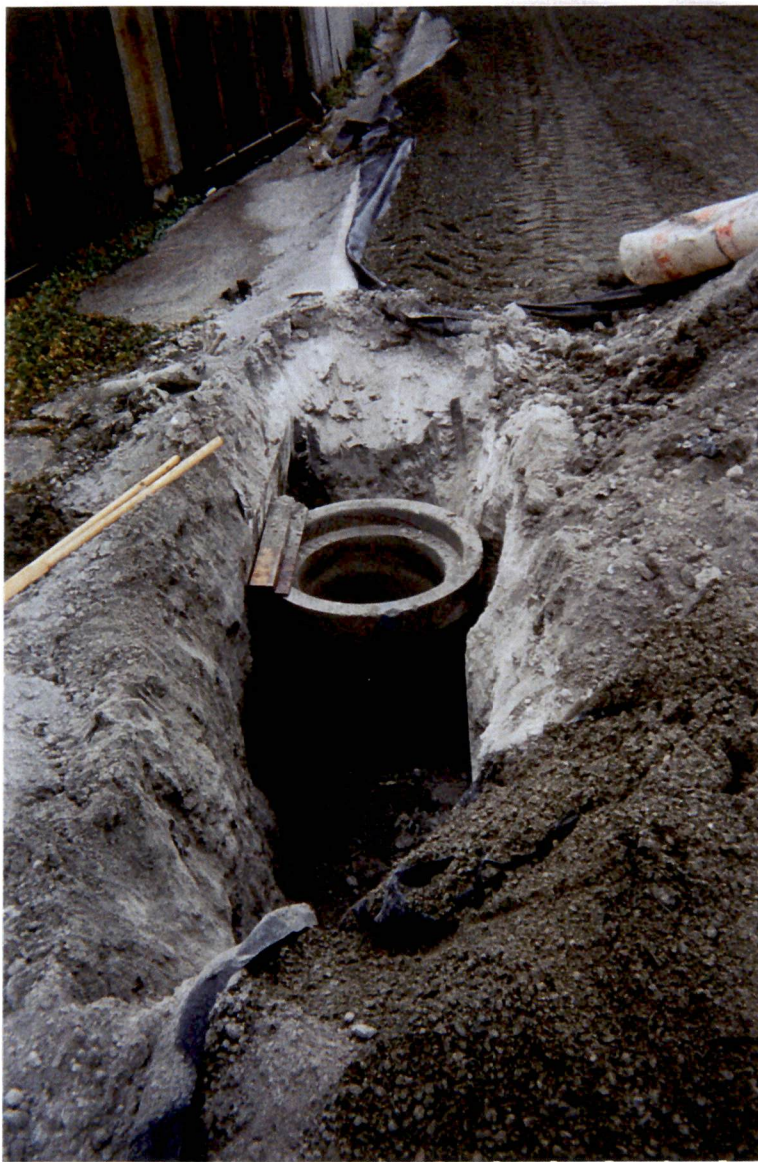
Photograph B7 Restoration of storm drain in fill area north of railroad tracks.
