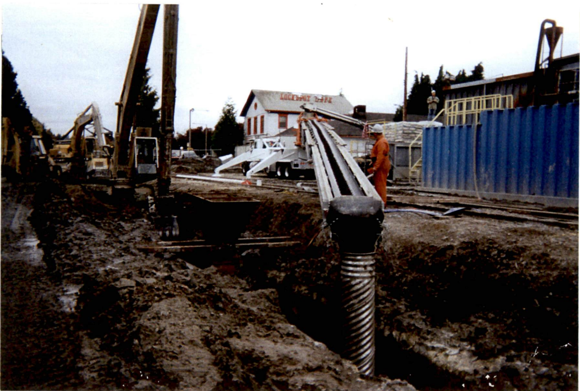
Photograph B-6 Filling grates with iron-sand mixture.
