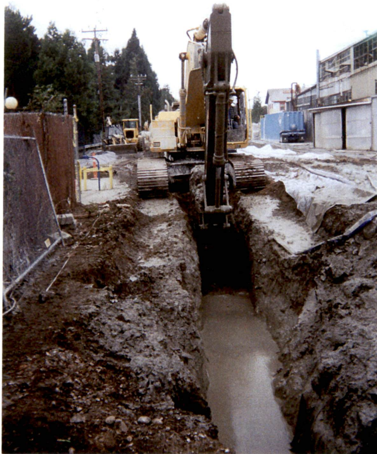
Photograph B5 Excavation of trench for cement-bentonite slurry
