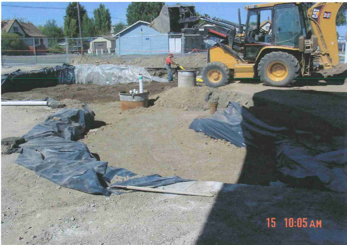
Unaffected overburden placed and compacted as backfill
