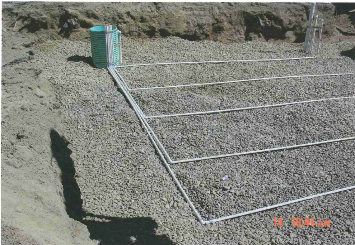
Distribution piping – note shallow rock in sidewall of excavation.
