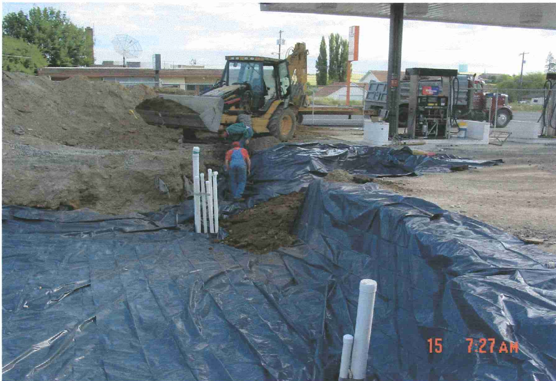
Filter fabric and plastic cover over drain rock – note vent & observation pipes
