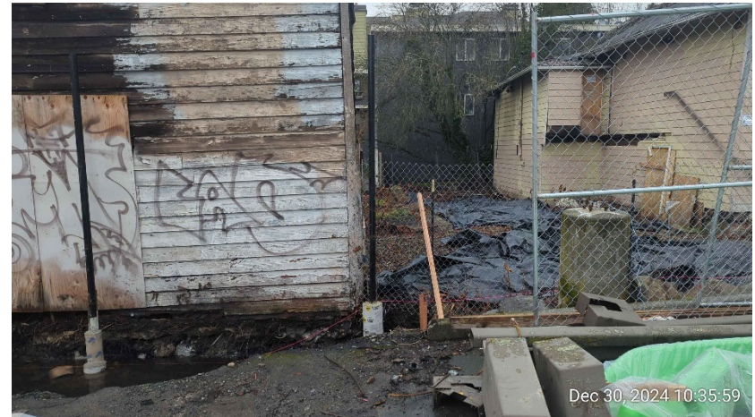
View of the NW corner of the site where posts were being installed for a new fence along the northern property boundary. The fence was designed to span the designated restricted area with no penetrations in this area.
