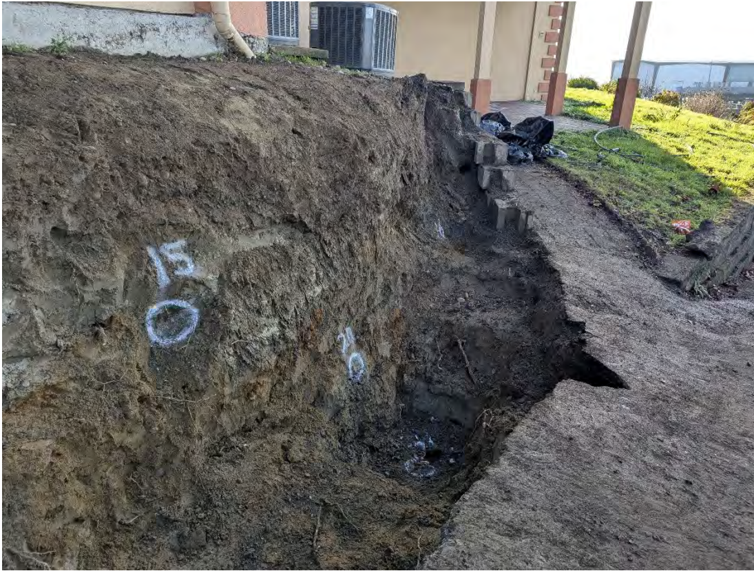
View of the final excavation and sample locations near where the perforated pipe ended.
