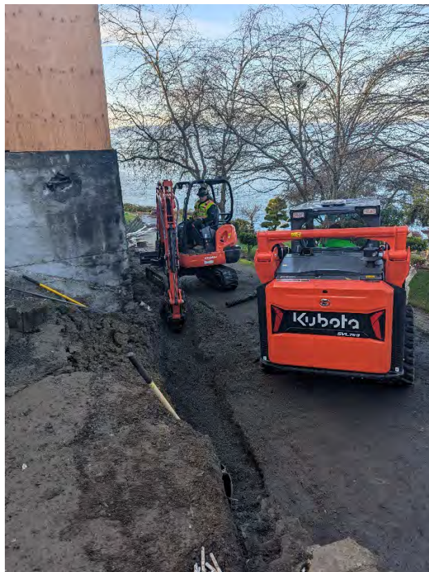
View of the excavation taking place on January 8, 2024. Material was excavated with the mini excavator and then placed in the skid-steer for transport to the dump truck parked along 75 th Place W.
