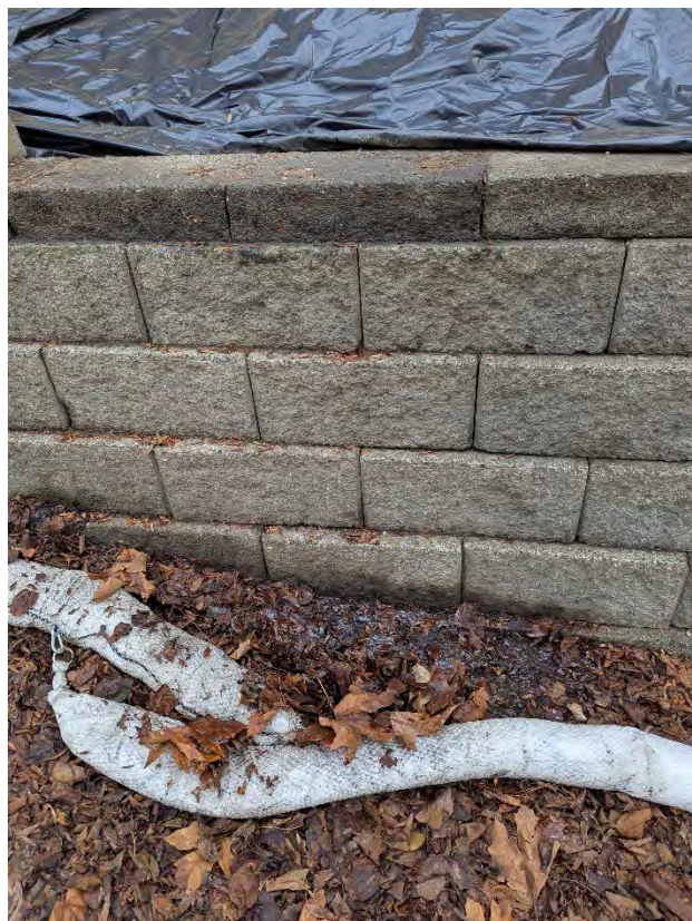
View of oily leaves and dark stained retaining wall blocks beneath the spill area on December 3, 2024.
