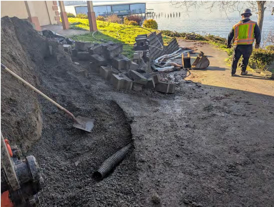
View of perforated pipe extending beneath the asphalt near southern end of the excavation (January 8, 2025).
