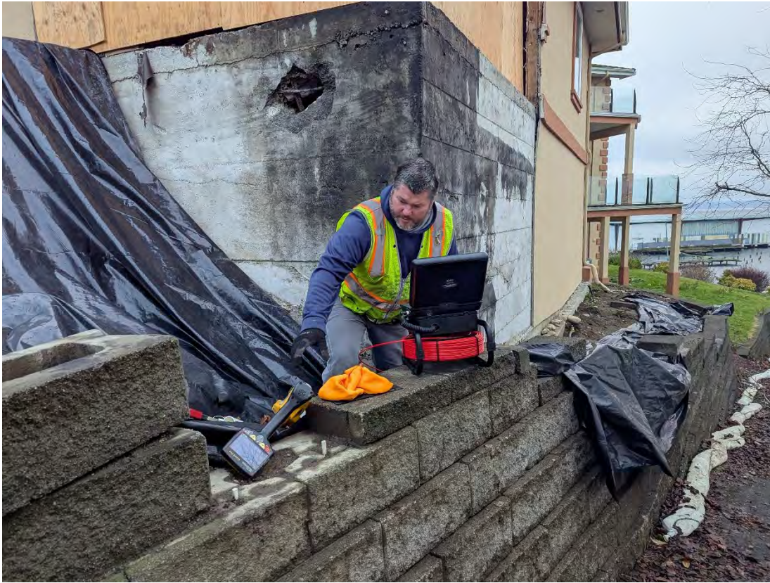
View of the camera and red cable being prepared to evaluate the footing drain system by CNI Locates on January 7, 2025.
