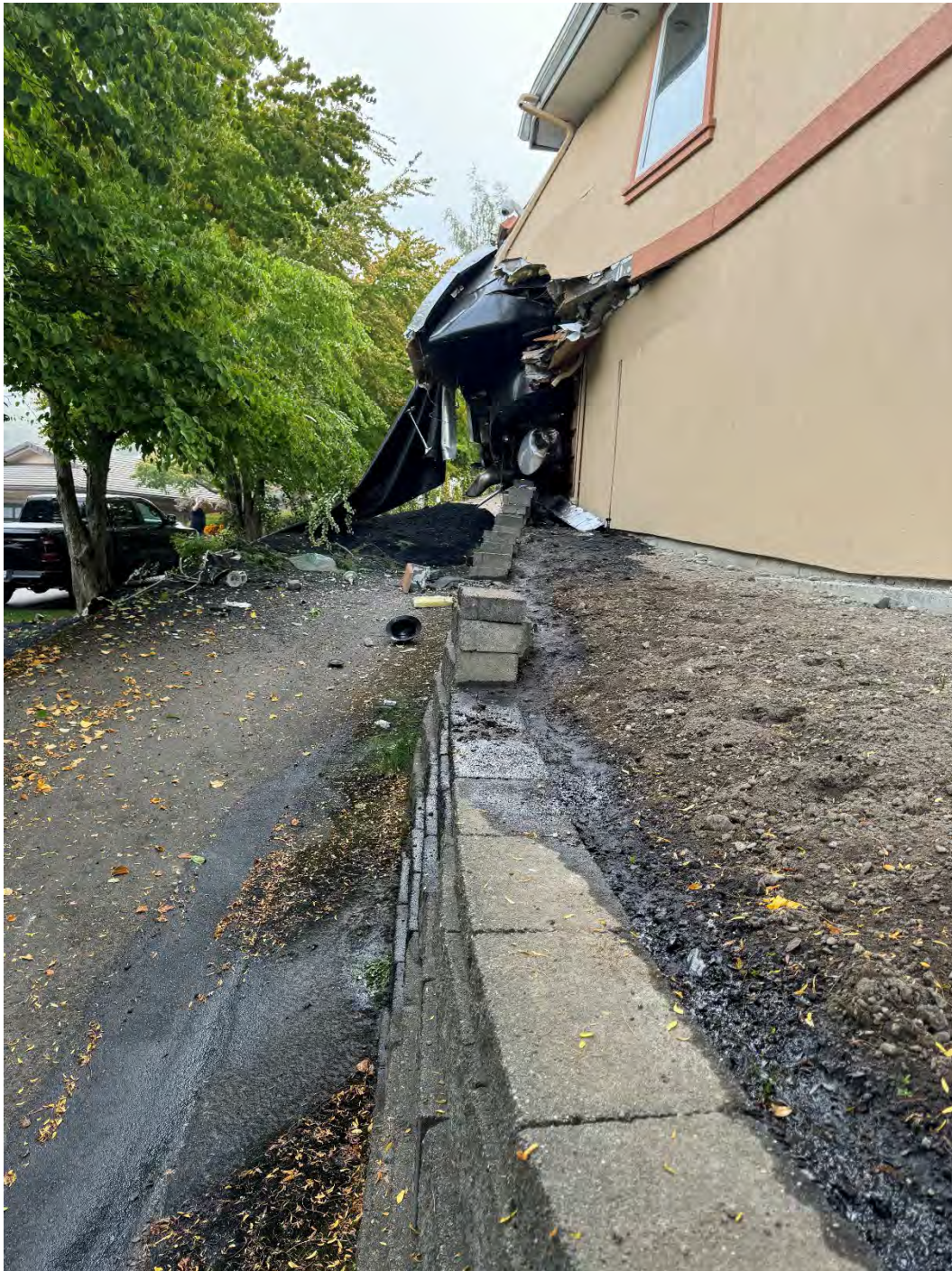
View of diesel spill with notable presence of diesel at northwest corner of the building, along soil edge of retaining wall, and along the base of the retaining wall on the asphalt pathway on September 4, 2024. Photo provided by Rick Nissen, property owner.
