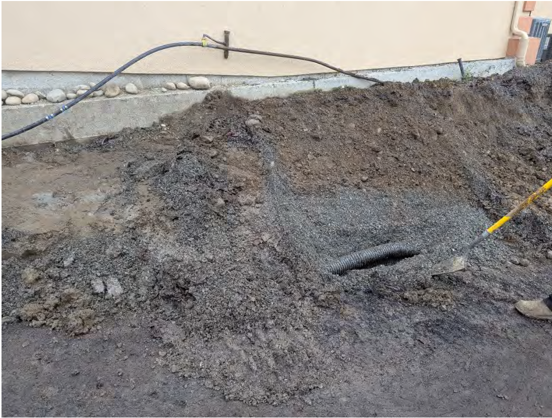
Initial discovery of a black 4" perforated pipe beneath the former retaining wall.
