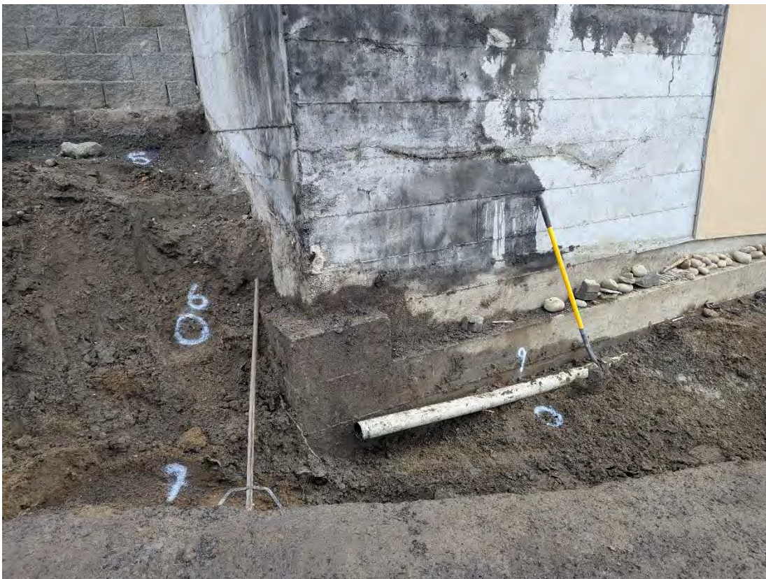
View of sample locations 5, 6, 7, and 9 near the northwest corner of the garage foundation and footing, following excavation.
