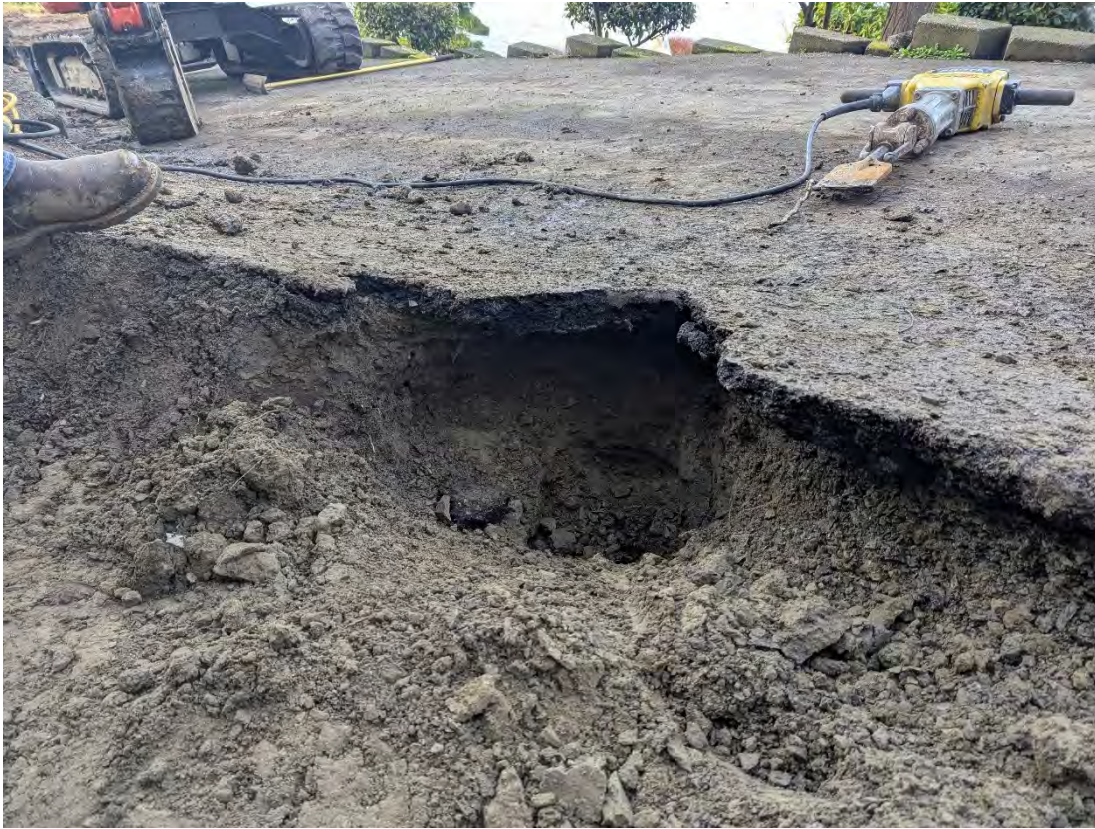
View of location where perforated pipe ended, approximately one to 1.5 feet west of retaining wall beneath the asphalt.
