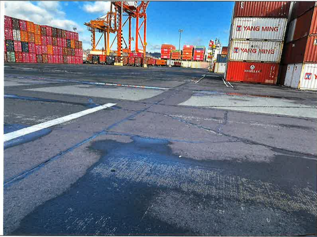
Typical area of crack and joint sealing
