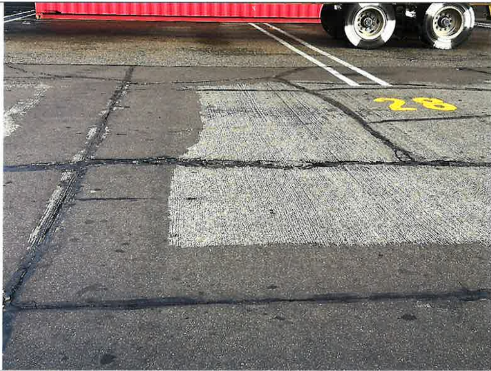
Typical joint and crack sealing in the intermodal yard
