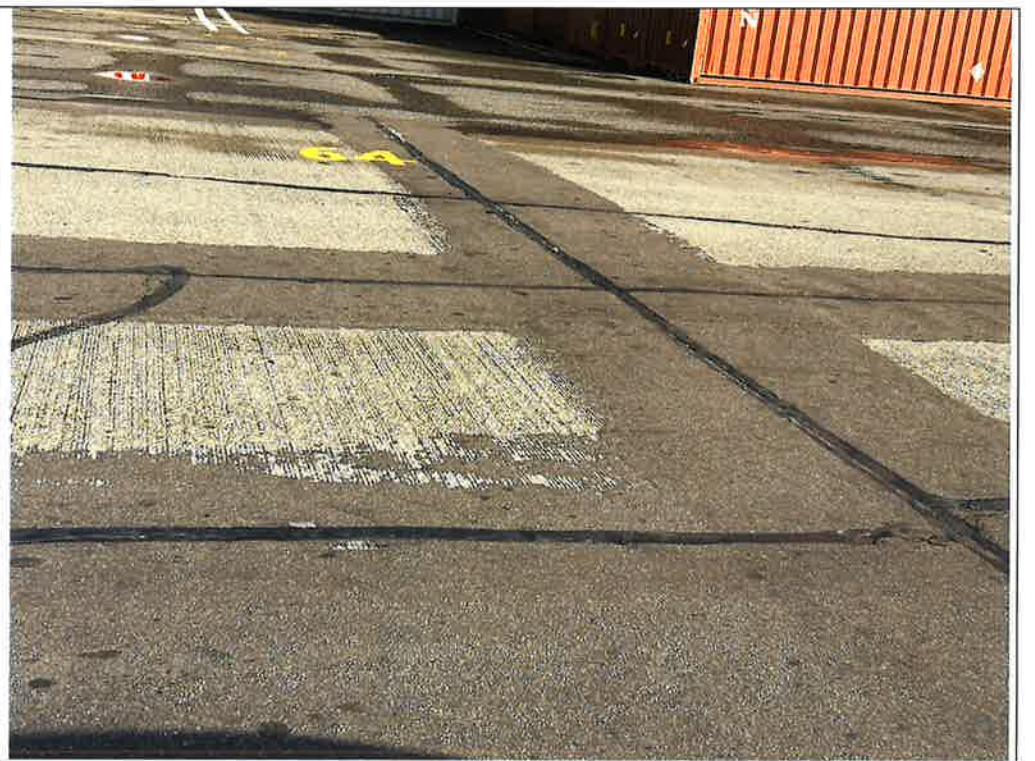
Typical joint and crack sealing.
