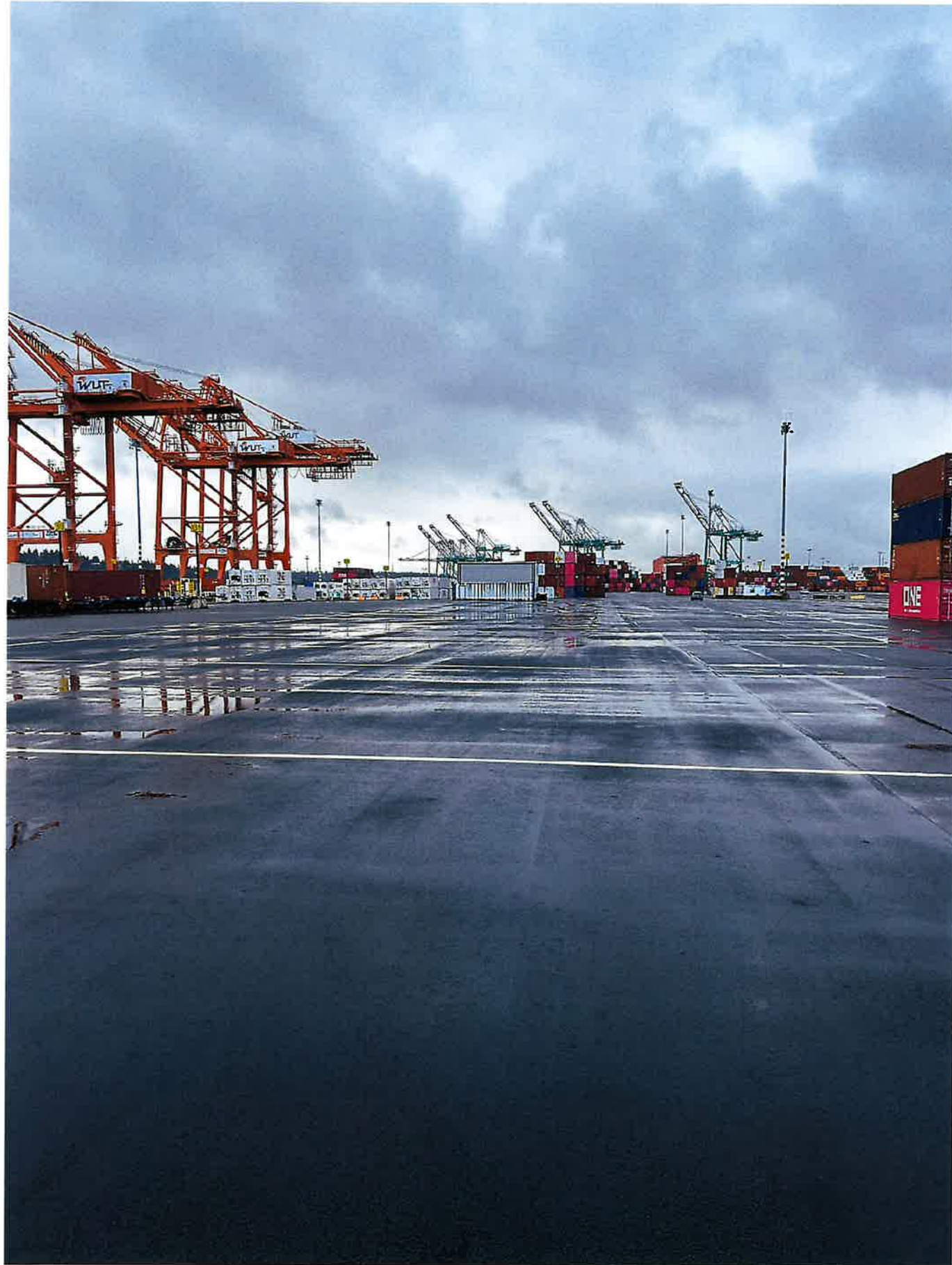
2024 repair area seen after paving. Work was completed on Thursday May 2 nd . Approximately 1000 tons of asphalt was removed and replaced. Surface water that is visible in areas is less than 1/8" deep. Pavement surface is solid and tight.
