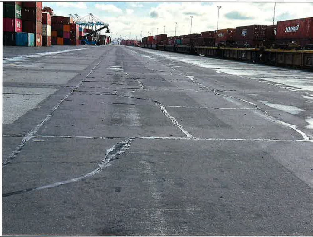
Typical joint and crack sealing. In 2010 the Port did an extensive repair of the concrete portion of the cap that included removal of all loose and spalled concrete. Rubberized mastic was placed back in the joints. In larger joints and pockets the mastic was extended with pea gravel to ensure better adhesion. The areas of work were then coated with an asphaltic slurry that included stone chips. This material is still present as seen in the area of black on the concrete. While surface cracking is occurring, the rubberized mastic installed previously is still in tack and providing protection from water intrusion. This effort provides a layer of surface protection for the previous repairs.
