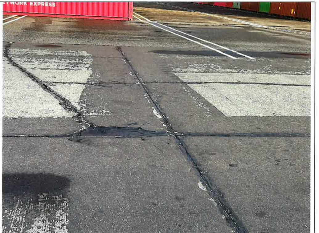
Area of larger spall filled with asphalt paving and adjacent cracks and joints sealed with AR 7000 Rubberized Mastic
