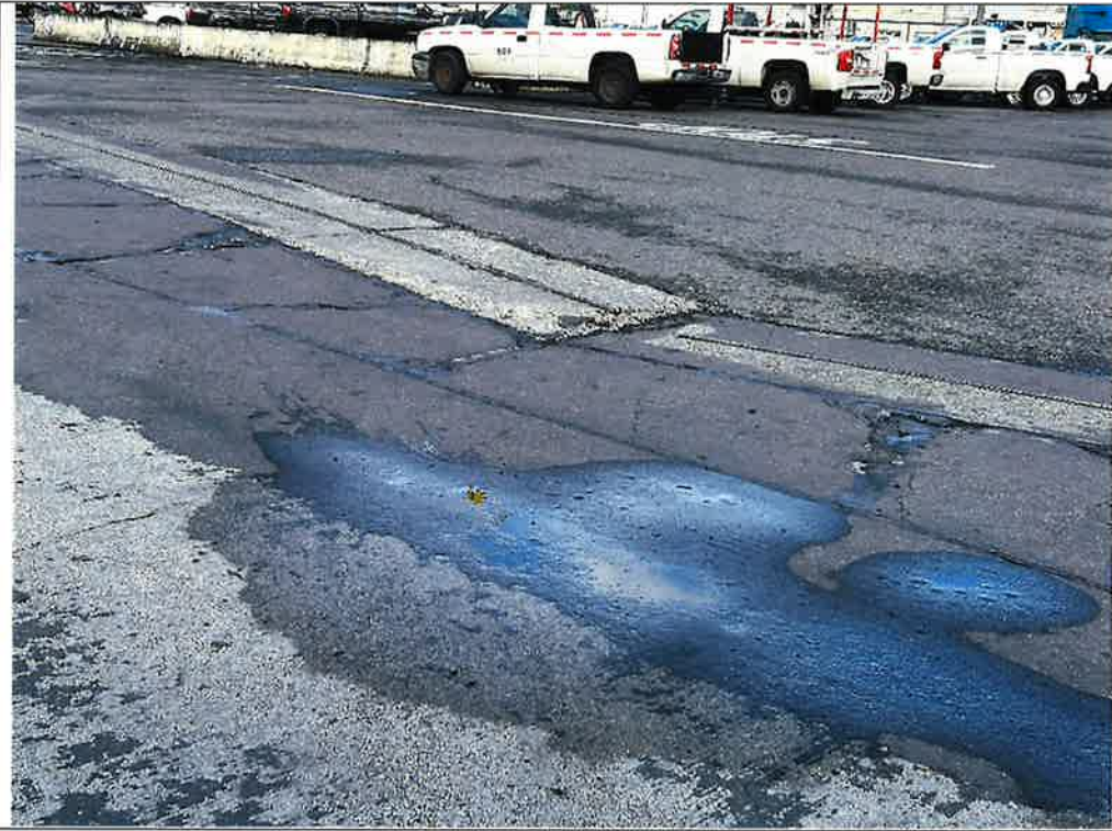
Cracks sealed at northeast end of work area around strip drain
