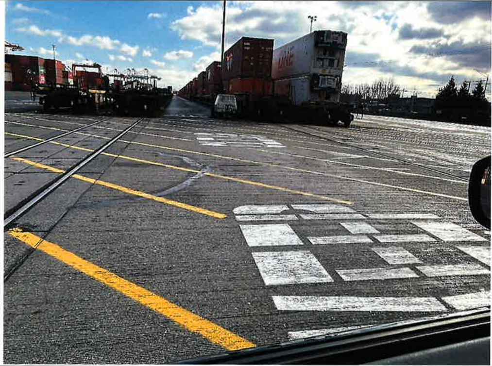
Within the crossing the tubs on the rail lines are not included in this maintenance effort. Only the crossing panel cracks are sealed.
