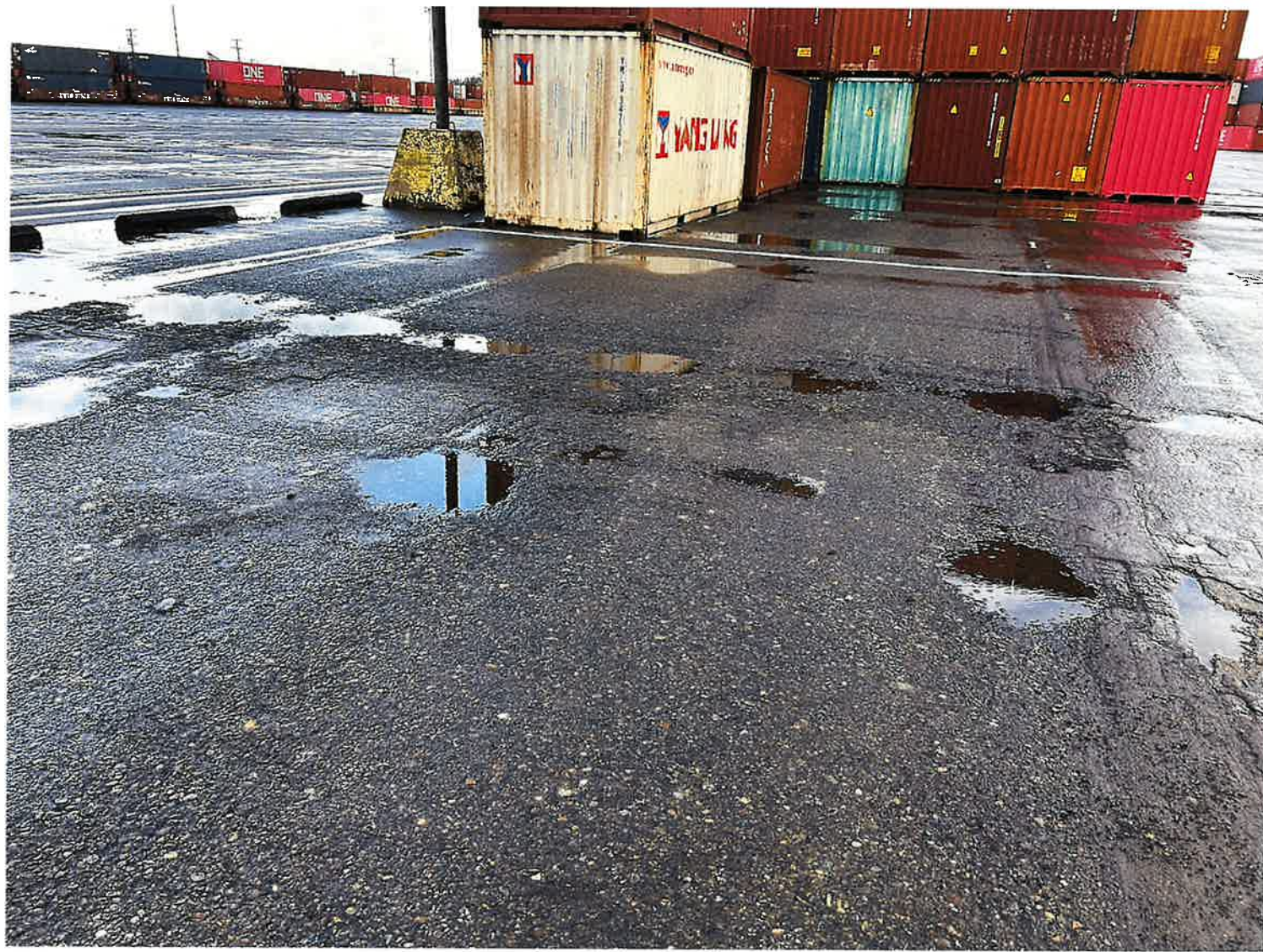
Adjacent area to repair seen after a recent rain. Damage from container pockets creates a field of puddles.
