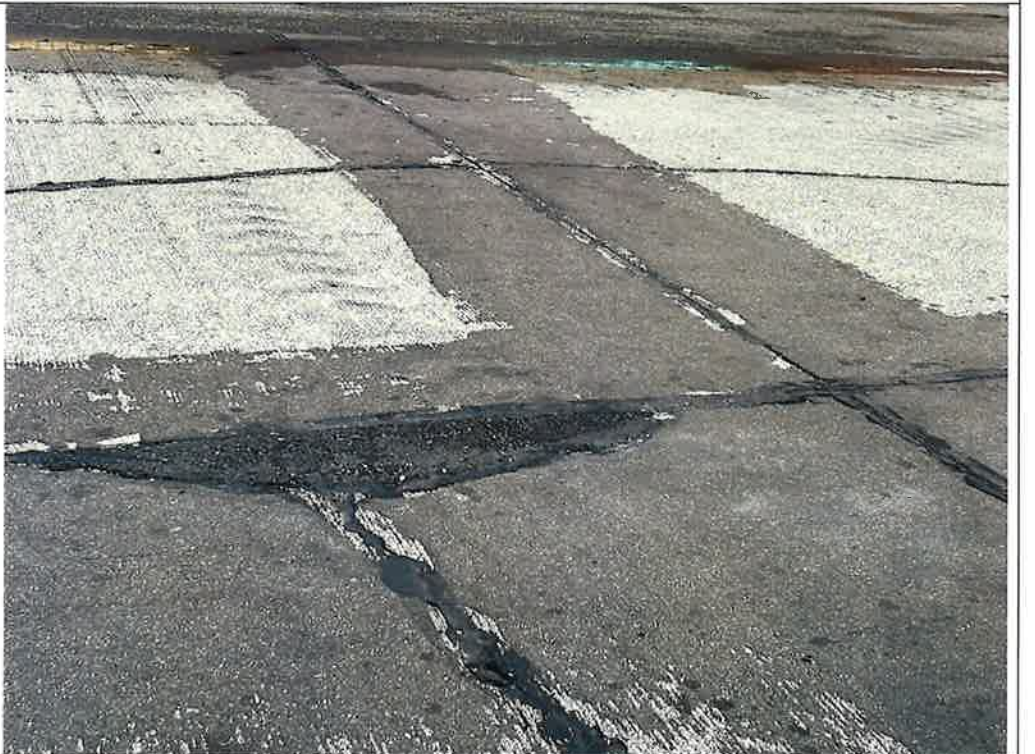
Area of larger spall repaired with asphalt
