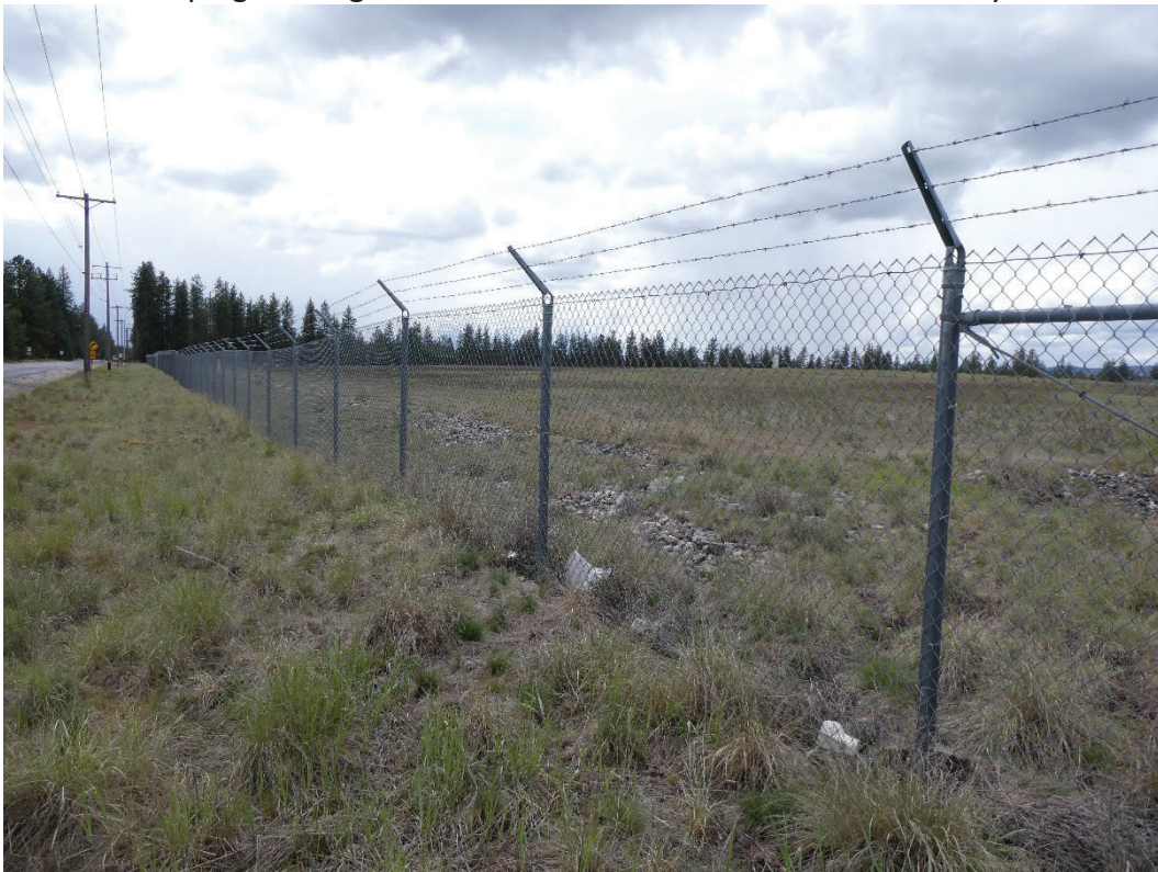
Fencing along landfill
