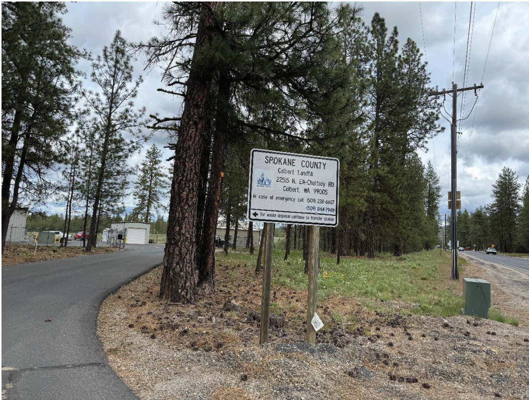
Signage at entrance of groundwater extraction and treatment facility
