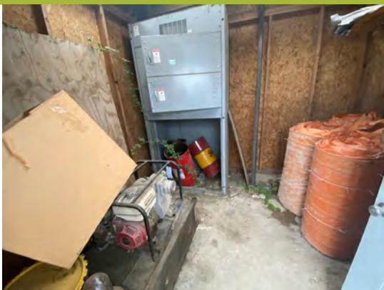
Photograph #23: Shed interior.
