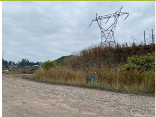
Photograph #10: Monitoring well located on northeast portion of site.
