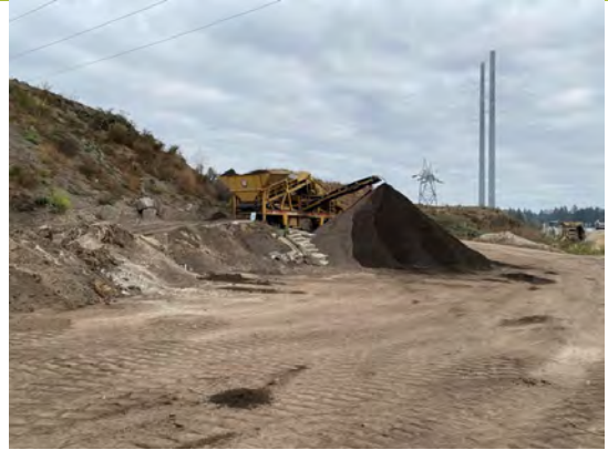
Photograph #32: On-site operations.
