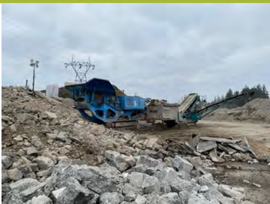
Photograph #11: On-site hydraulic machinery.
