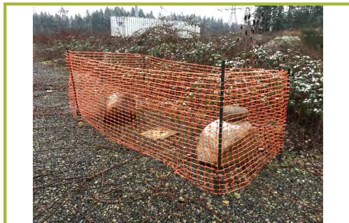
Photograph #2: View of MW-3 located near the stormwater retention pond. Looking south west.
