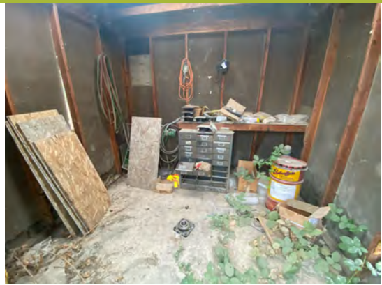
Photograph #22: Shed interior.
