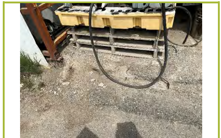
Photograph #24: Condition of soil surrounding AST (no staining) and diesel exhaust fluid.
