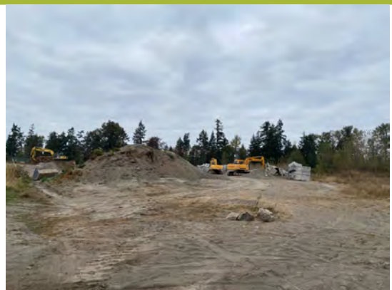
Photograph #6: On-site operations.
