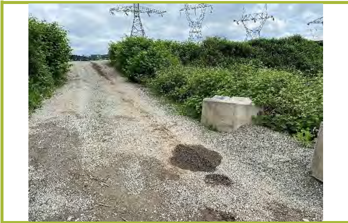
Photograph #15: De minimis staining north of stormwater detention pond.
