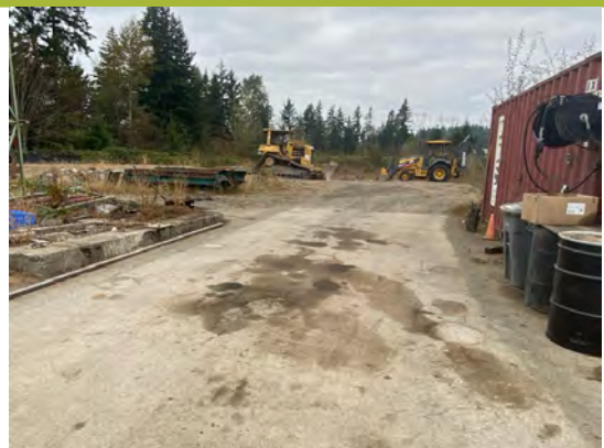
Photograph #18: Deminimus staining adjacent to storage container.
