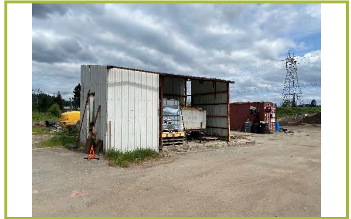
Photograph #22: Shed located on northwest corner of Subject Property (stores diesel exhaust fluid AST).
