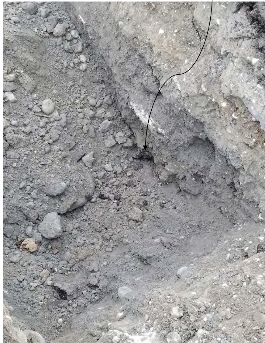
Trench 2 (note visible pieces of asphalt)
