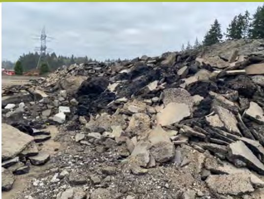
Photograph #29: Crushed asphalt.
