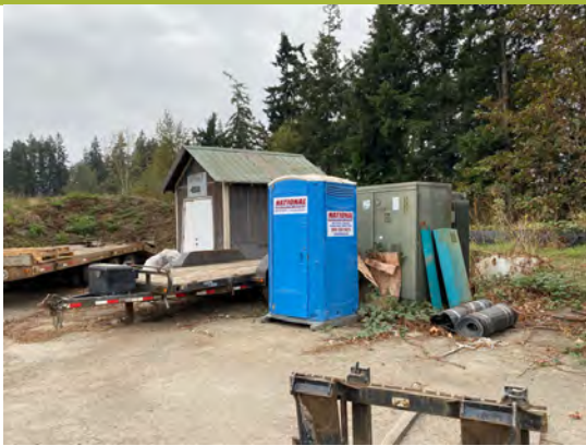
Photograph #21: Storage sheds on northwest portion of site.
