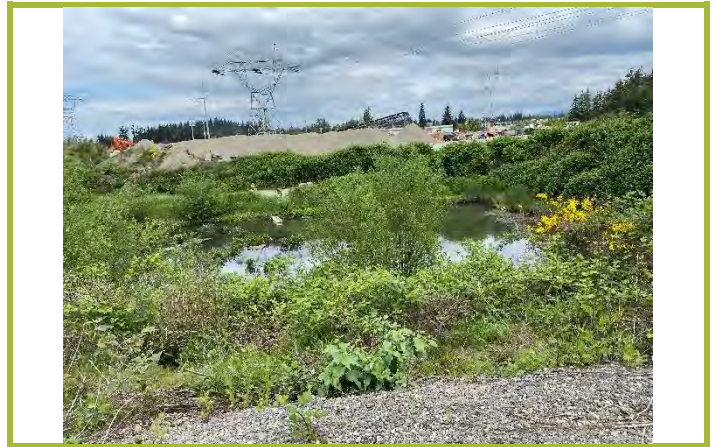
Photograph #16: View of detention pond; no sheen observed.
