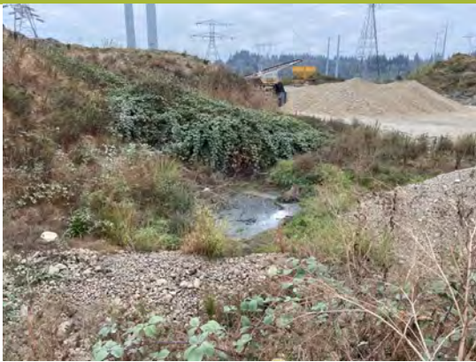
Photograph #33: Water pooling after hard rain.
