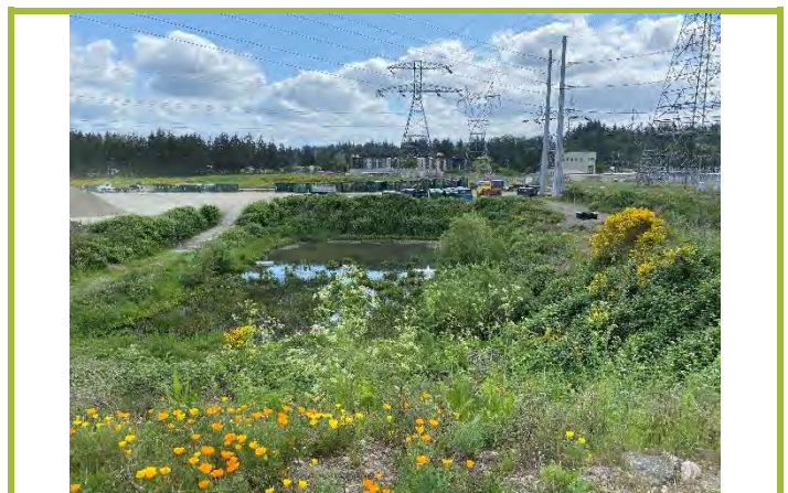
Photograph #6: Stormwater detention pond on southeast portion of Subject Property.
