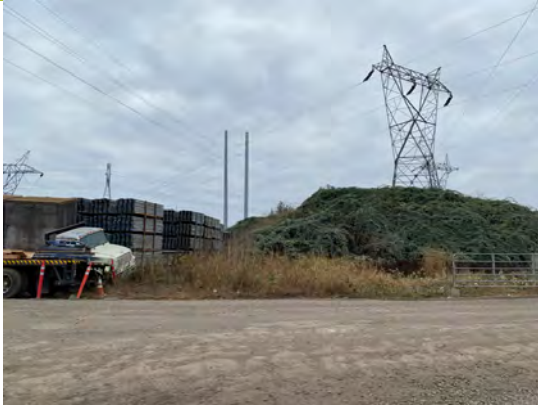
Photograph #1: Northeast corner of site.
