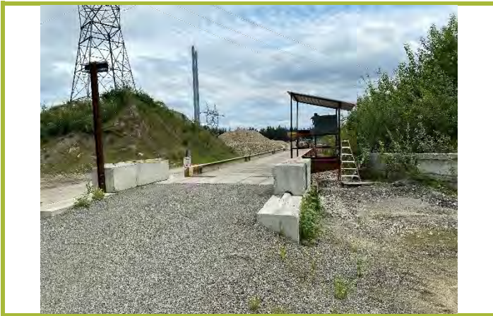
Photograph #19: Weigh station located on southeast portion of Subject Property.
