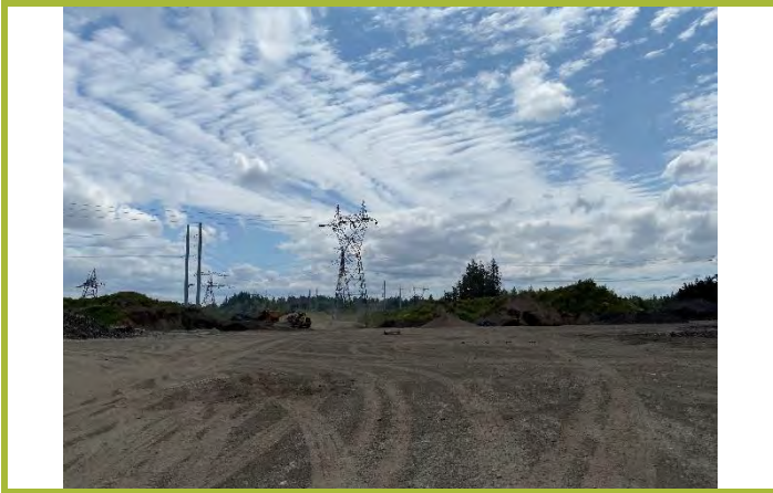
Photograph #1: General condition of the Subject Property.
